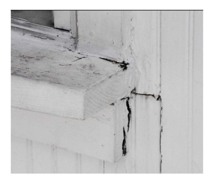
WARPING AND ROTTING BEADED BOARD SIDING
