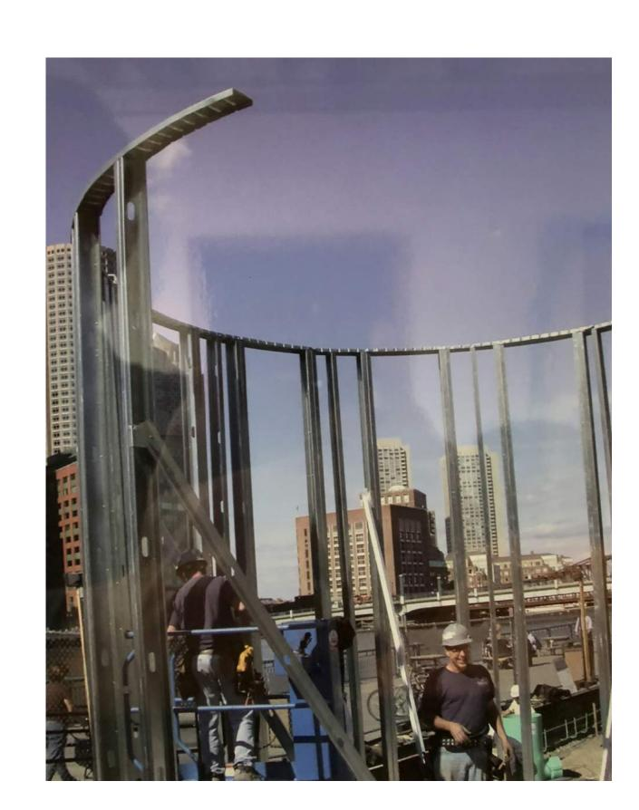
6 MILK BOTTLE BOTTOM REBUILT IN METAL STUD FRAMING
