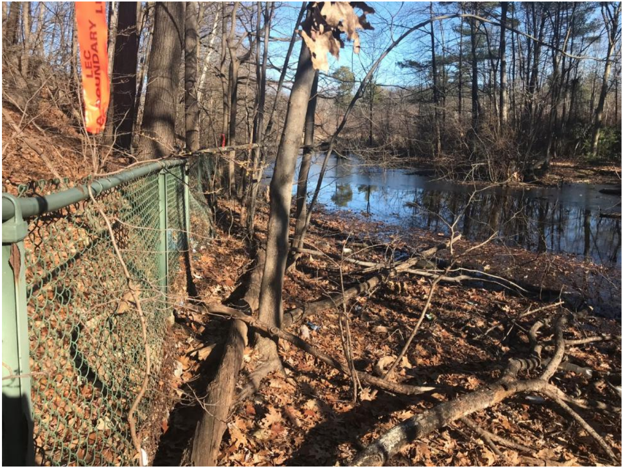
View of southern extent of fence to be removed. Fence is located at or slightly within wetland.
