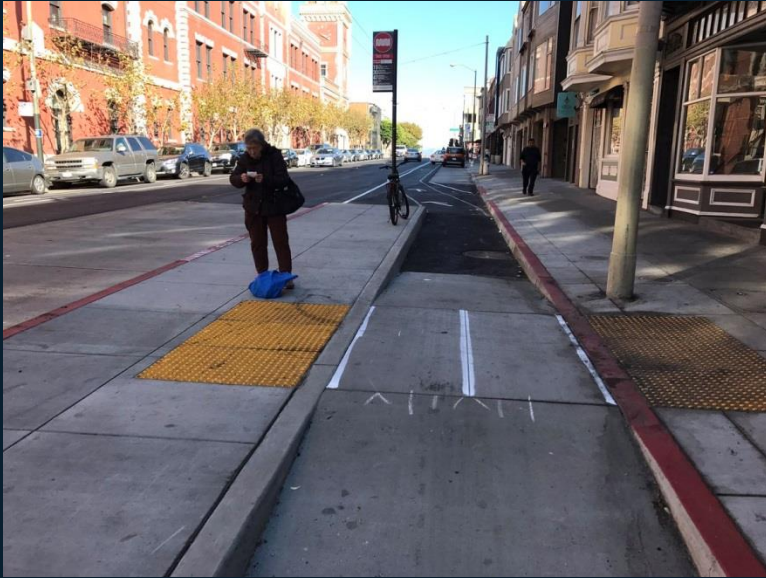
San Francisco (under construction)
