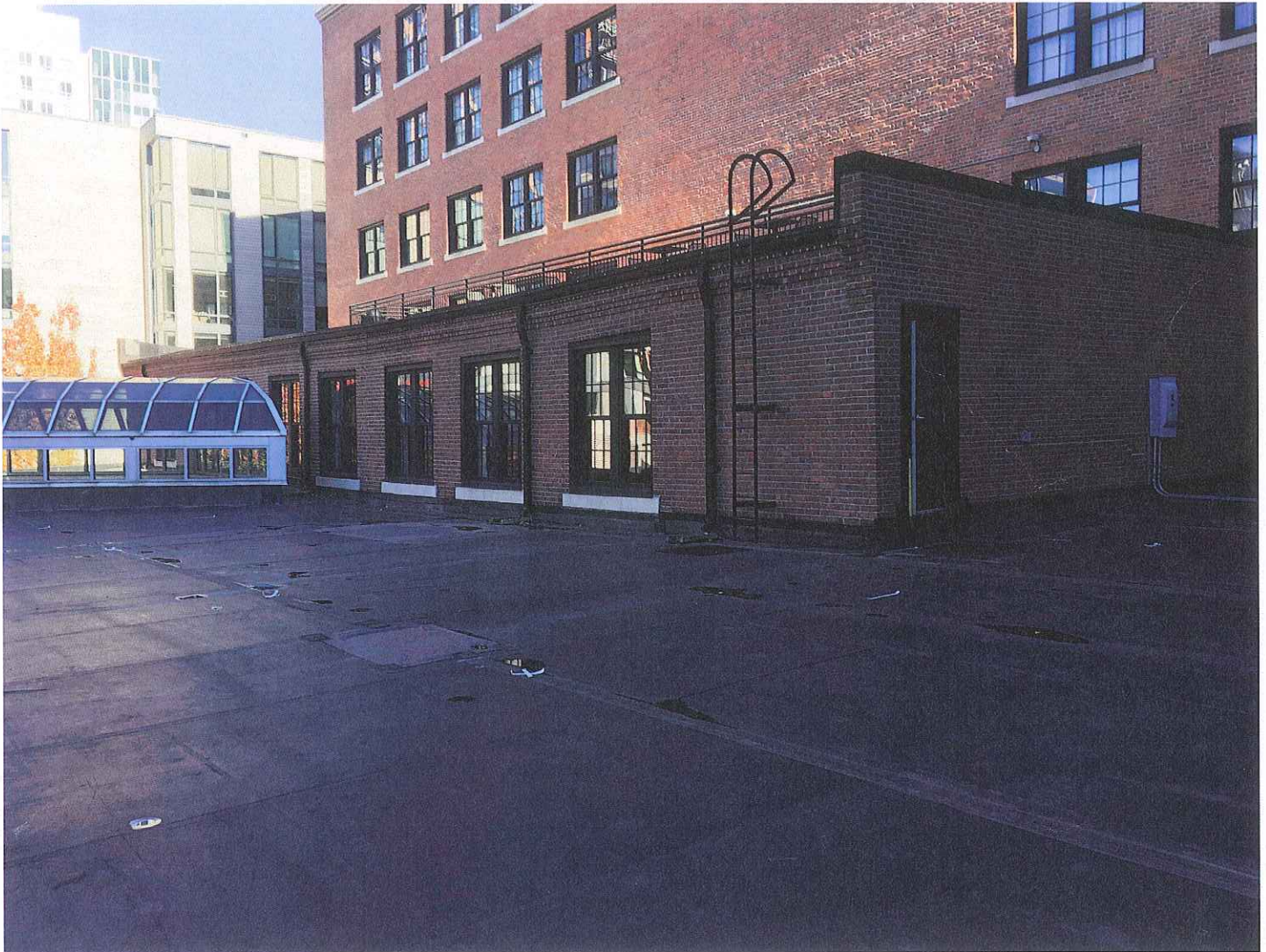
Existing Roof Conditions 11.07.2018
