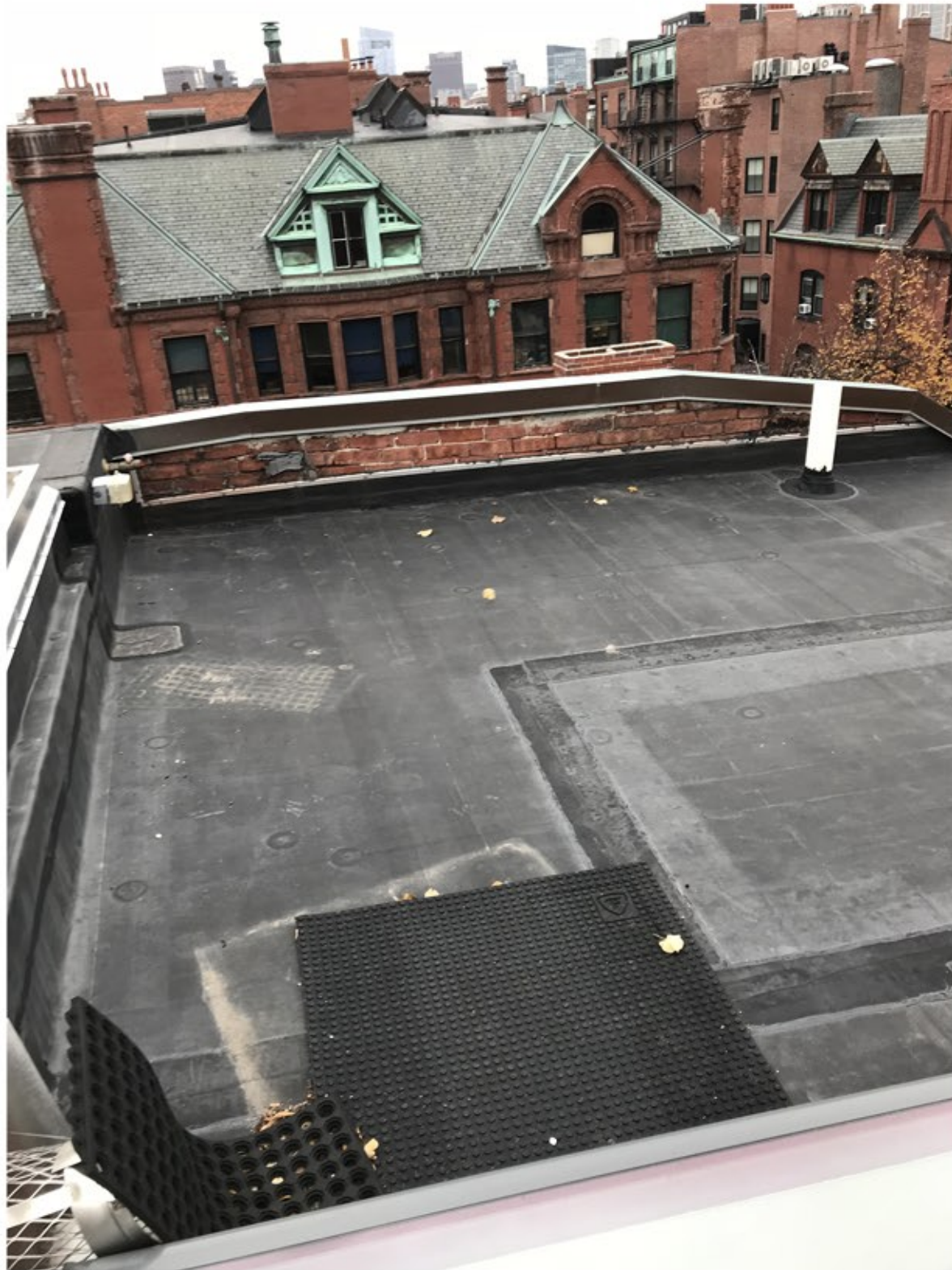
EXISTING REAR ROOF
