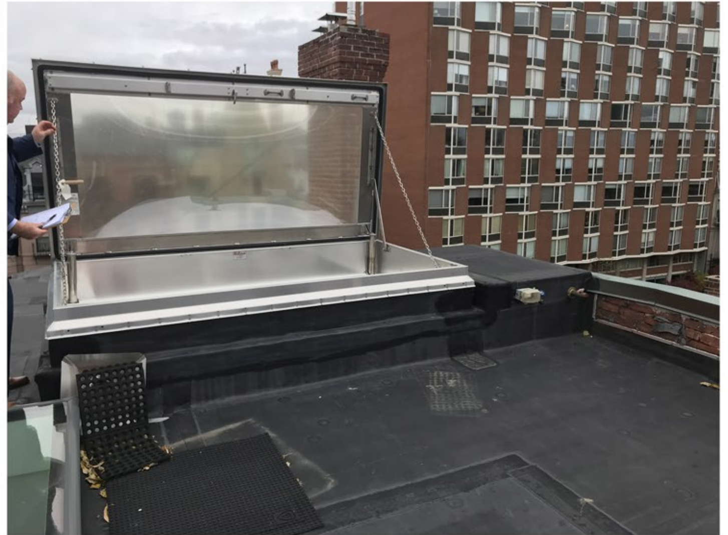
EXISTING ROOF HATCH
