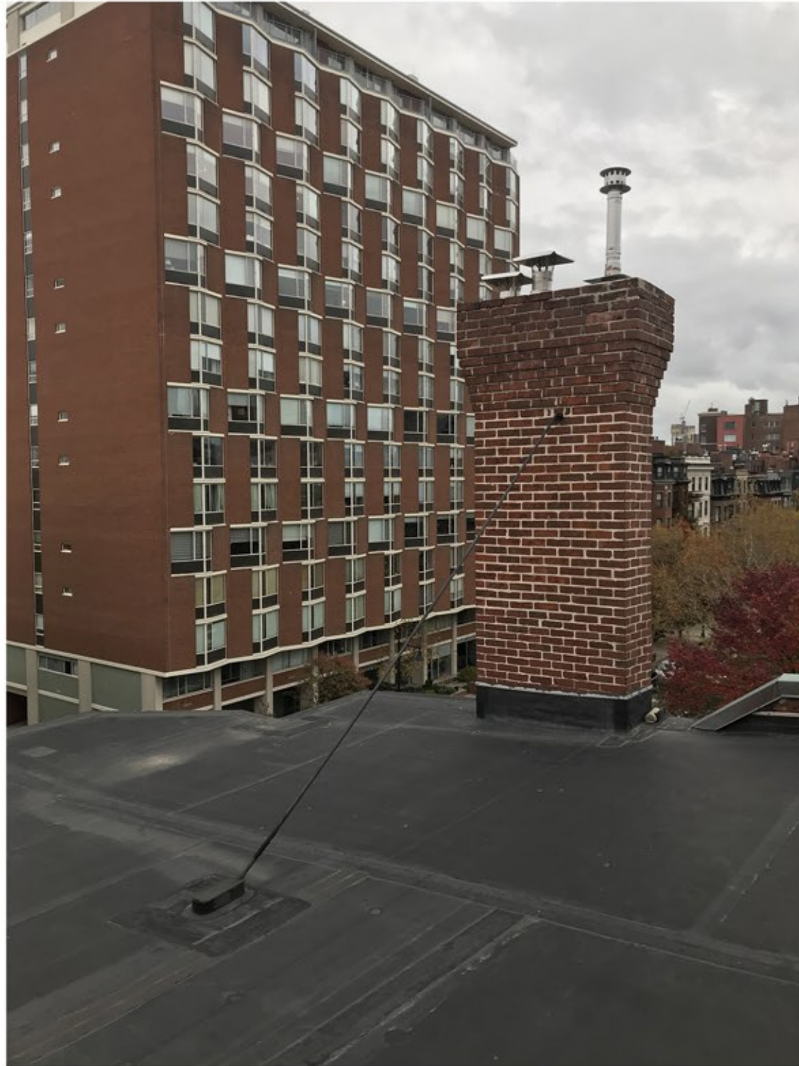
EXISTING FRONT ROOF
