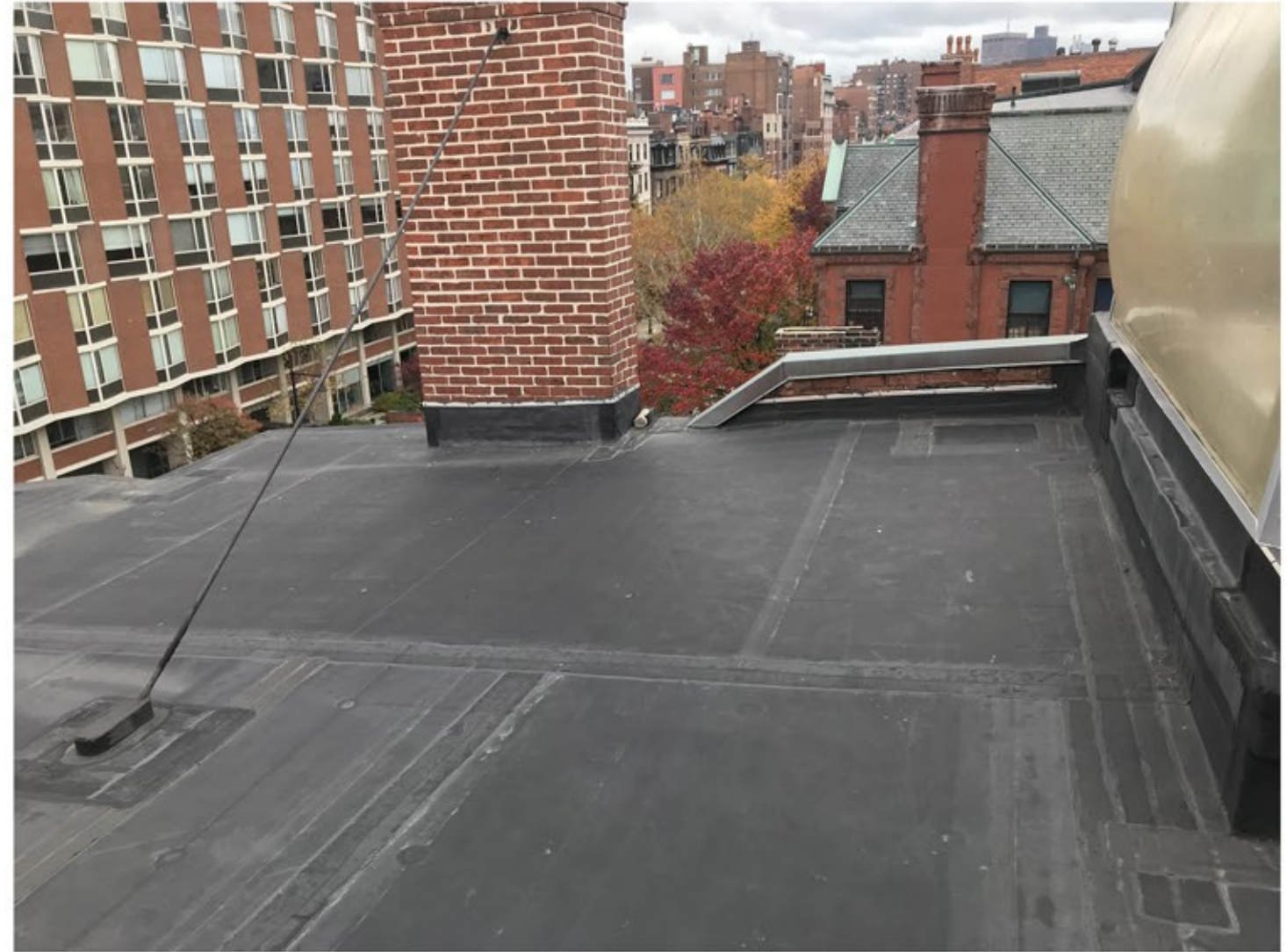
EXISTING FRONT ROOF
