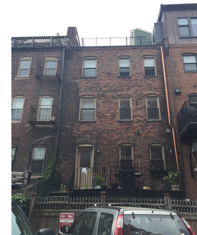
4 EXISTING CONDITIONS @ REAR 1/4" = 1'-0"
