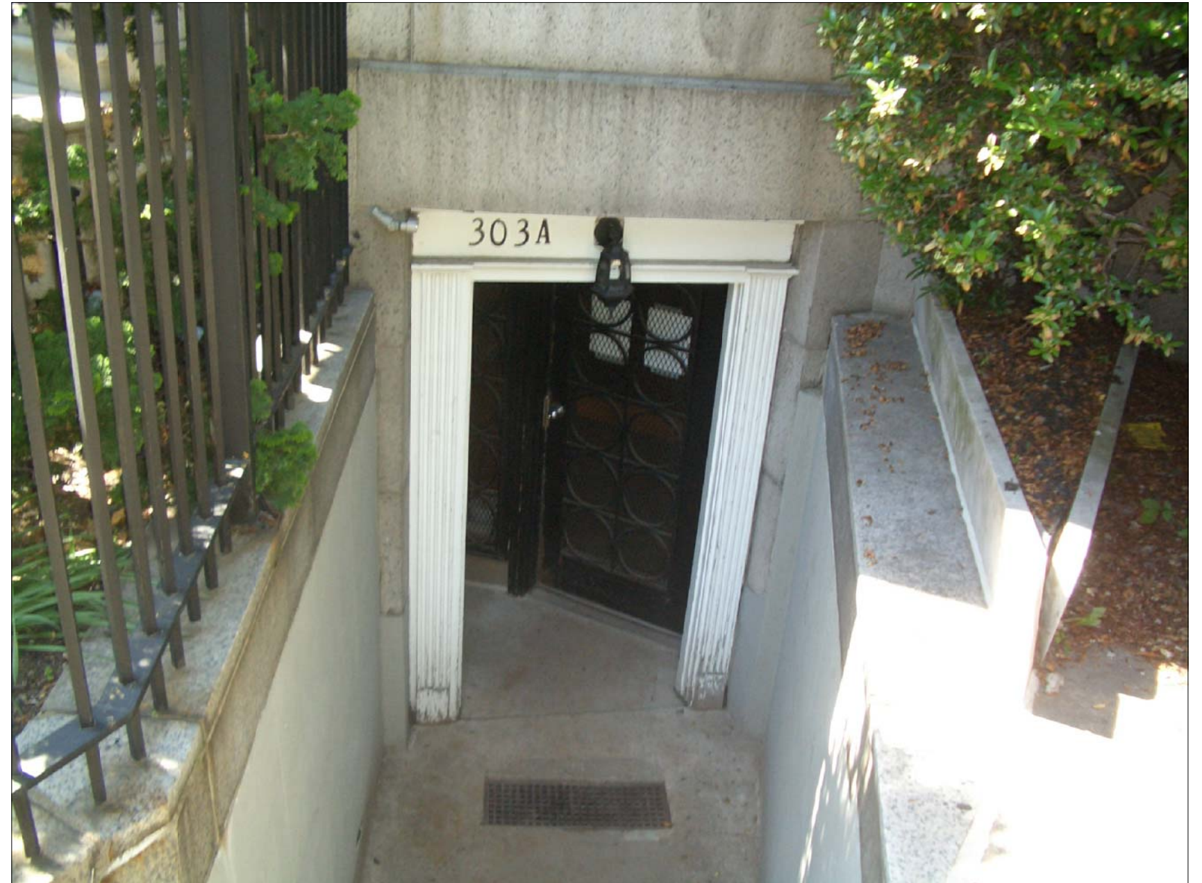
BASEMENT DOOR 303 Commonwealth Avenue
