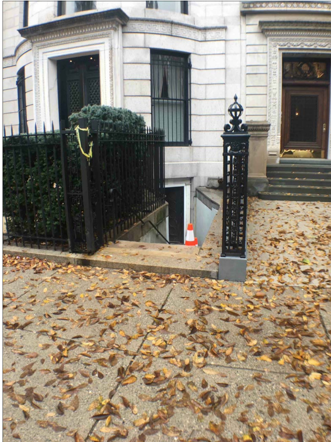
AREA WAY ENTRANCE 303 Commonwealth Avenue
