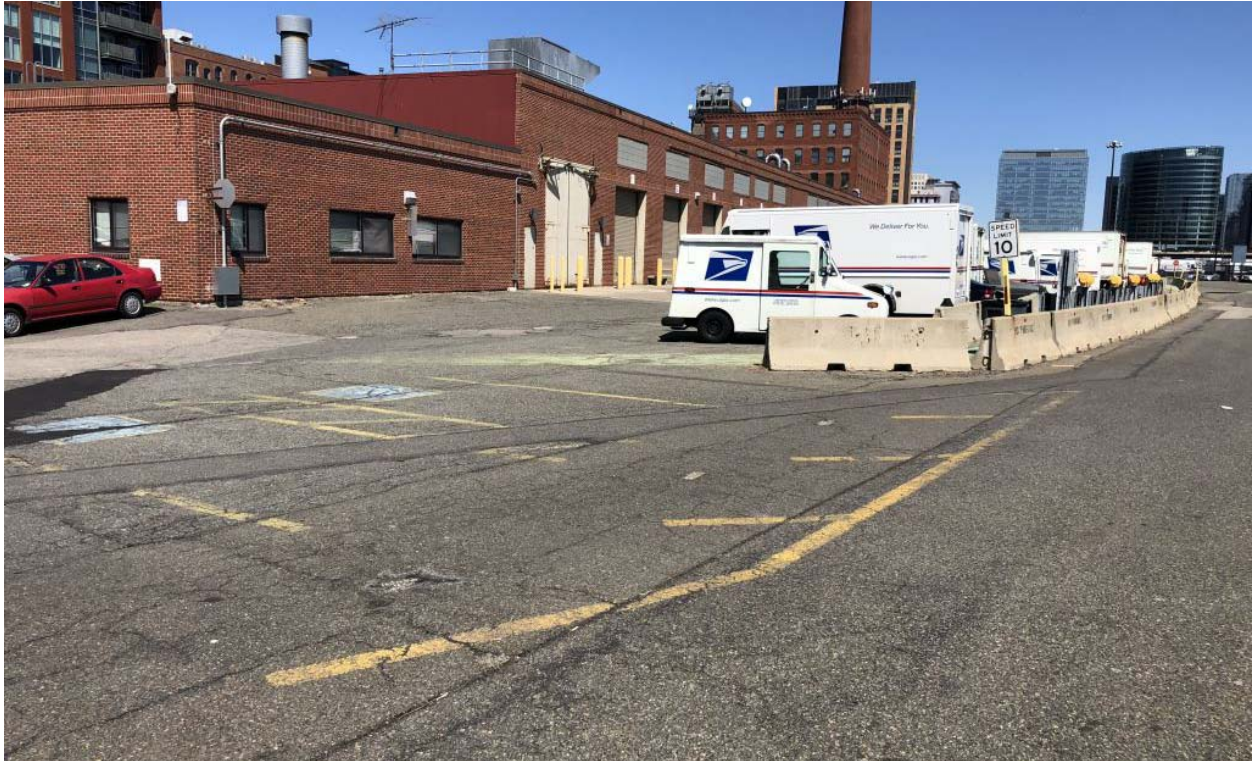
Photo 3 – Parking and maintenance bay doors along southeasterly side of VMF building looking northeast, with access laneway at right (GRA photo)
