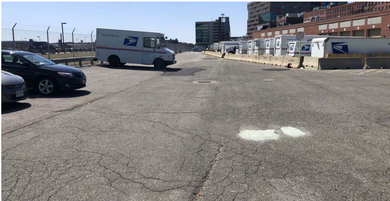
Photo 4 – Access laneway along southeasterly side of VMF looking southwest (GRA photo)
