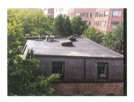
Existing Condensers on roof will be replaced with Fujitsu 24K condensers which have a lower height profile, and are smaller overall (shown below):  $27\,9/16$ " H x 13" D x 35" W
