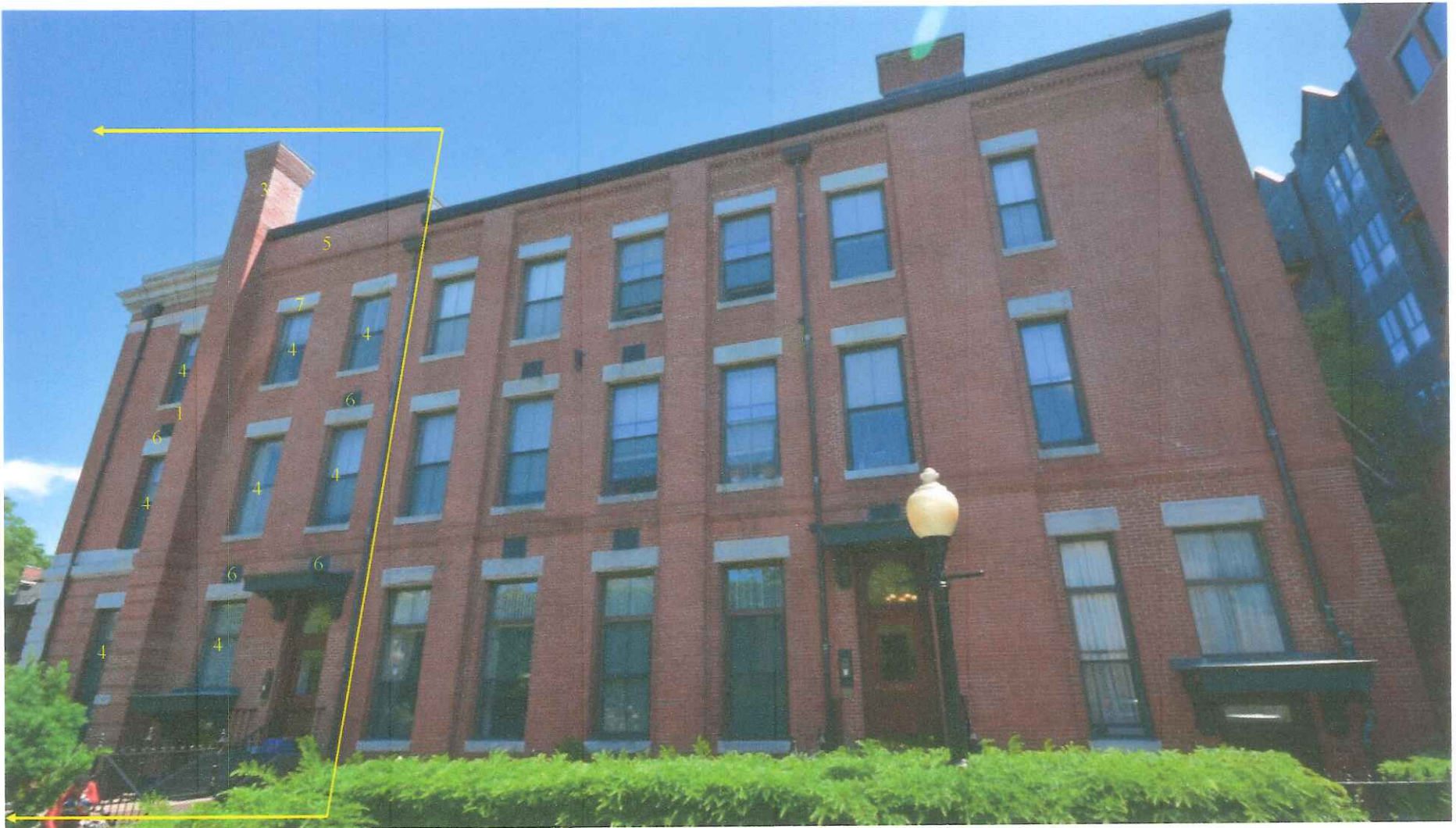
70-80 Warren Avenue – Right Side, West Facing Elevation
