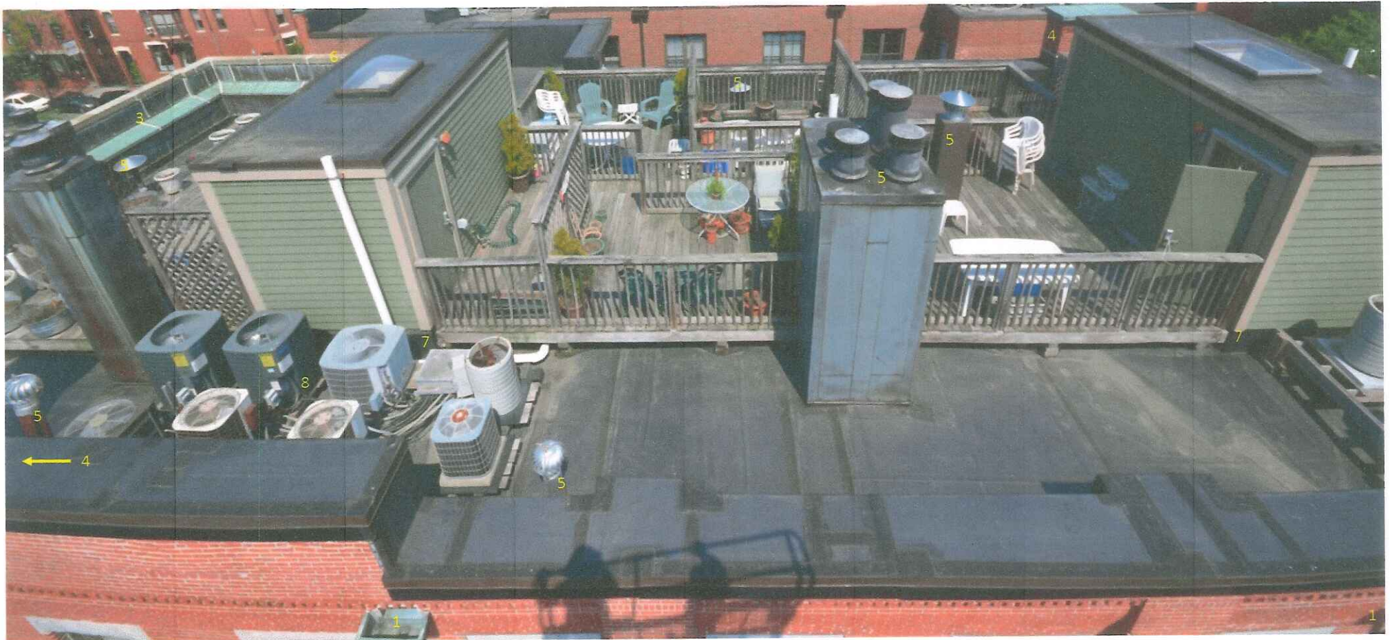
70-80 Warren Avenue Roof
