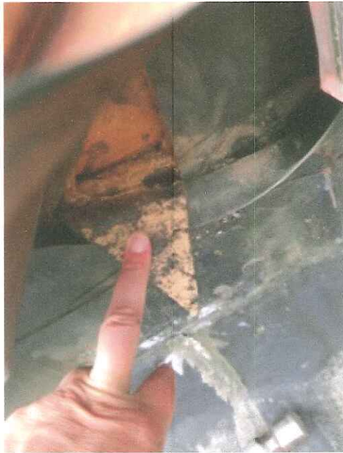
Parapet has many layers of roofing products on it including two layers of EPDM, asphalt, fiberboard over plywood.
