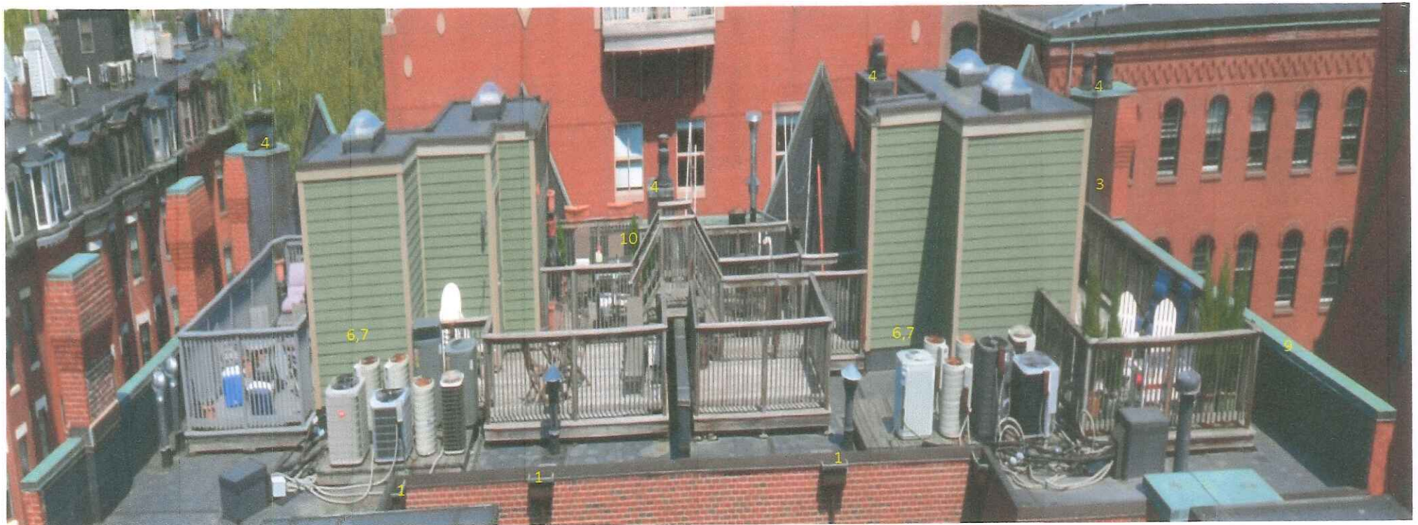
4- 18 Clarendon Street Roof
