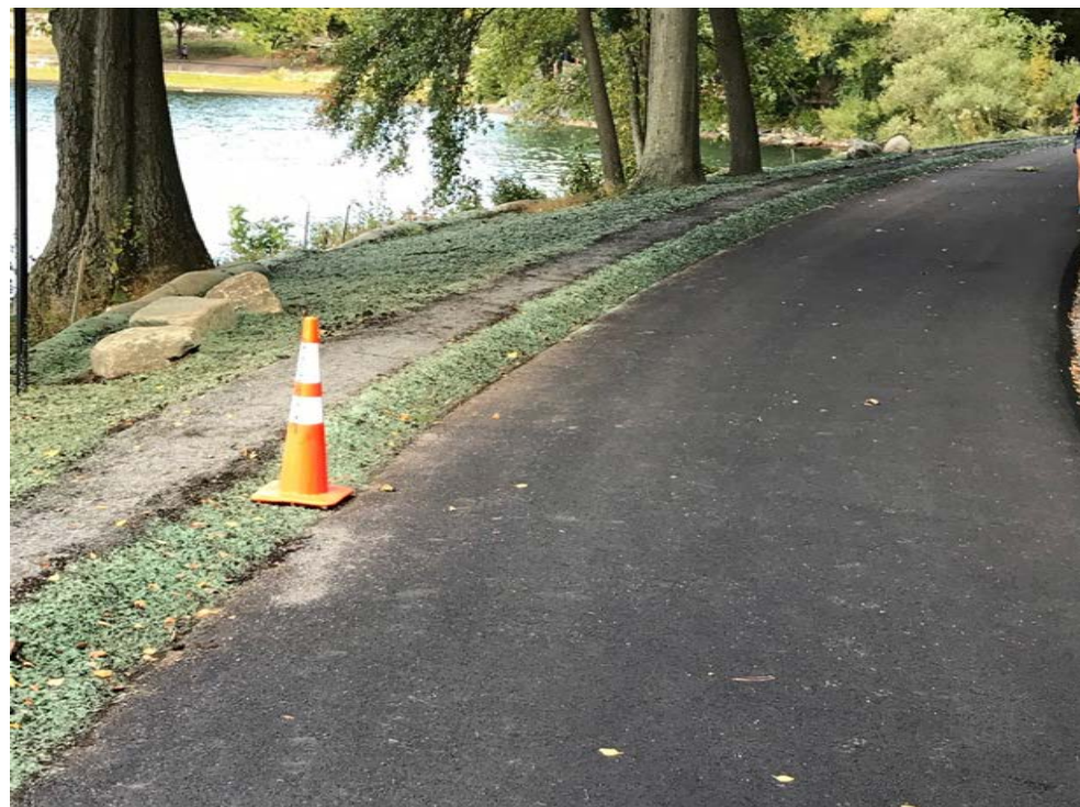
Location of proposed cobblestone spillway; Sediment shows evidence of puddling.
