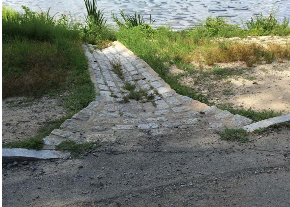
Example of an existing cobblestone spillway, prior to retrofit.
