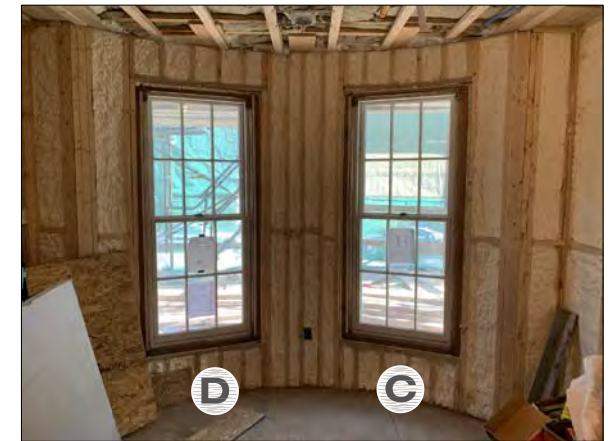
10 Exhibit - Existing non-original windows; interior view at First Floor
