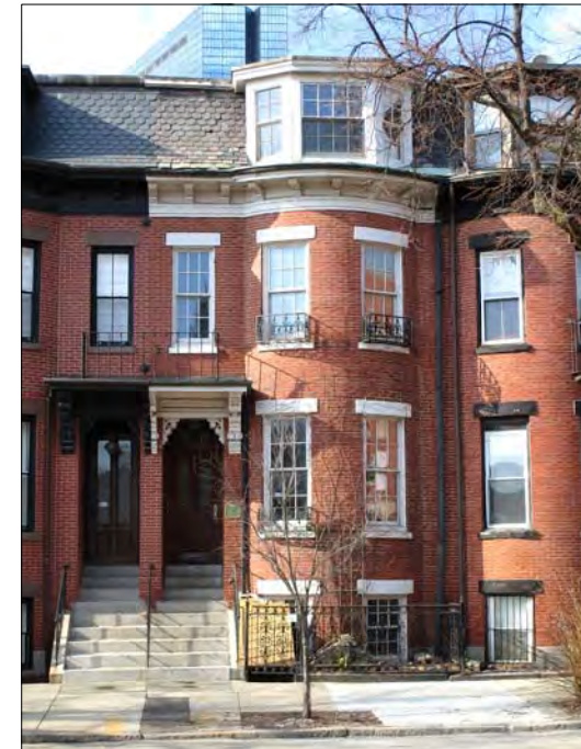
11 Exhibit - Existing facade of subject property, 77 Warren Ave.
