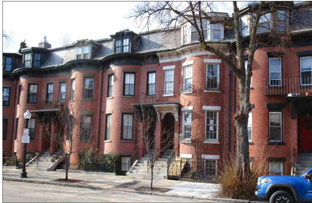
15 Exhibit - Existing facade of subject property, 77 Warren Ave. with adjacent neighbors.
