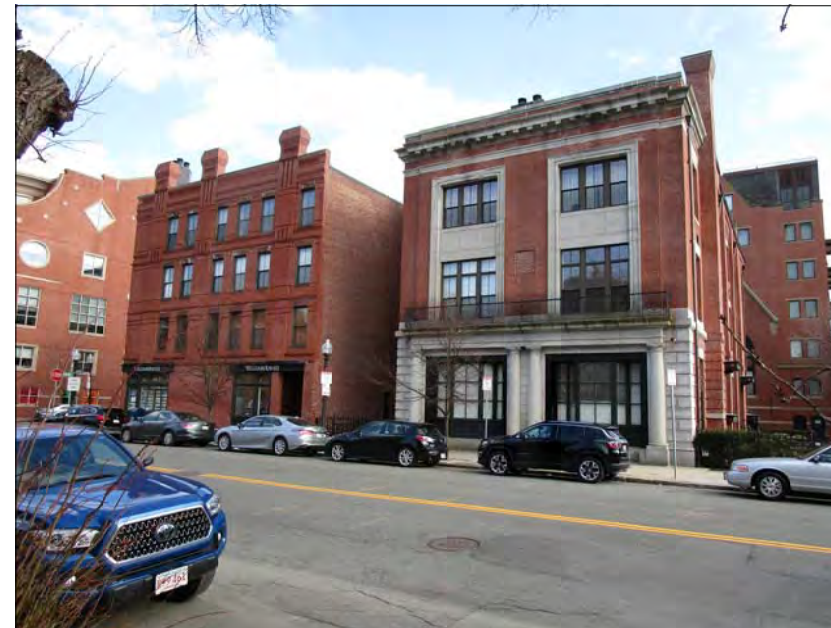
18 Exhibit - Streetscape; Warren Ave. - view looking across street from subject property
