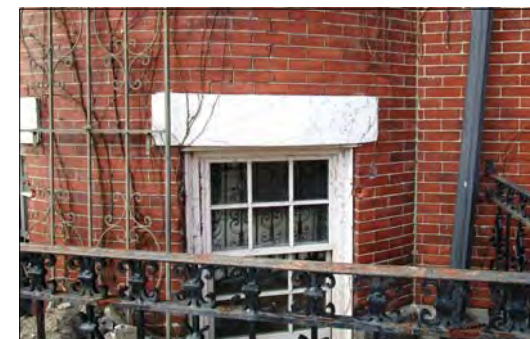
13 Exhibit - Existing masonry lintel of subject property, 77 Warren Ave.
