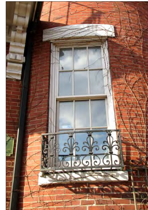
5 Exhibit - Existing non-original window frame and sash of subject property, 77 Warren Ave.
