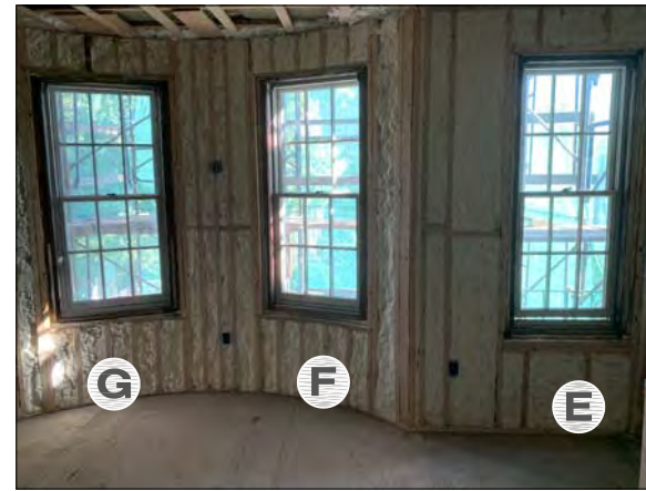
7 Exhibit - Existing non-original windows; interior view at Third Floor
