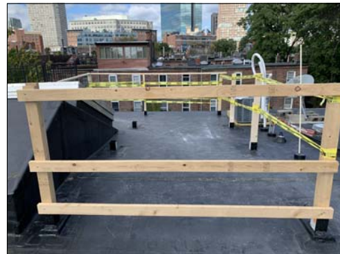
27 Exhibit - Mock-up roof deck railing - North view
