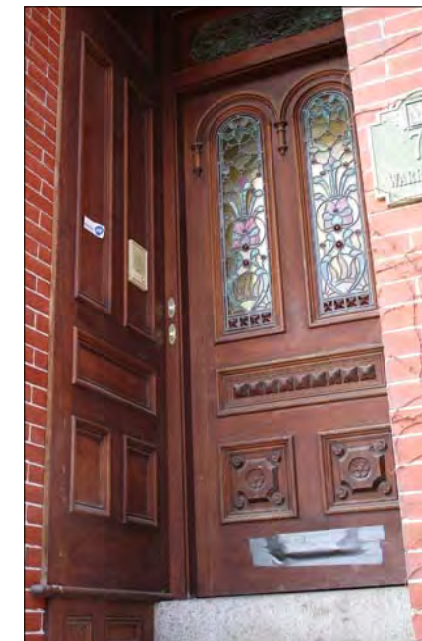
4 Exhibit - Existing non-original entry door and surround of subject property, 77 Warren Ave.
