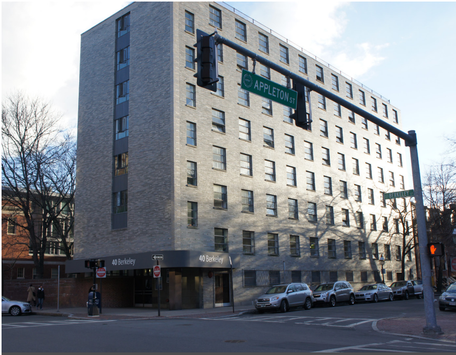
A - Appleton Street Facade
