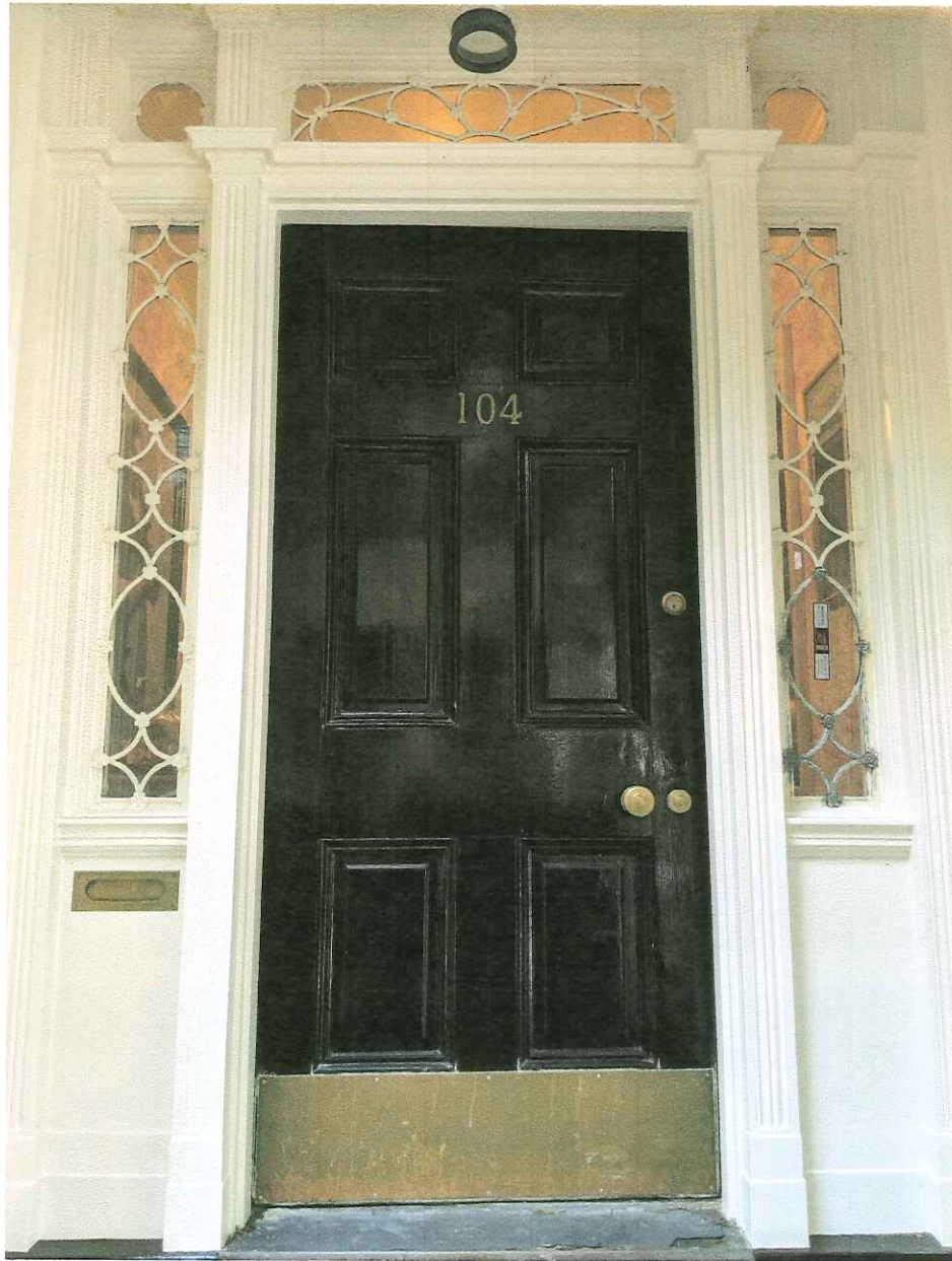
104 door existing condition
