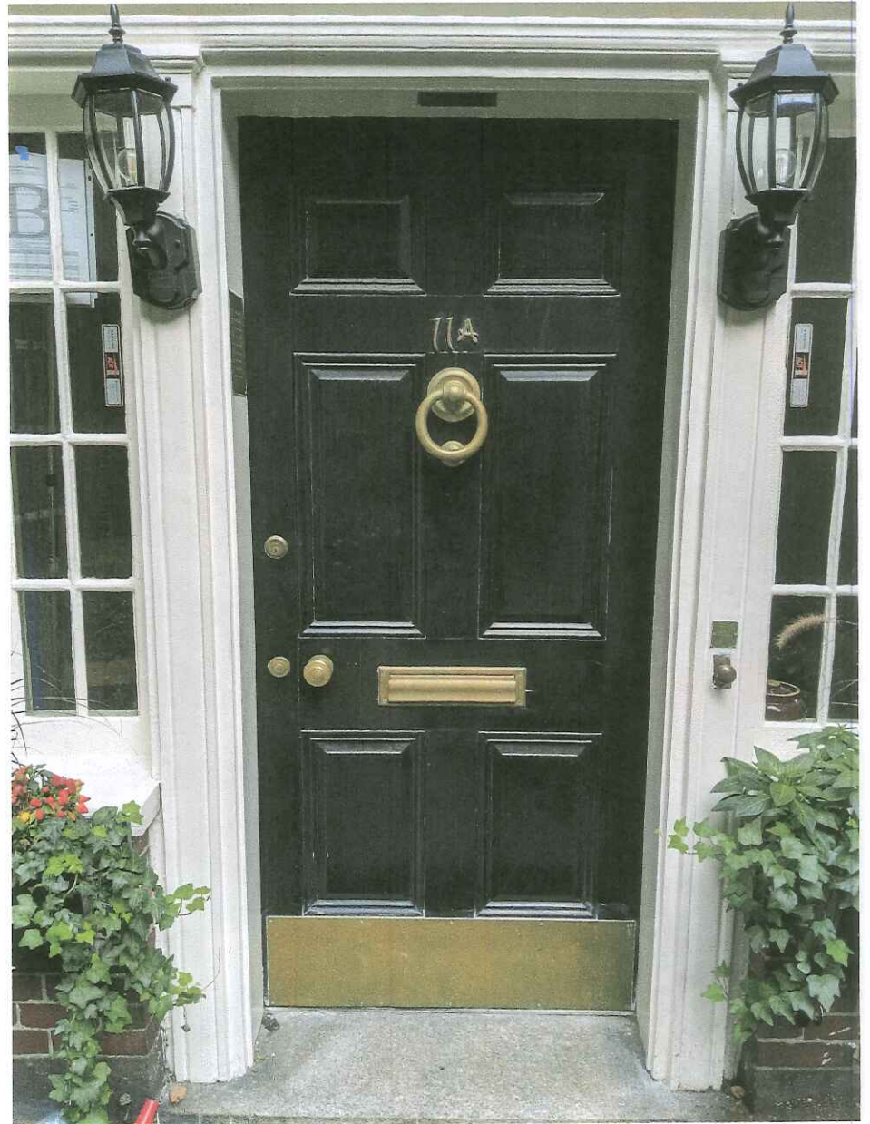
11A Door existing condition
