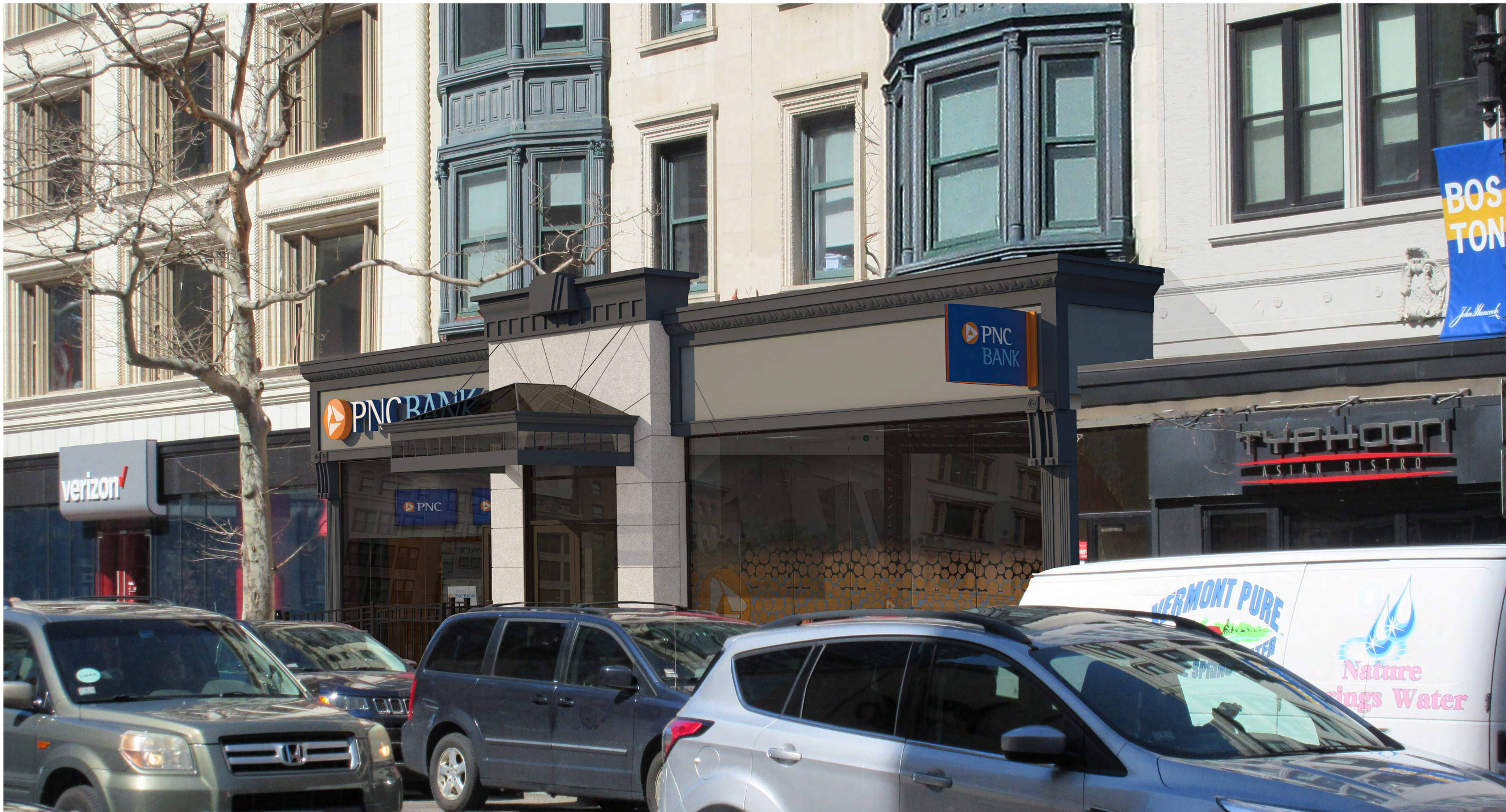
VIEW #2 LOOKING WEST ON BOYLSTON ST
