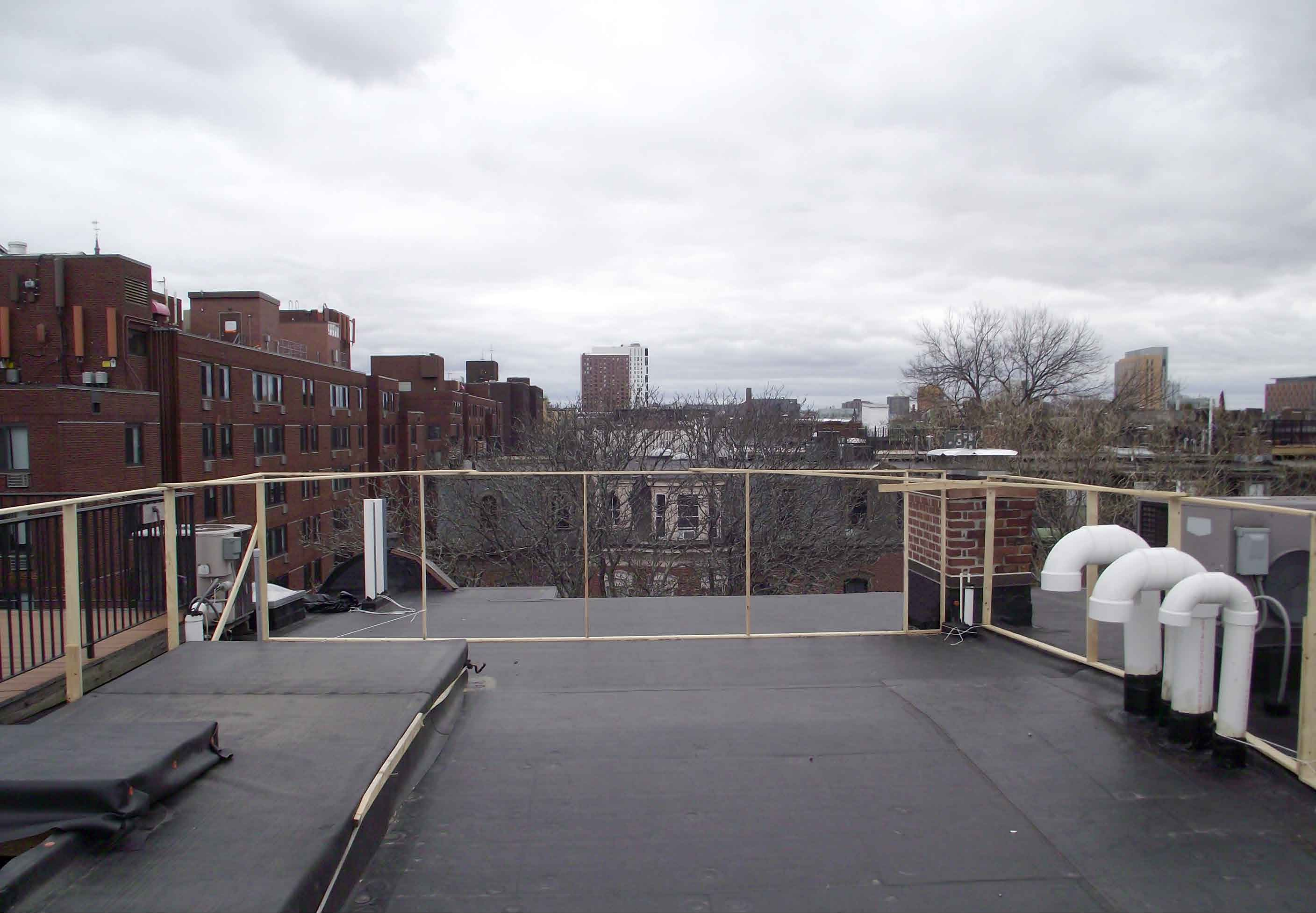
Rooftop Proposed Conditions: View Facing Front of Building / Rutland Sq
