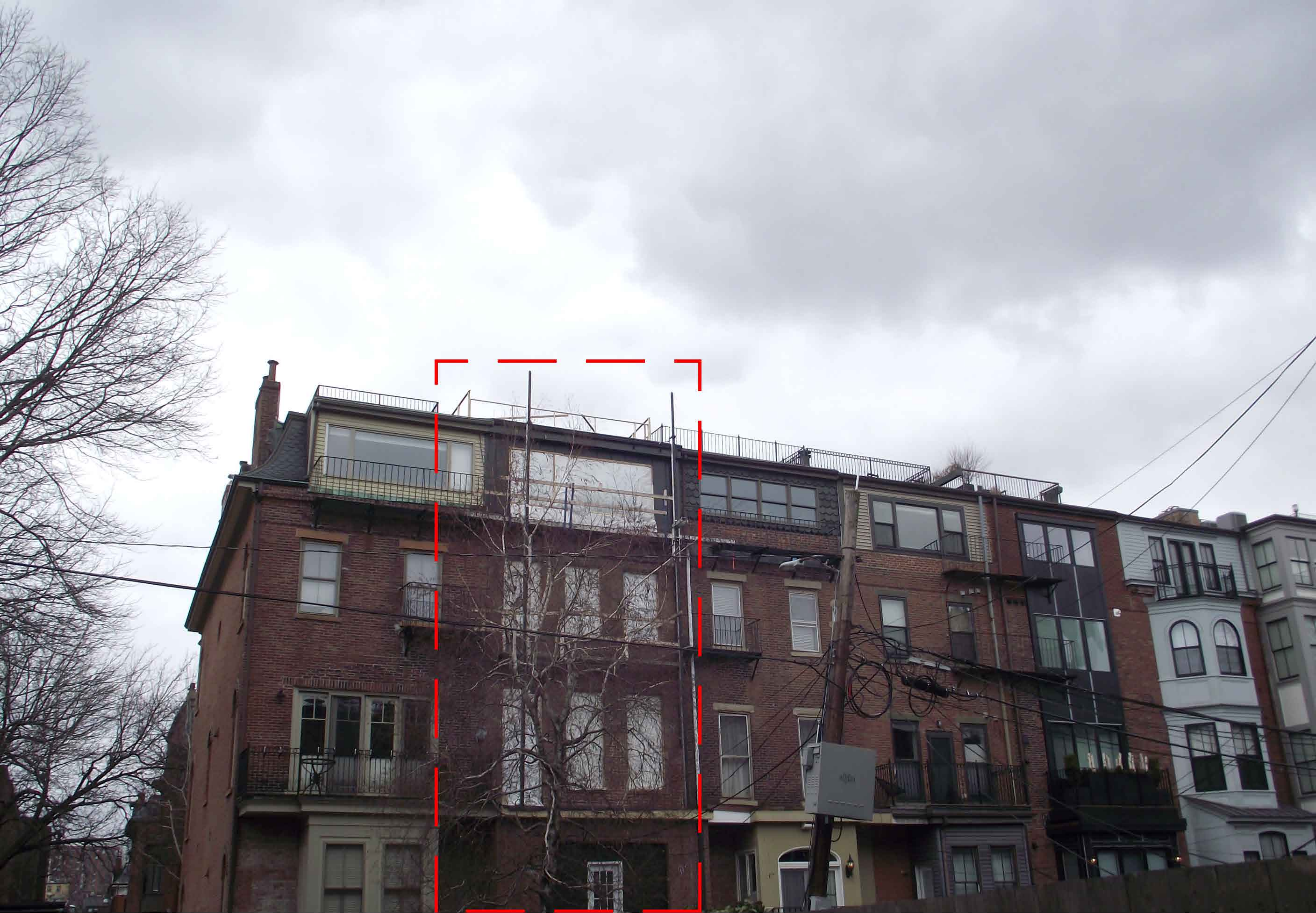
Rooftop Proposed Conditions: View of Rear of 5 Rutland Sq from Private Alley
