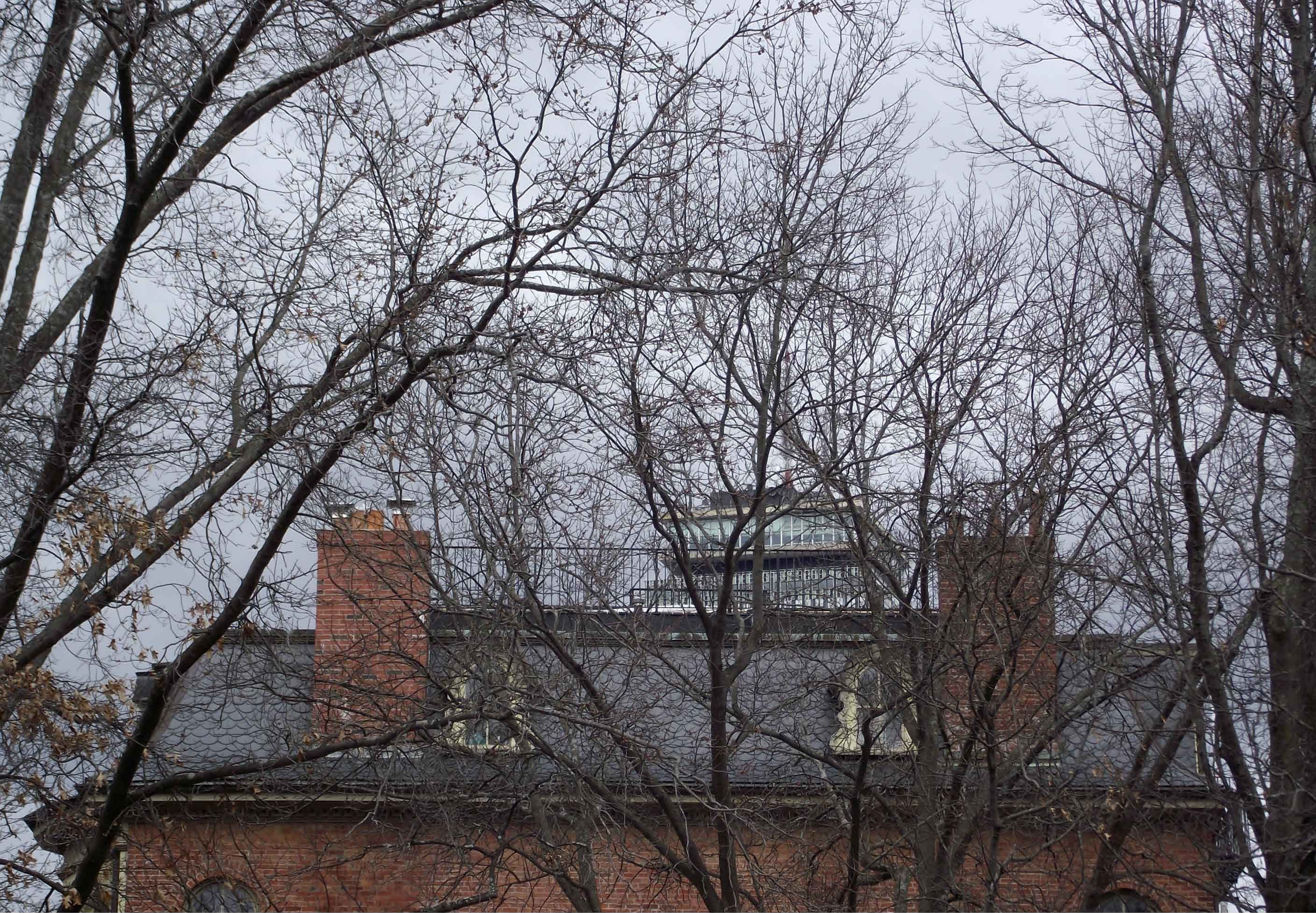
Rooftop Proposed Conditions: View from Tremont Street
