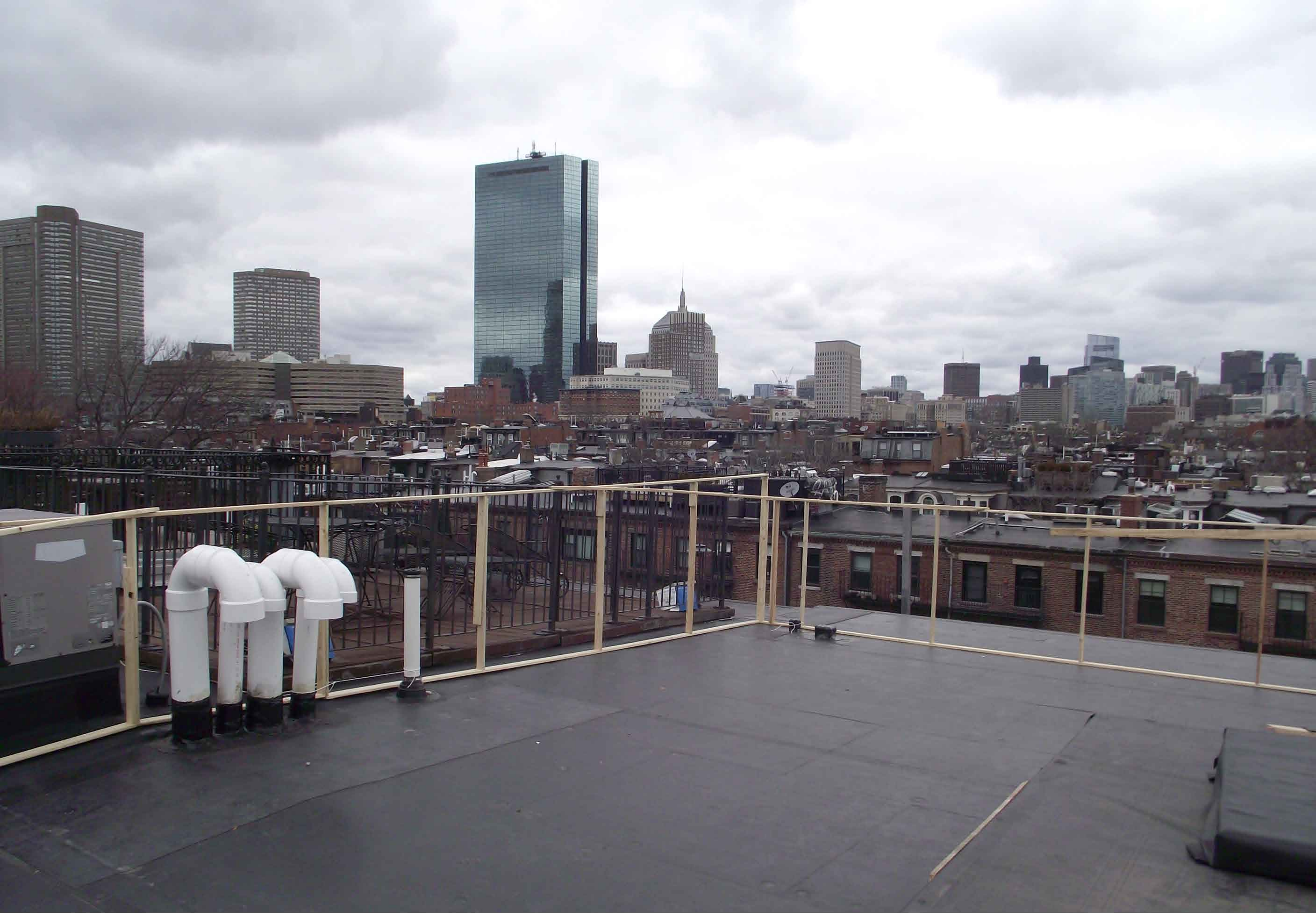
Rooftop Proposed Conditions: View Facing 7 Rutland Sq
