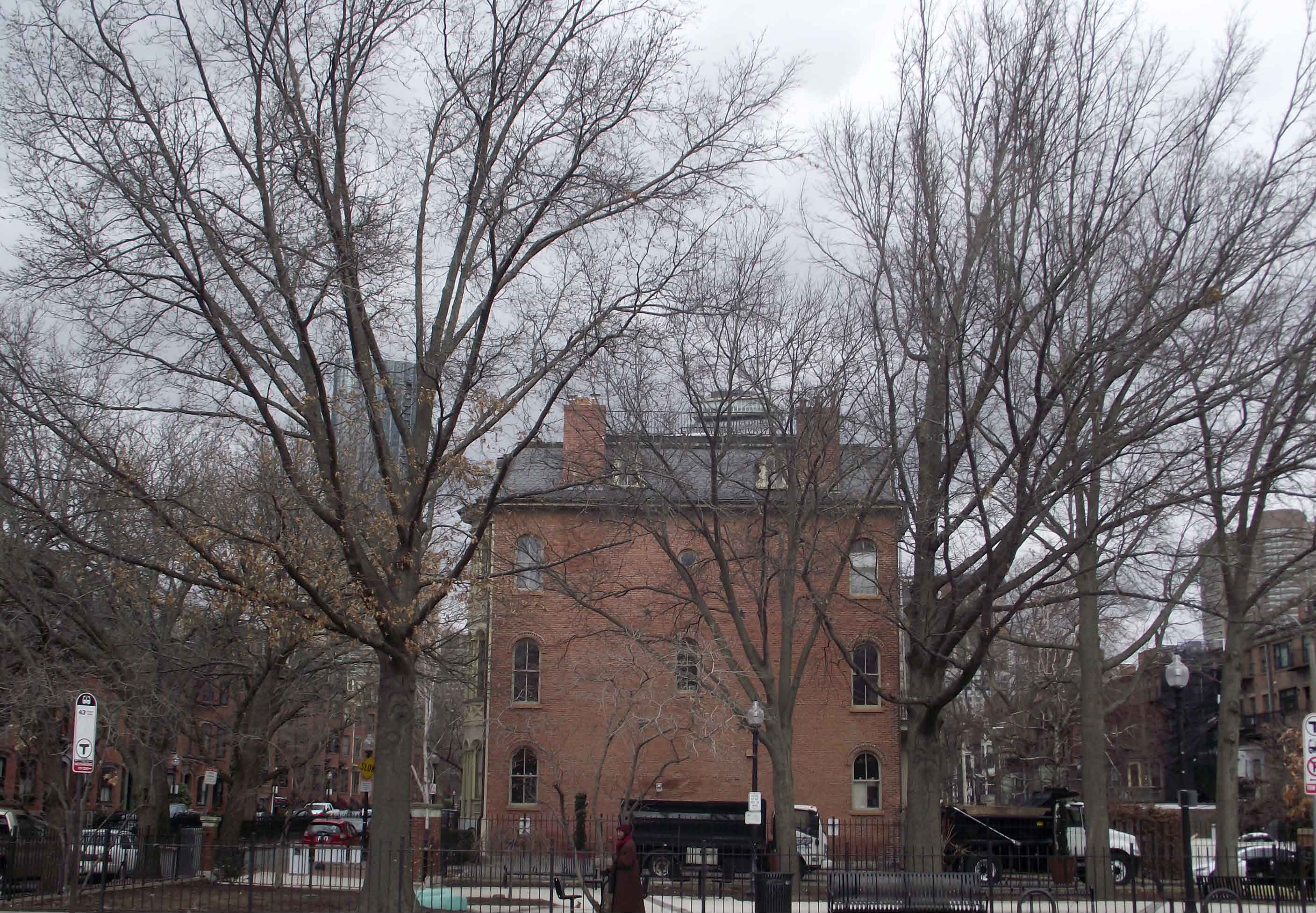
Rooftop Proposed Conditions: View from Tremont Street
