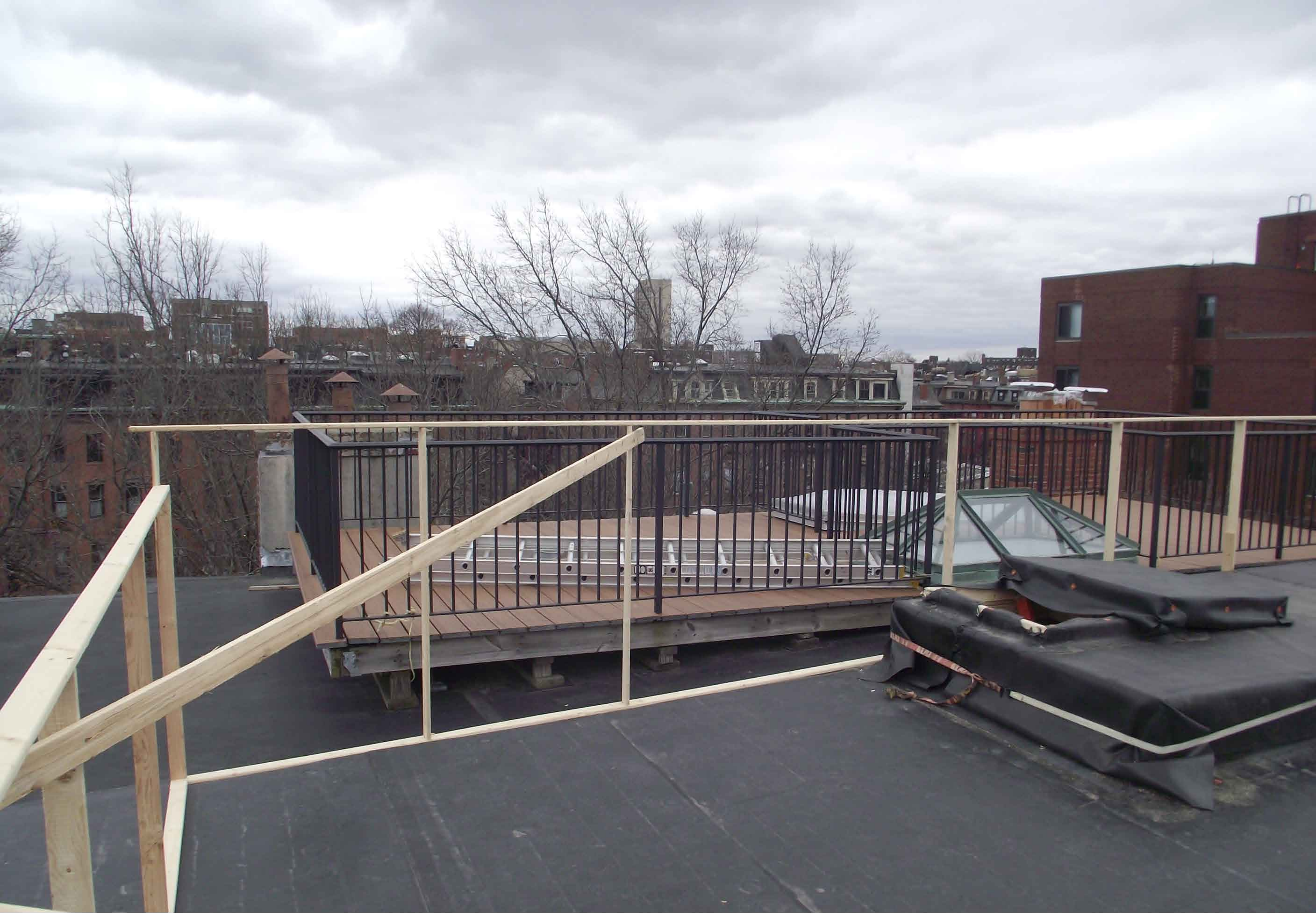
Rooftop Proposed Conditions: View Facing 3 Rutland Sq
