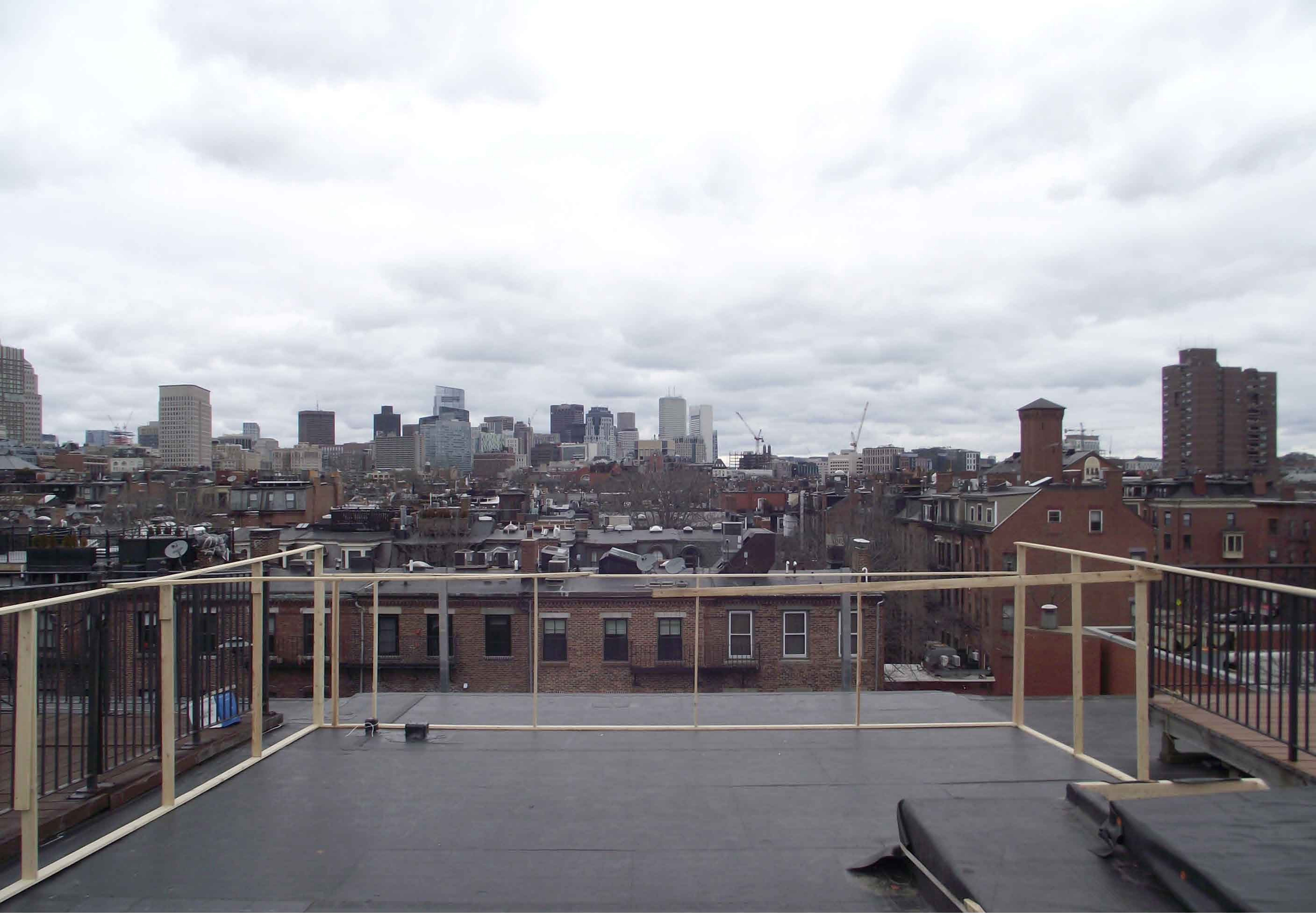
Rooftop Proposed Conditions: View Facing Rear of Building / Back Alleyway
