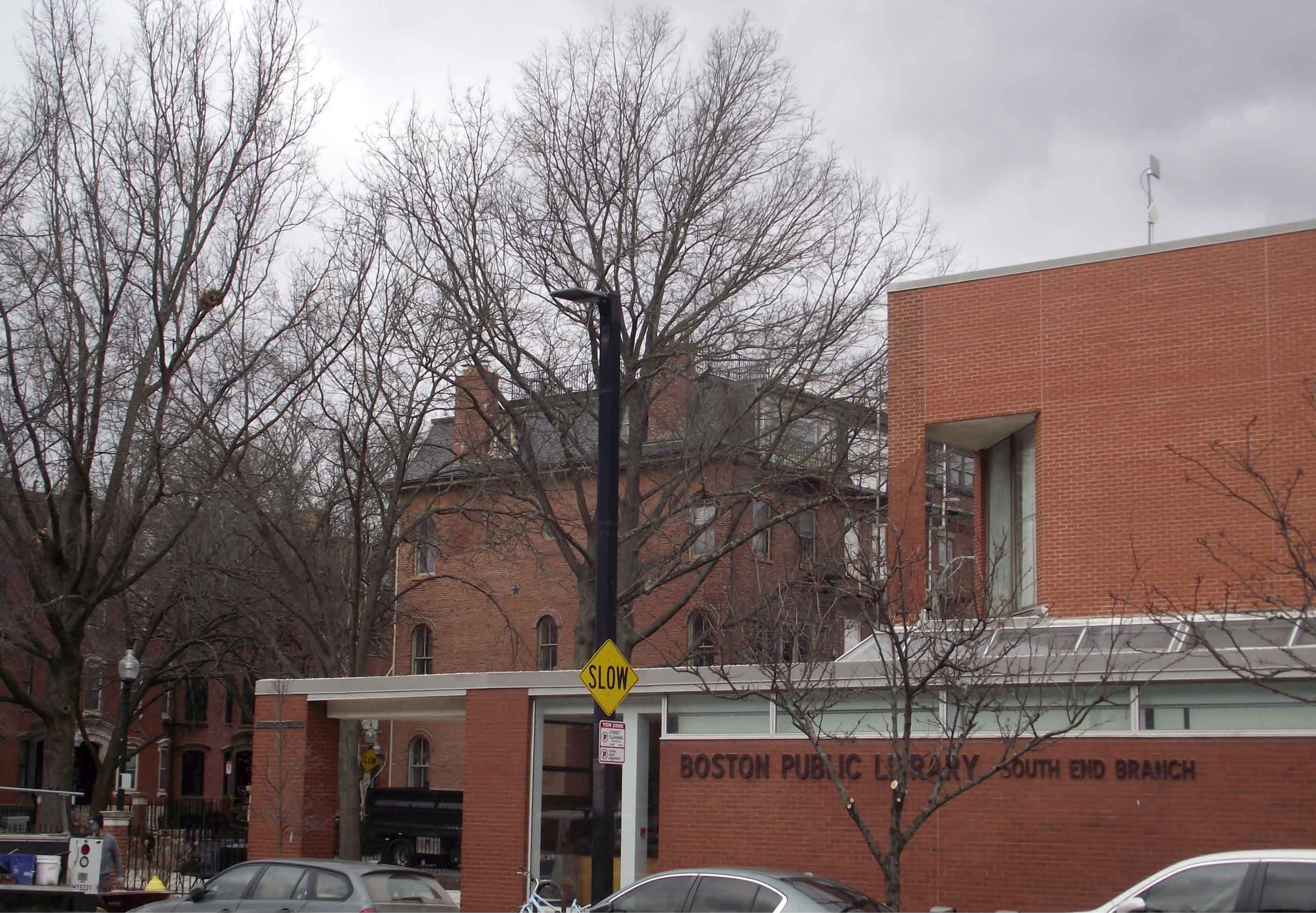
Rooftop Proposed Conditions: View from Tremont Street
