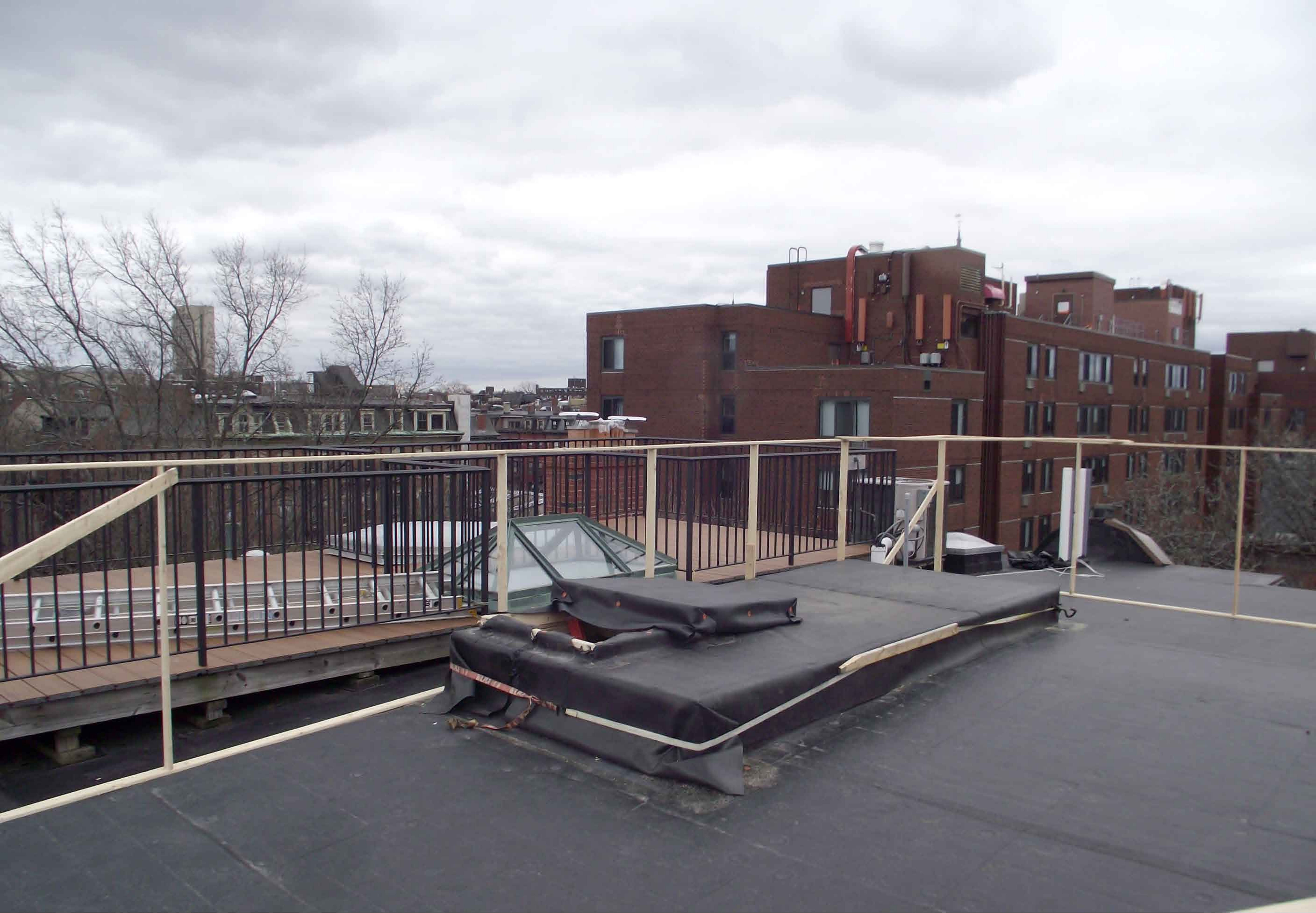
Rooftop Proposed Conditions: View Facing 3 Rutland Sq
