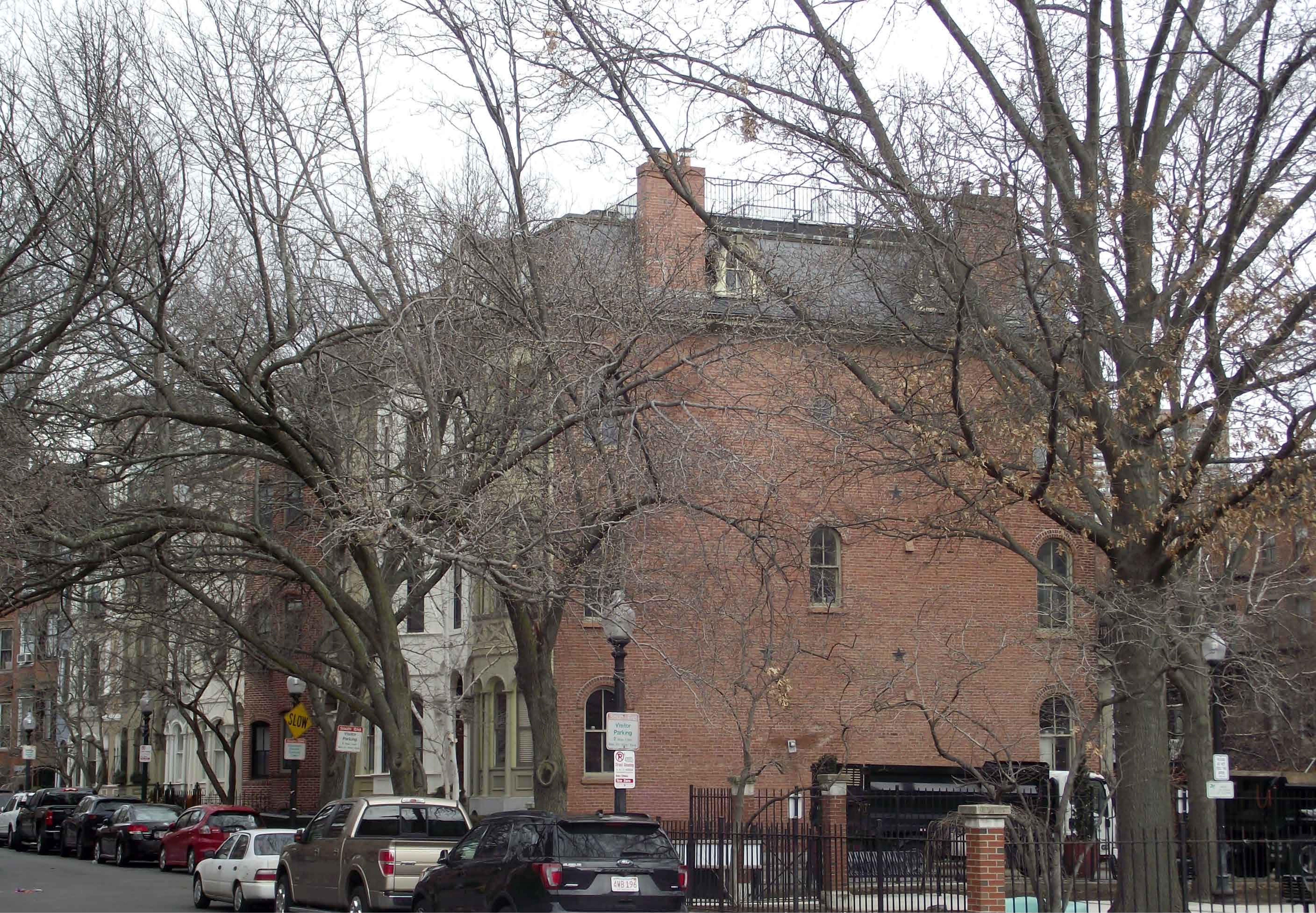
Rooftop Proposed Conditions: View from Tremont Street
