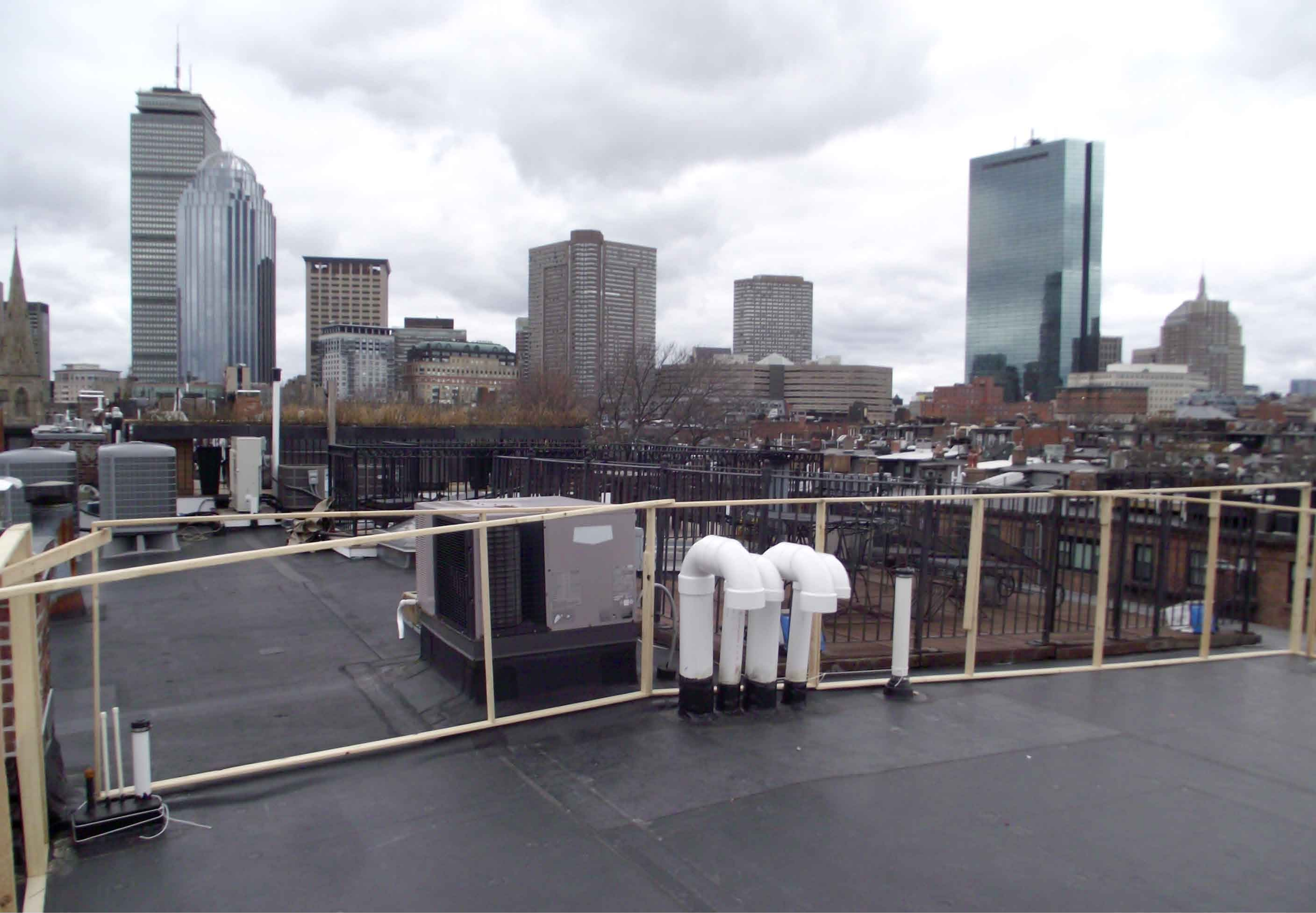
Rooftop Proposed Conditions: View Facing 7 Rutland Sq
