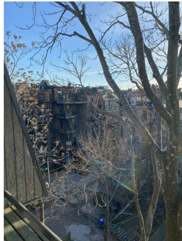
EXISTING PATIO AT MANSARD ROOF
