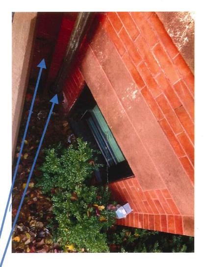
Proposed: Tankless water heater vent either on side of stair or on brick. Vent pipe would be either black iron or made to appear as black iron and mimic the adjoining spout: neighbors have down spouts that go into white PVC- but we would like to make this both aesthetically pleasing and historically pleasing, and make it unobtrusive. We have a large financial investment we would like to maintain and enhance.
