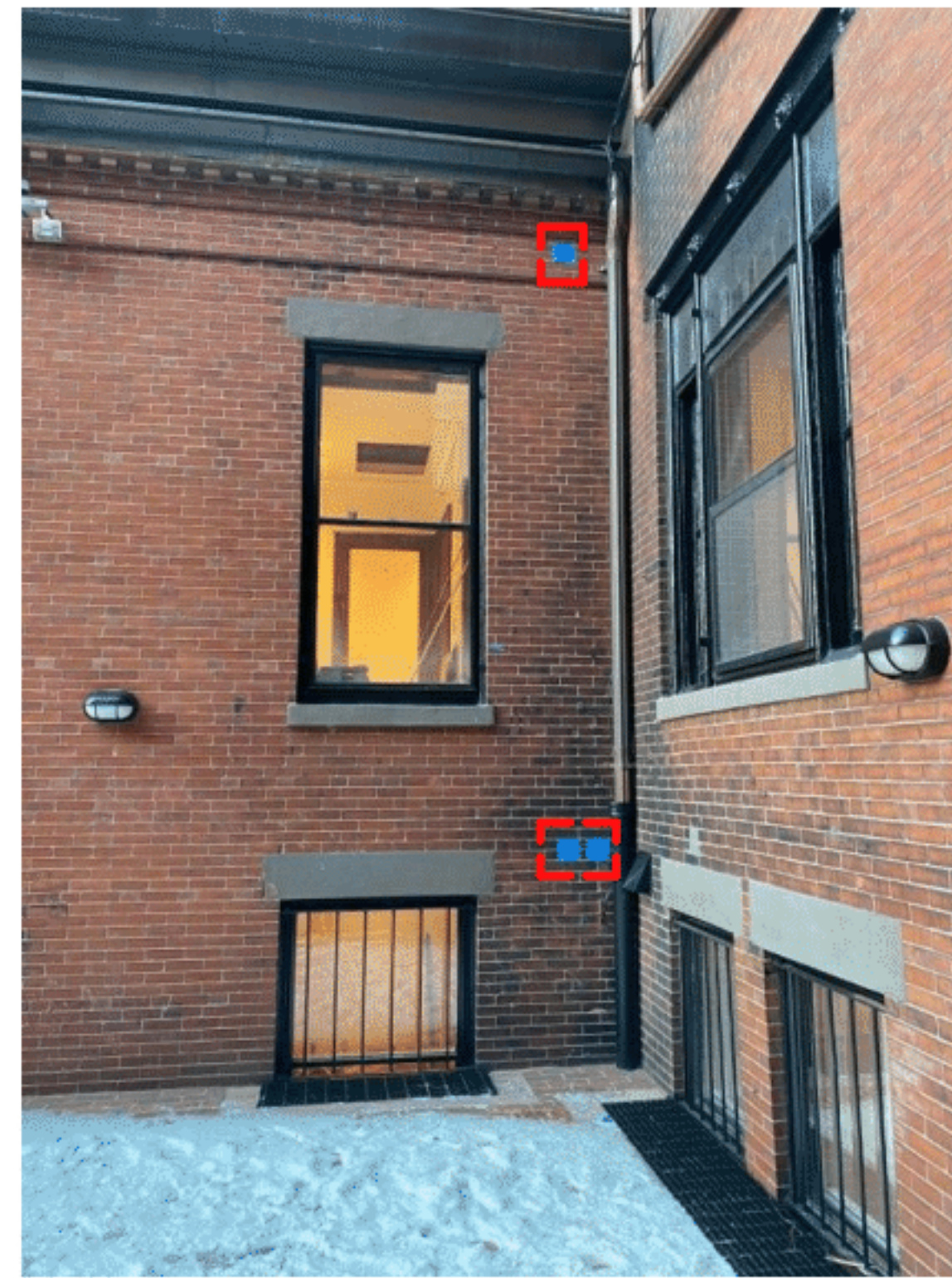
Proposed Rear Wall @ Alley 421 (Blue Tape Marks Location of New Vents)
