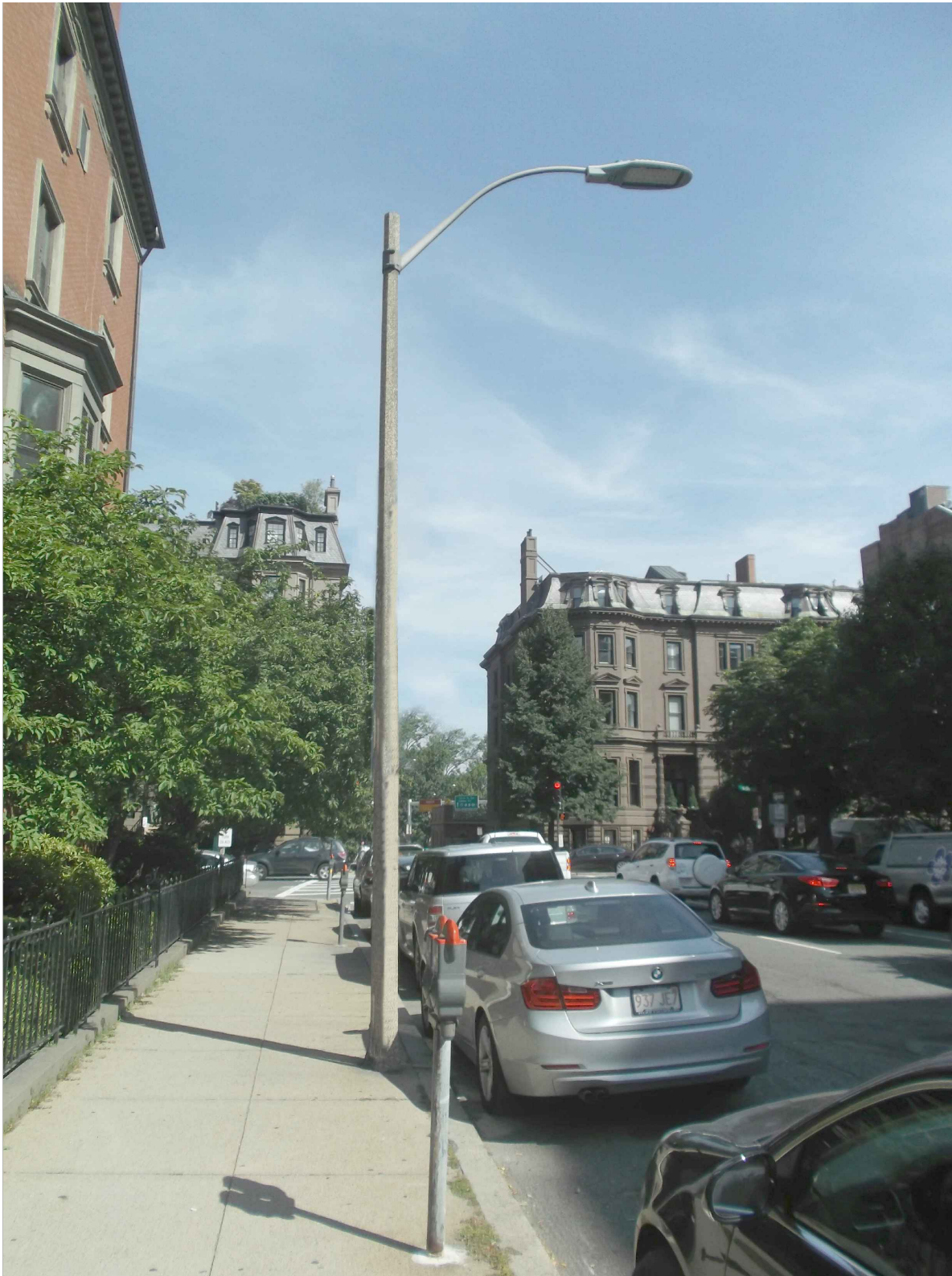
STANDARD CONCRETE LIGHT POLE EXISTING CONDITIONS - EXHIBIT X-1
