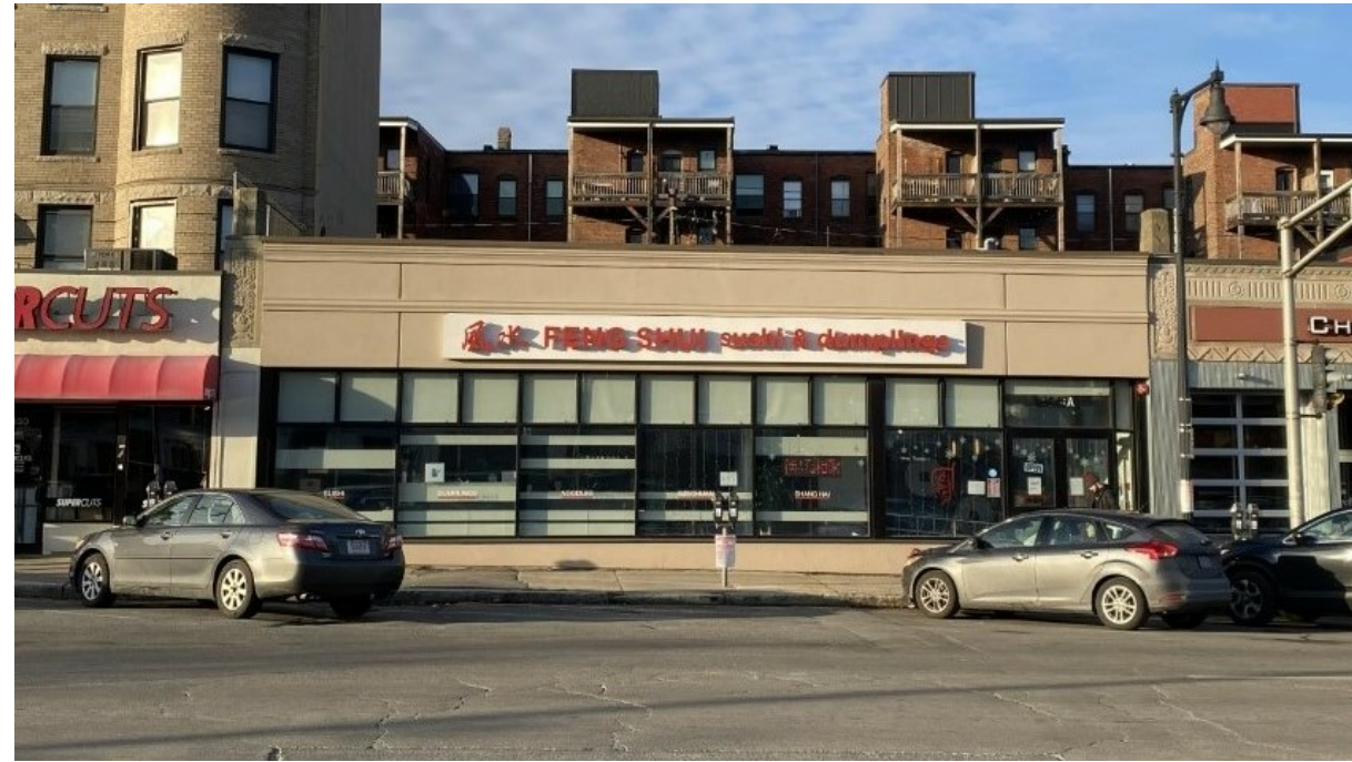
EXISTING FACADE FROM EAST BOUND SIDE OF BEACON STREET
