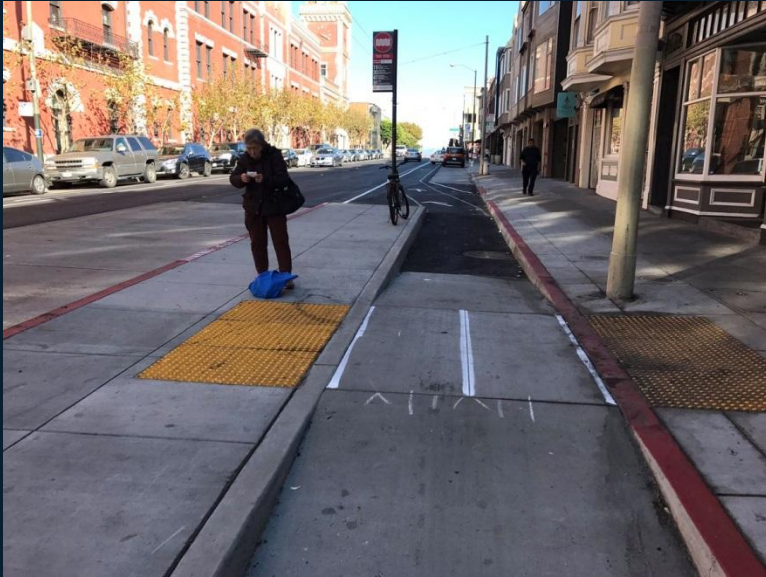
San Francisco (under construction)
