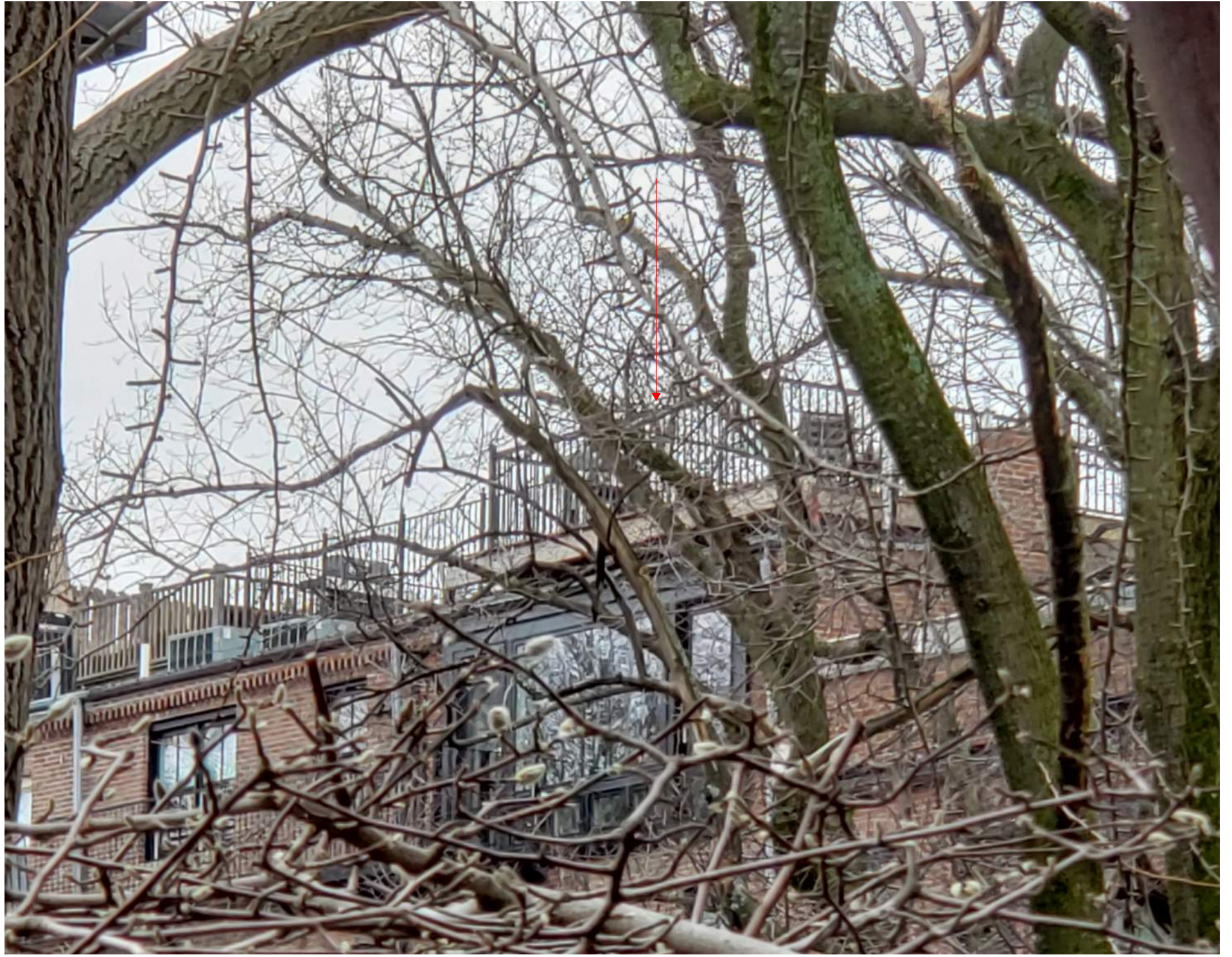
43 Rutland Square Roof Deck - Viewed from West Newton
