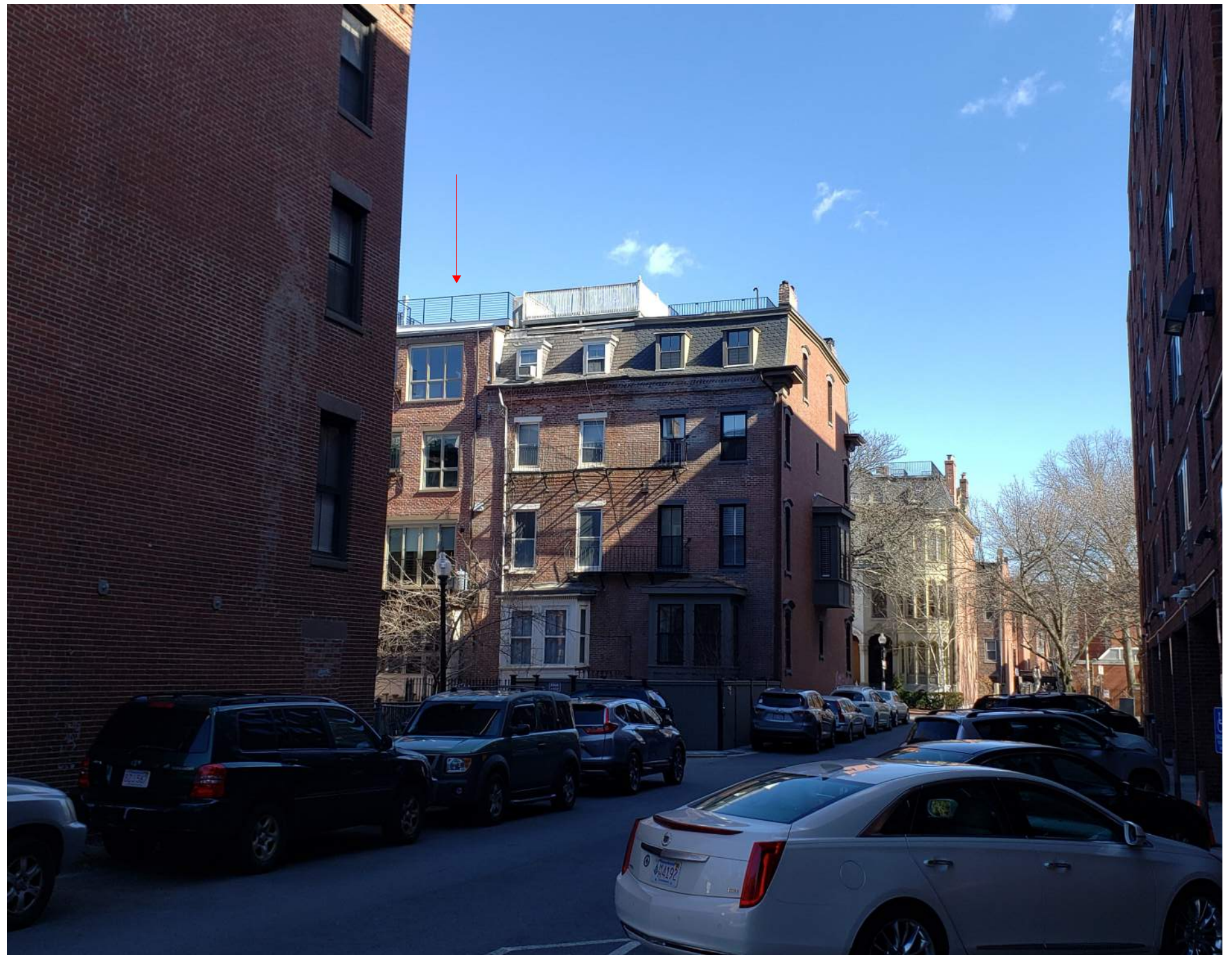
8 Rutland Roof Deck - Viewed from Concord Square
