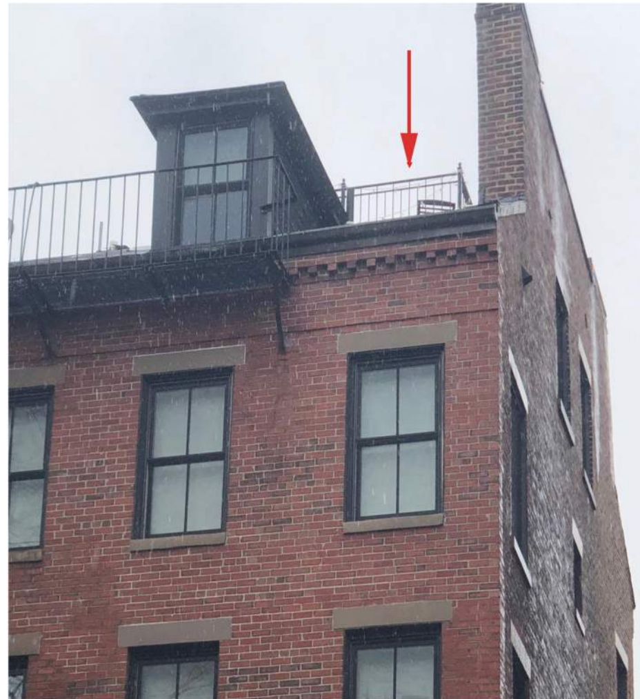
153 West Brookline Roof Deck - Viewed from West Brookline
