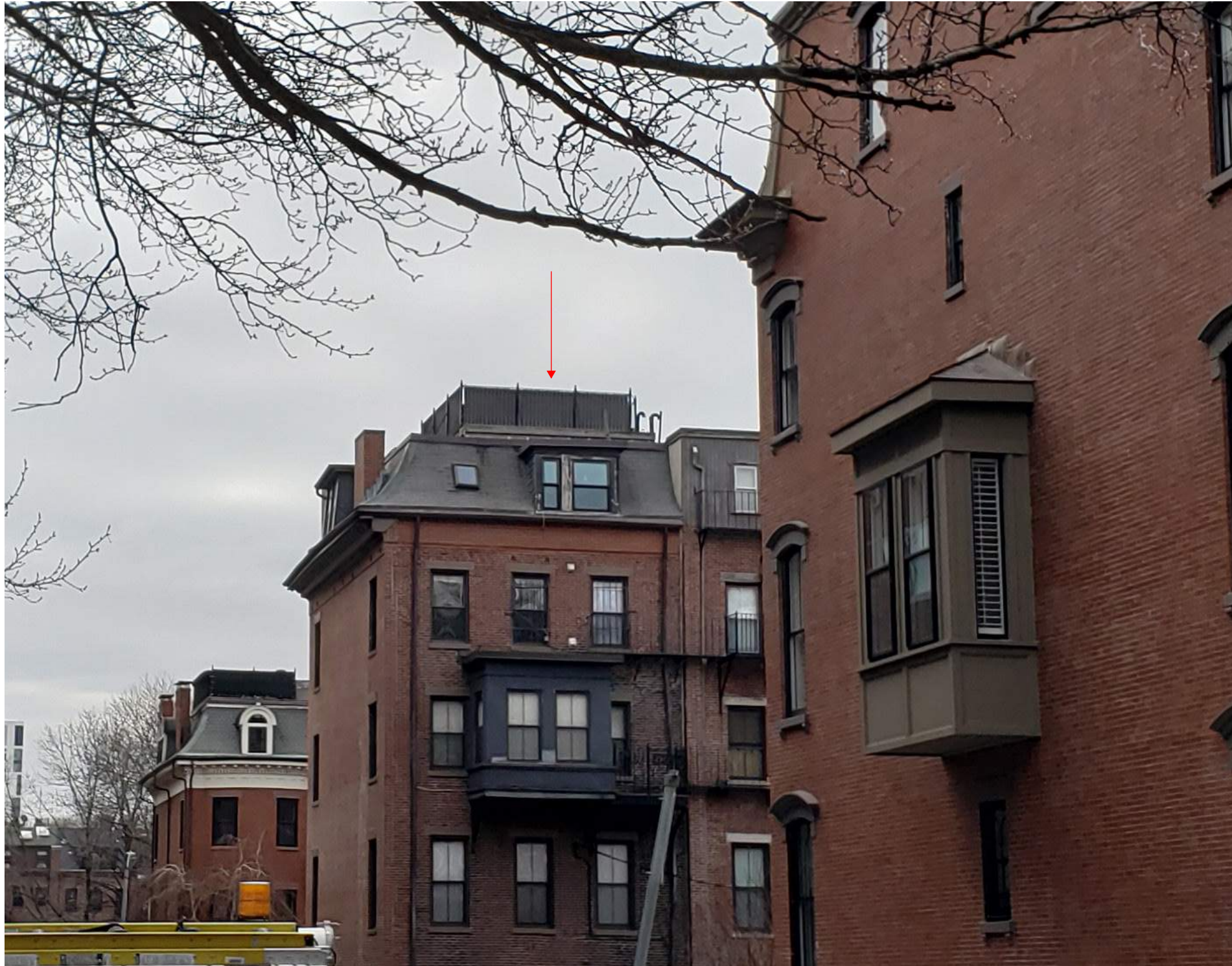
1 Concord Square Roof Deck - Viewed from Rutland Square
