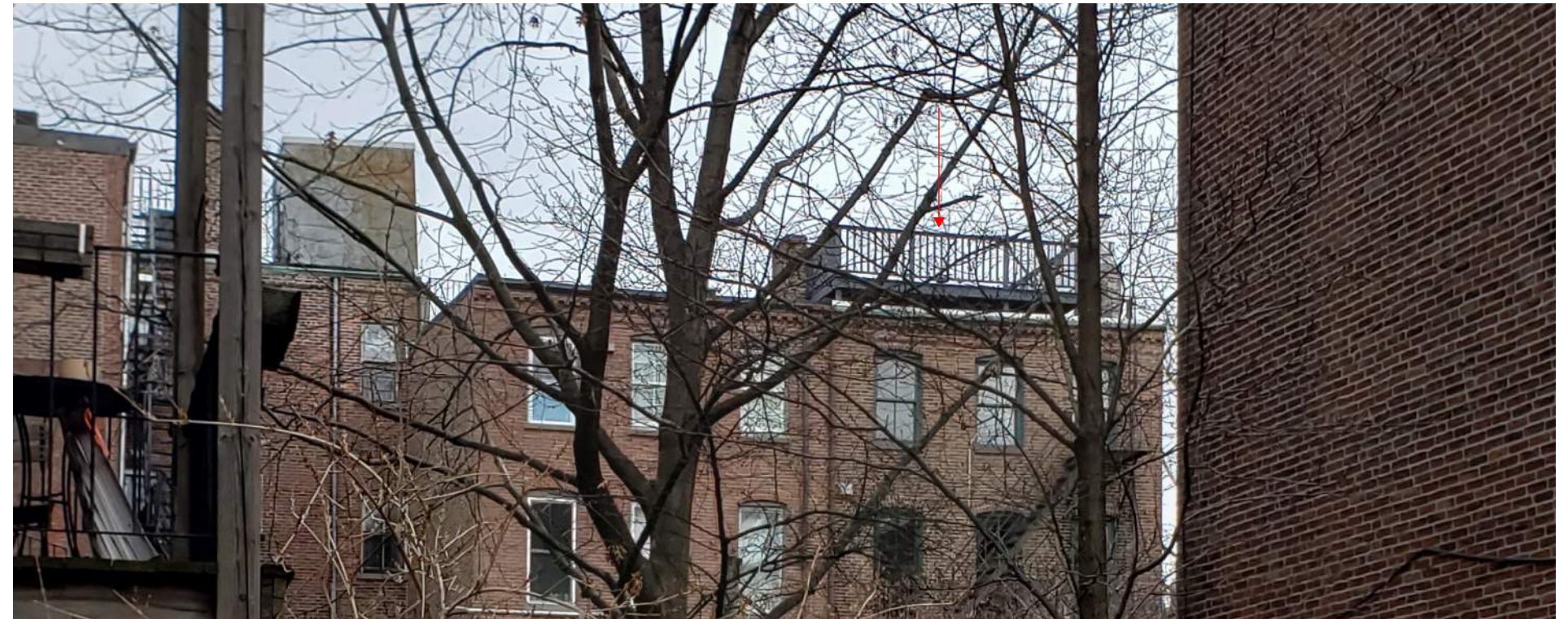
170 West Newton Roofdeck - Viewed from Rutland Square
