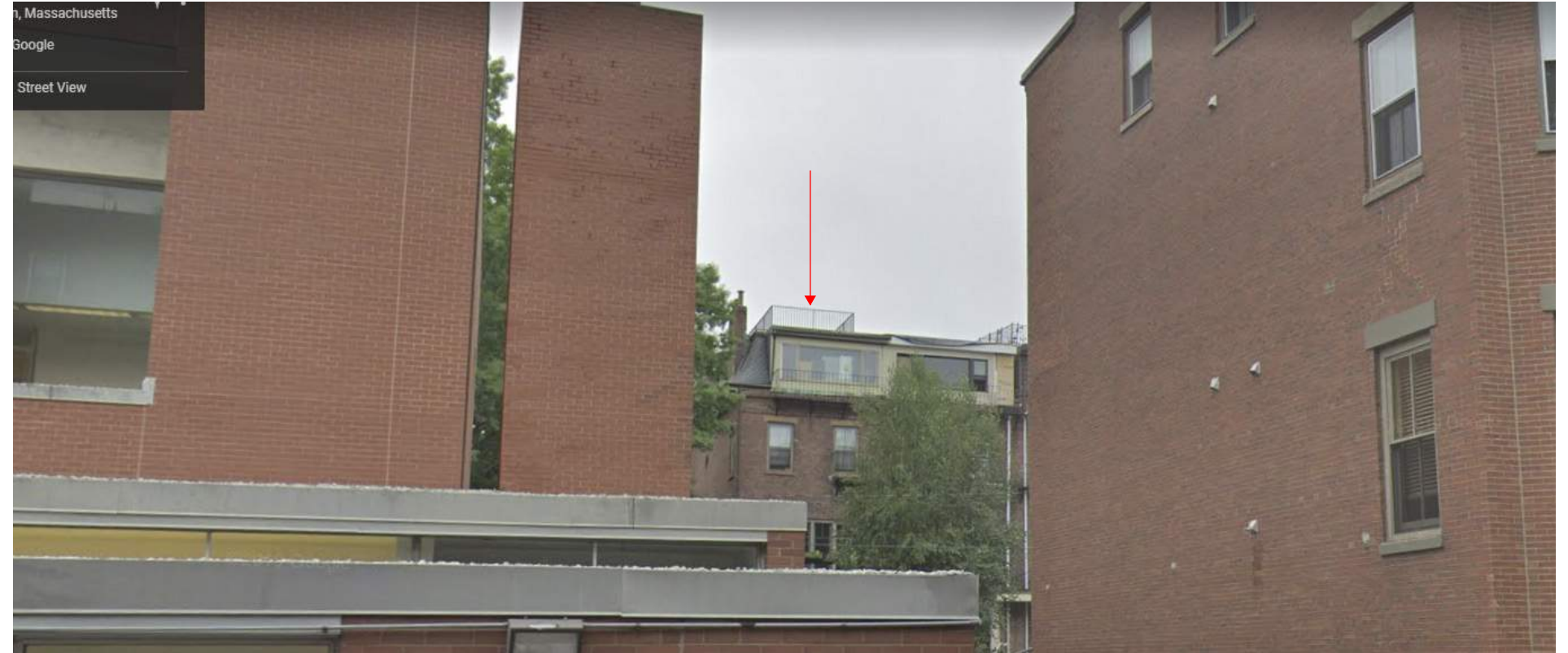
3 Rutland Roofdeck - Viewed from West Newton
