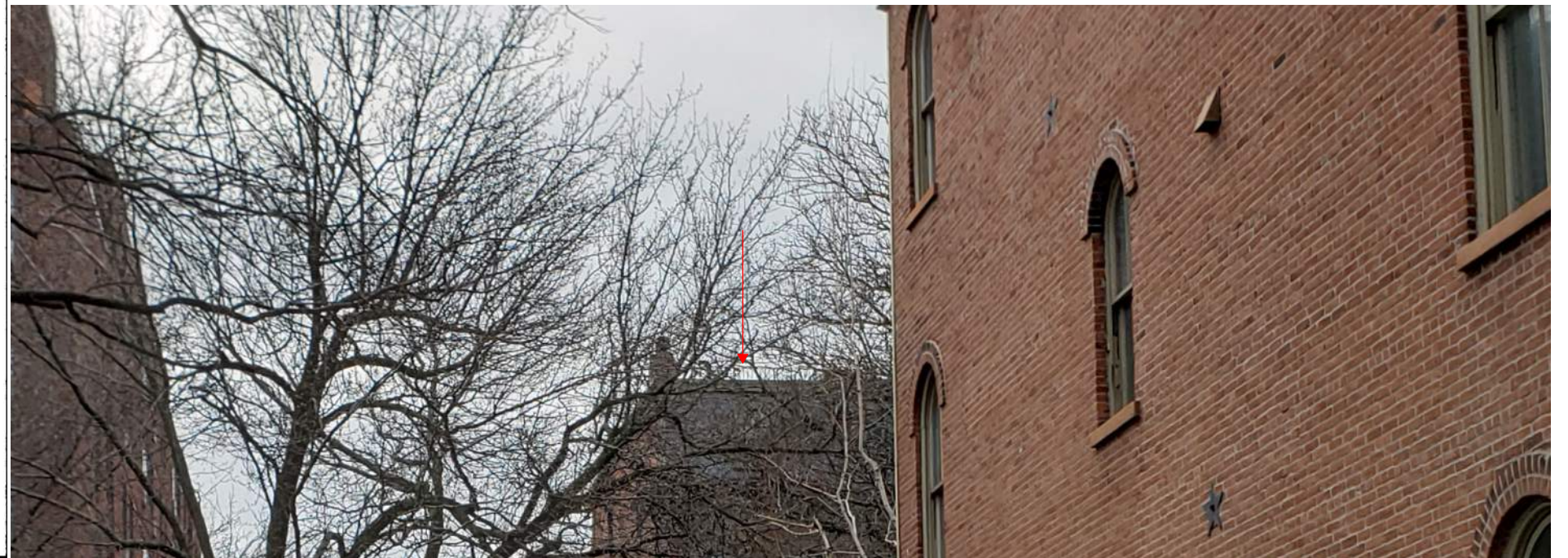
4 Rutland Roof Deck - Viewed from public alley adjacent to 3 Rutland Square
