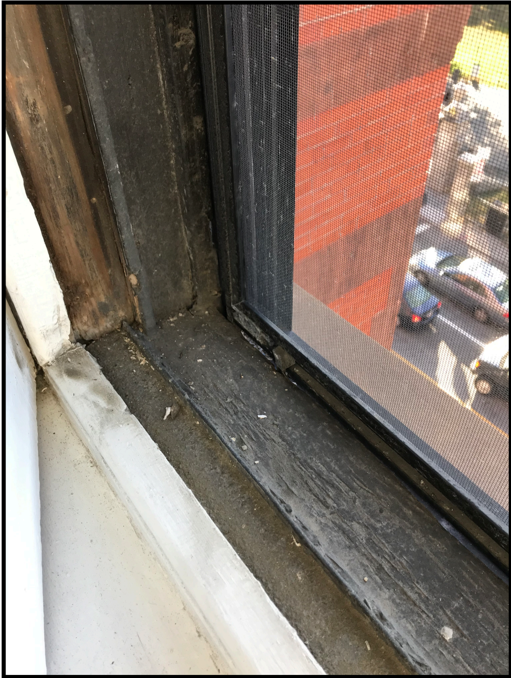
Existing Triple-Track storms on too-short sill
