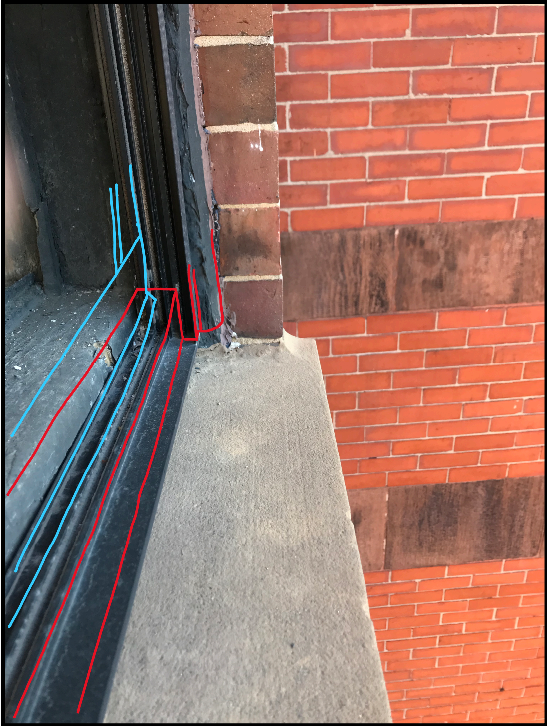
Proposed sill extension (Red) into existing Brick Mold Proposed location of storm window bottom edge (Blue)
