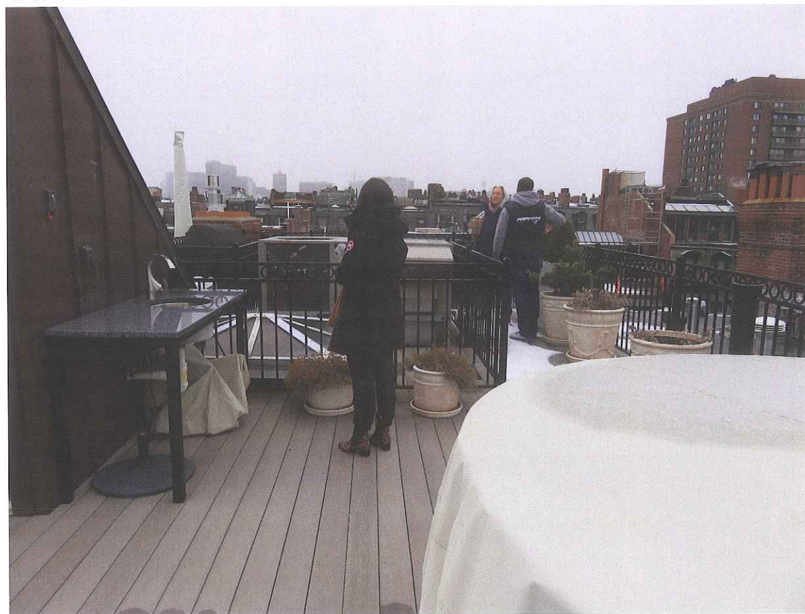
EXISTING ROOF DECK - SKYLIGHT
