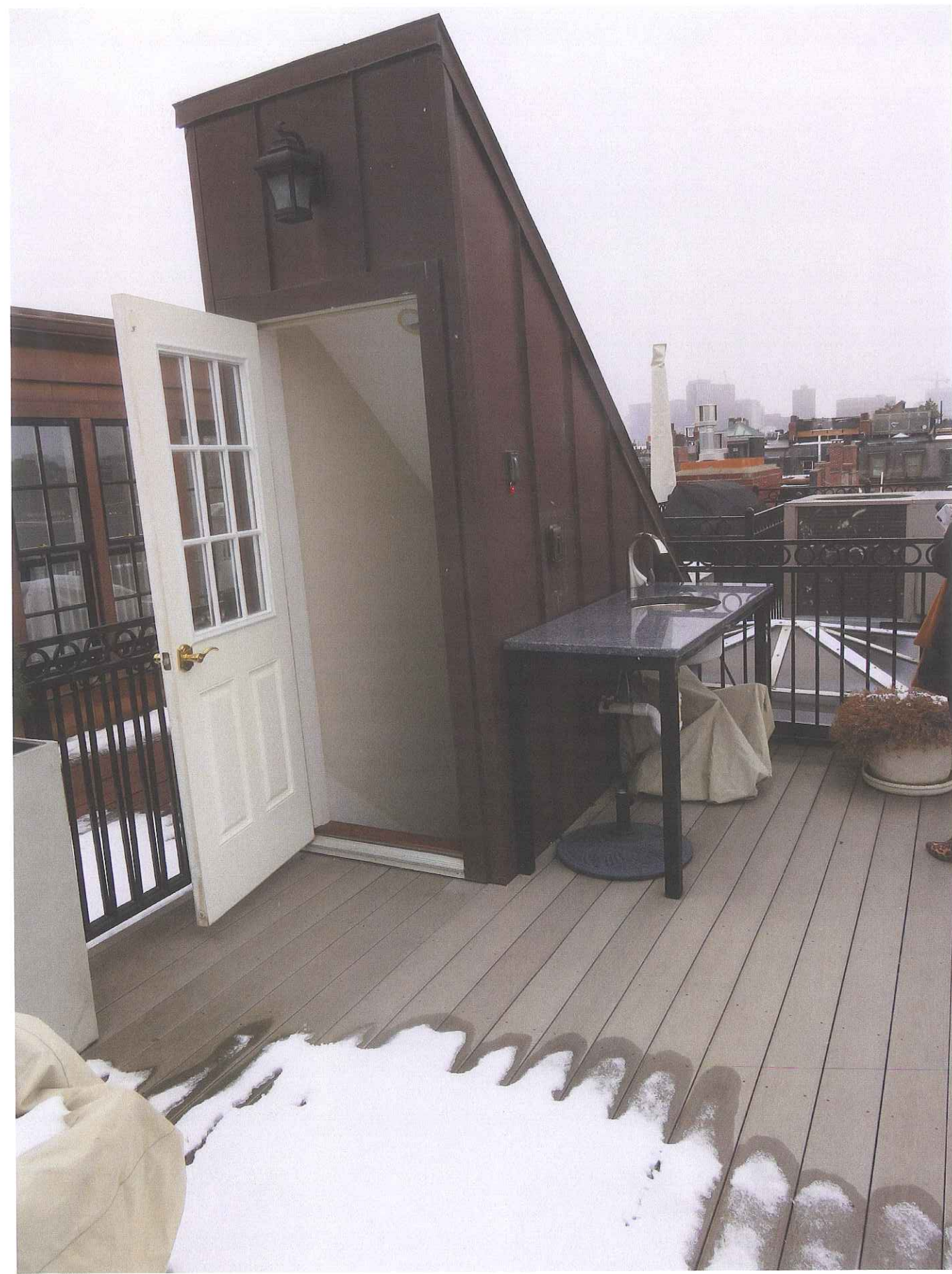
EXISTING ROOF DECK - HEADHOUSE
