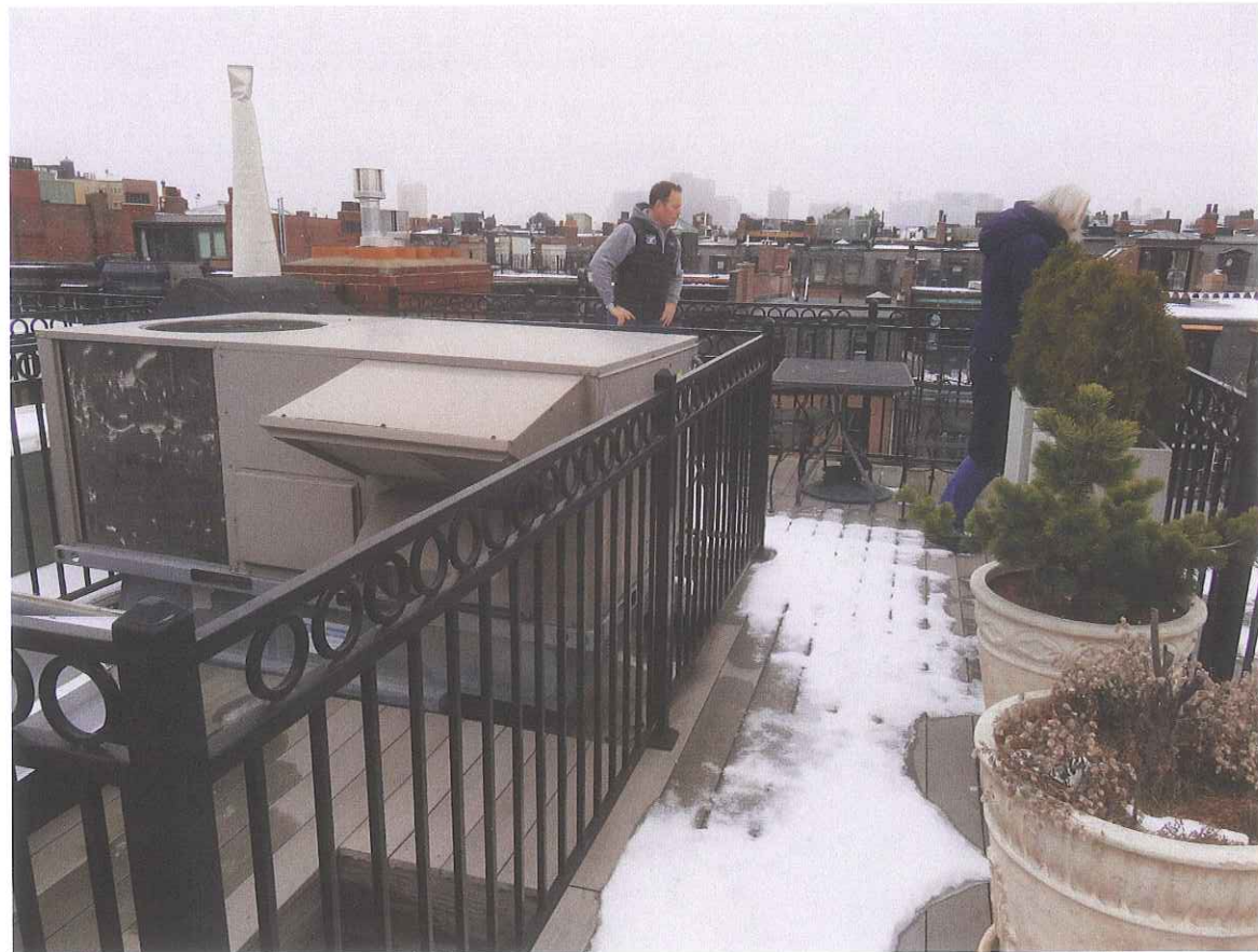
EXISTING ROOF DECK - MECHANICAL
