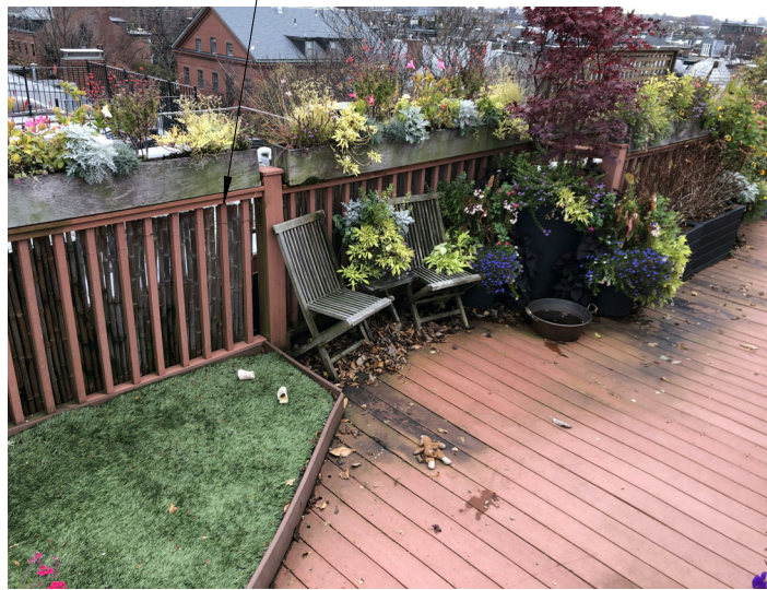
EXISTING COMPOSITE RAILINGS
