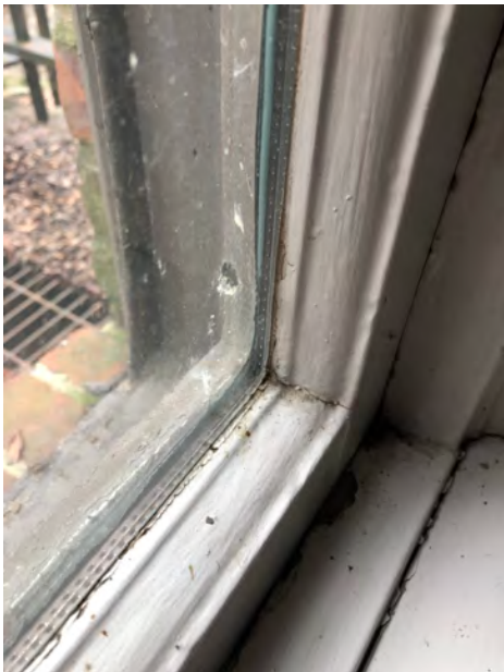
Interior Detail of Double-Hung Sash at Rear Facade
