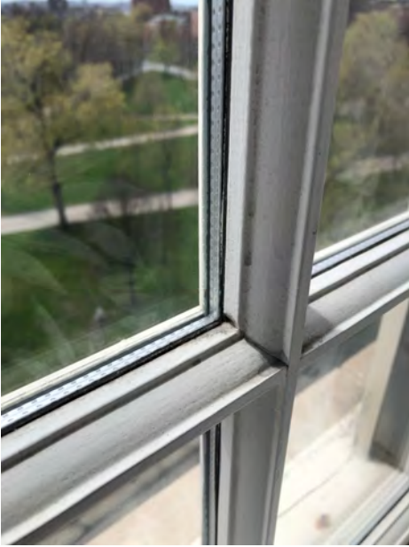
Clear Insulated Glass from 1997 at Front Facade; Clear Aluminum Spacers Used Due to White Exterior (Dark Spacers Would Result in SDL Appearance)
