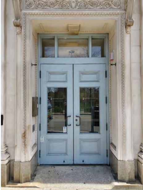
Recessed Entrance to 3 Park Street with Granite Plinth and Limestone Surrounds
