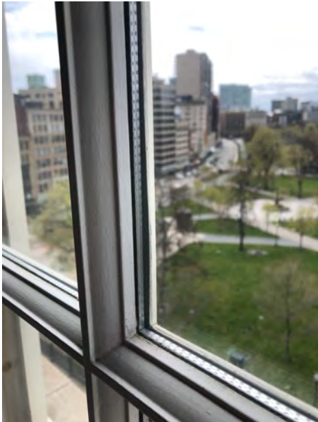
Interior Detail of 8/8 Wood True-Divided Light Double-Hung Window Sash on Park Street Facade
