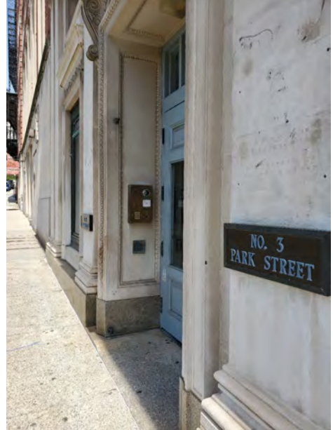
Looking Up Park Street in Direction of State House; Existing Video Door Intercom System on Jamb
