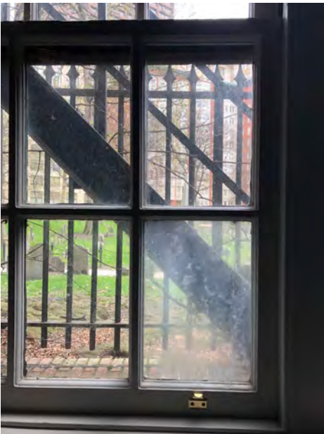
Fogged Appearance Due to Trapped Moisture; Failed Seals on Some Individual Lights
