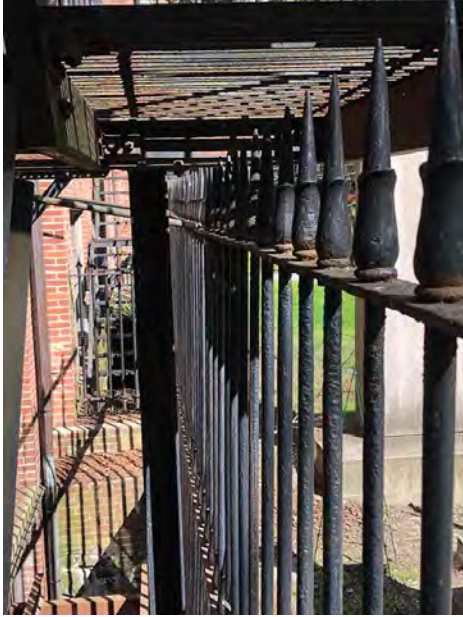
Wrought Iron Fence Below Grating at Second Floor Landing
