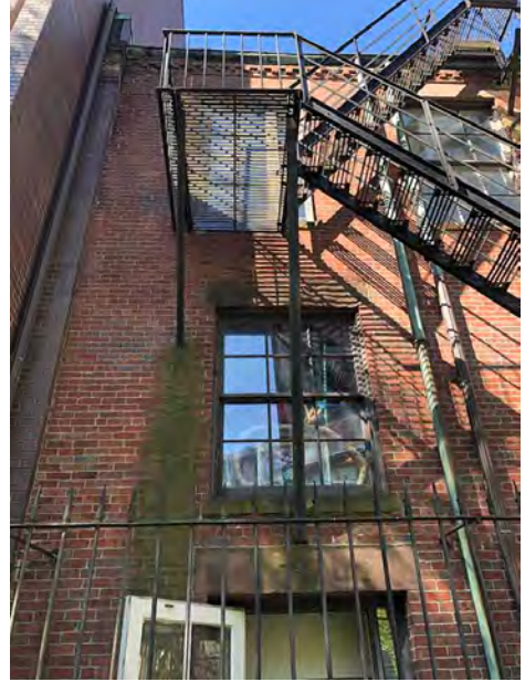
Landing at Third Floor Supported by Pair of Brackets
