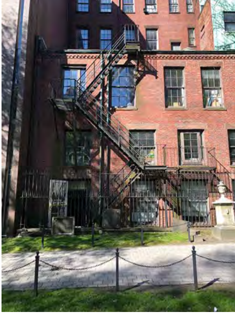
Fire Escape at Rear Facade of 2 Park Street Serving Floors 1, 2, 3 and 4
