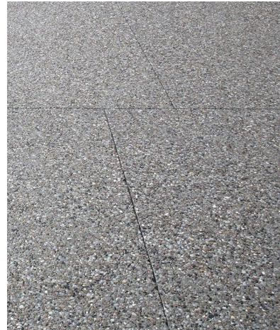
Seeded Concrete Walkway & Boulders in Stone Drainage Bed
