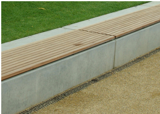
Seatwall / Bench Concrete Base with Wood Top
