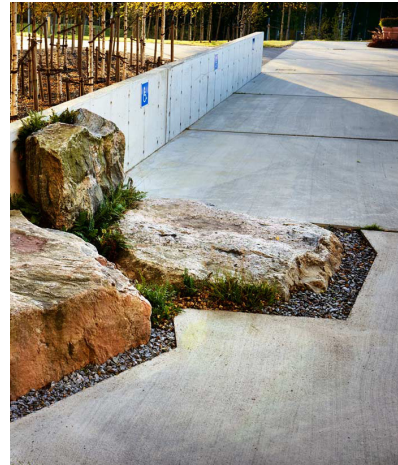
Seeded Concrete Walkway & Boulders in Stone Drainage Bed
