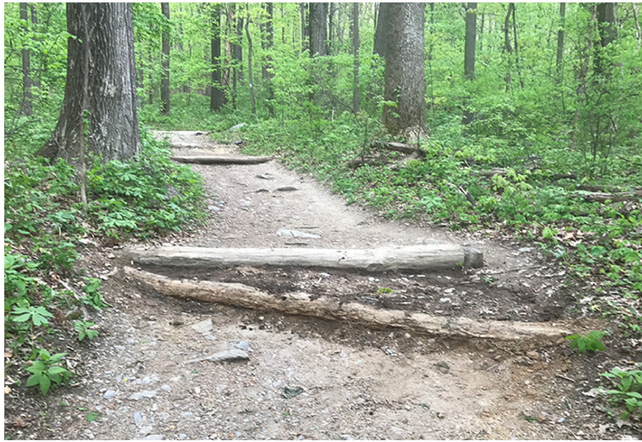
1. Water Bars (Divert Water Off Path)
