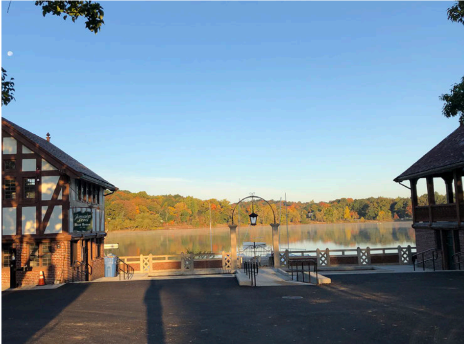
Boathouse Plaza following flagpole removal under Certificate of Design Approval, 19.551.142, Emerald Necklace, Phase 2
