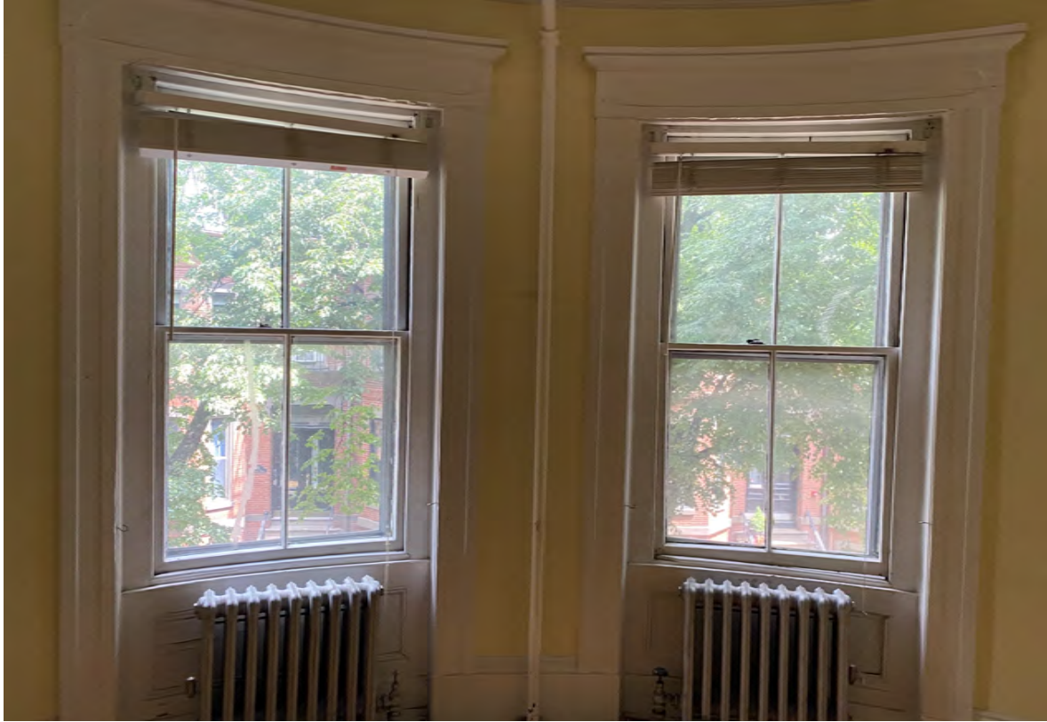
SECOND LEVEL CURVED SASH WOOD
