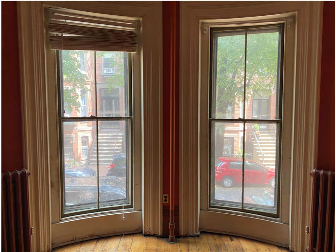
PARLOR LEVEL CURVED SASH WOOD
