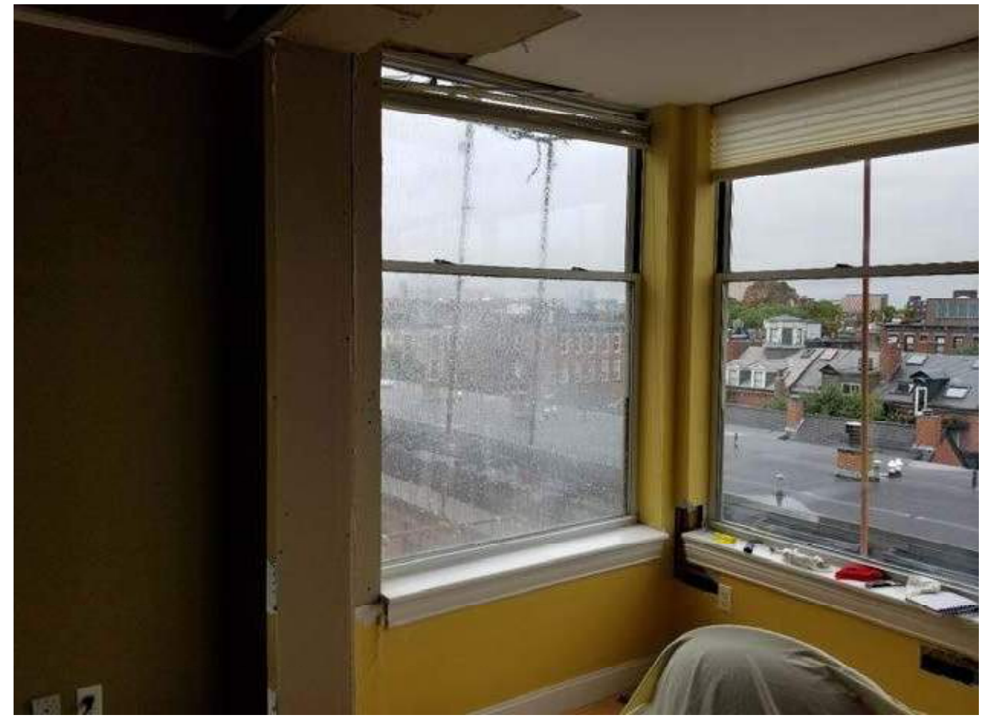
TYPICAL EXISTING DOUBLE HUNG WINDOWS Interior View
