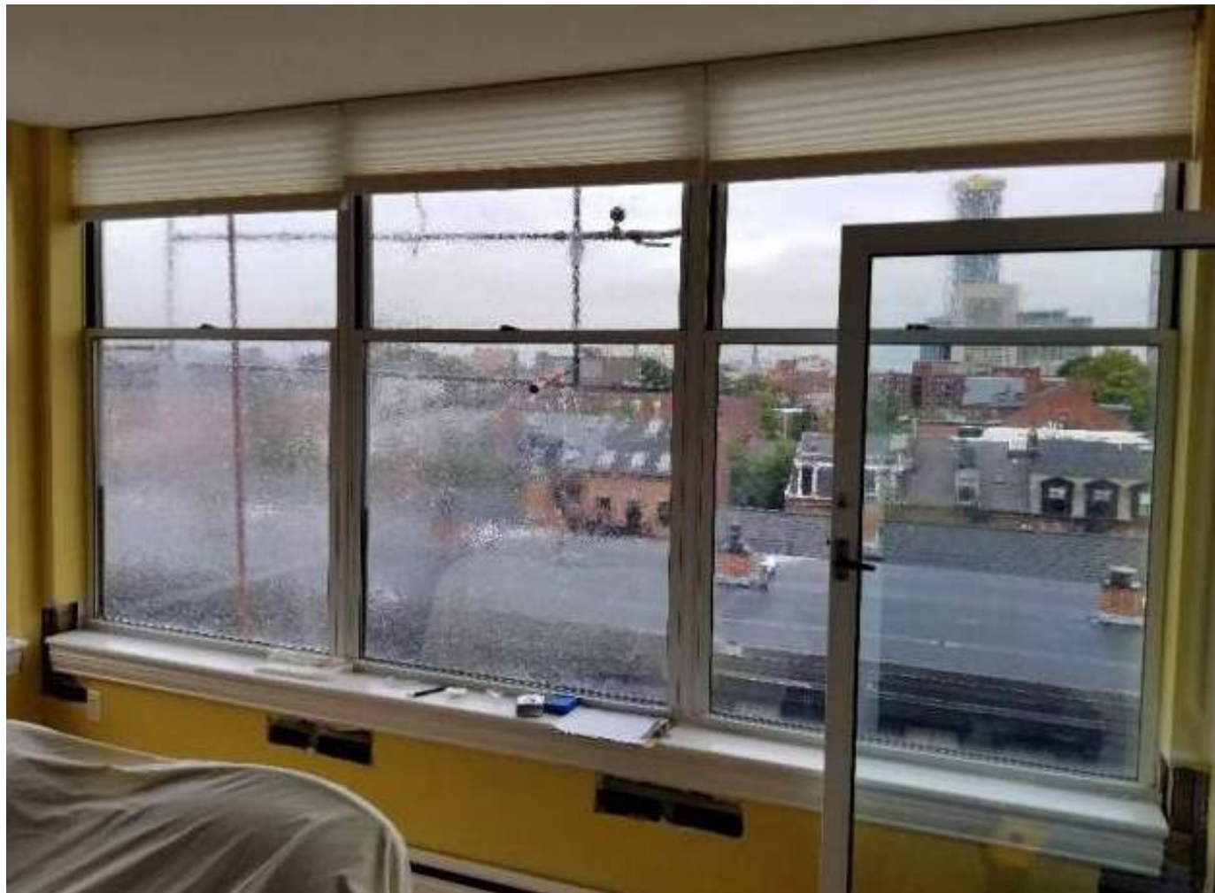
TYPICAL EXISTING DOUBLE HUNG WINDOWS Interior View
