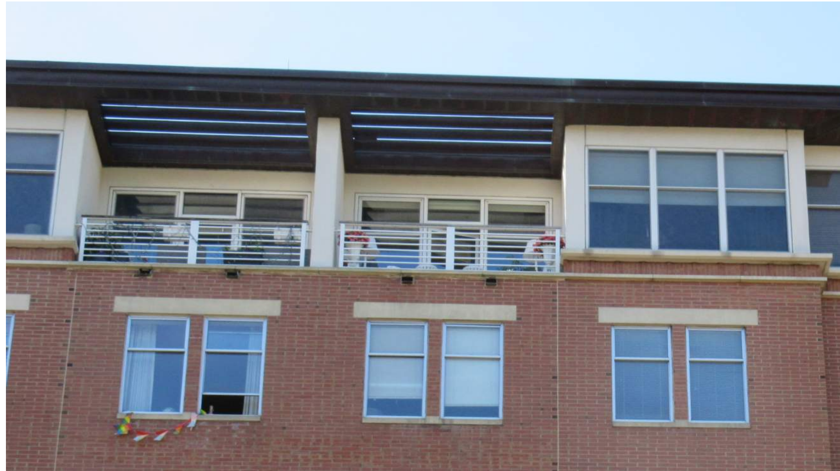
TYPICAL EXISTING WINDOWS and TERRACE DOORS Washington Street View
