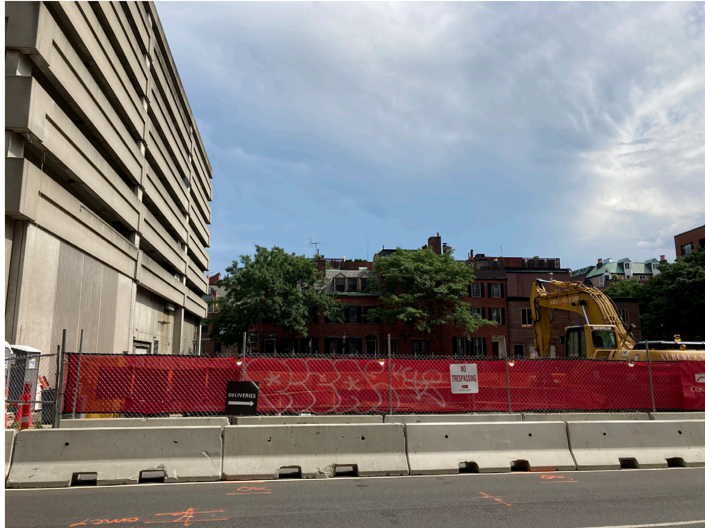
View of Existing Construction Site for New Residential Tower (212 Stuart Street)
