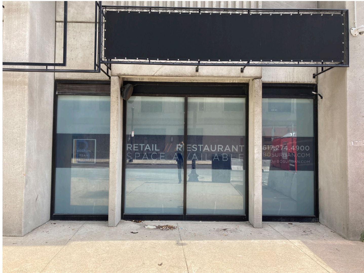
Detail View of Existing Storefront (Future Tenant Side)
