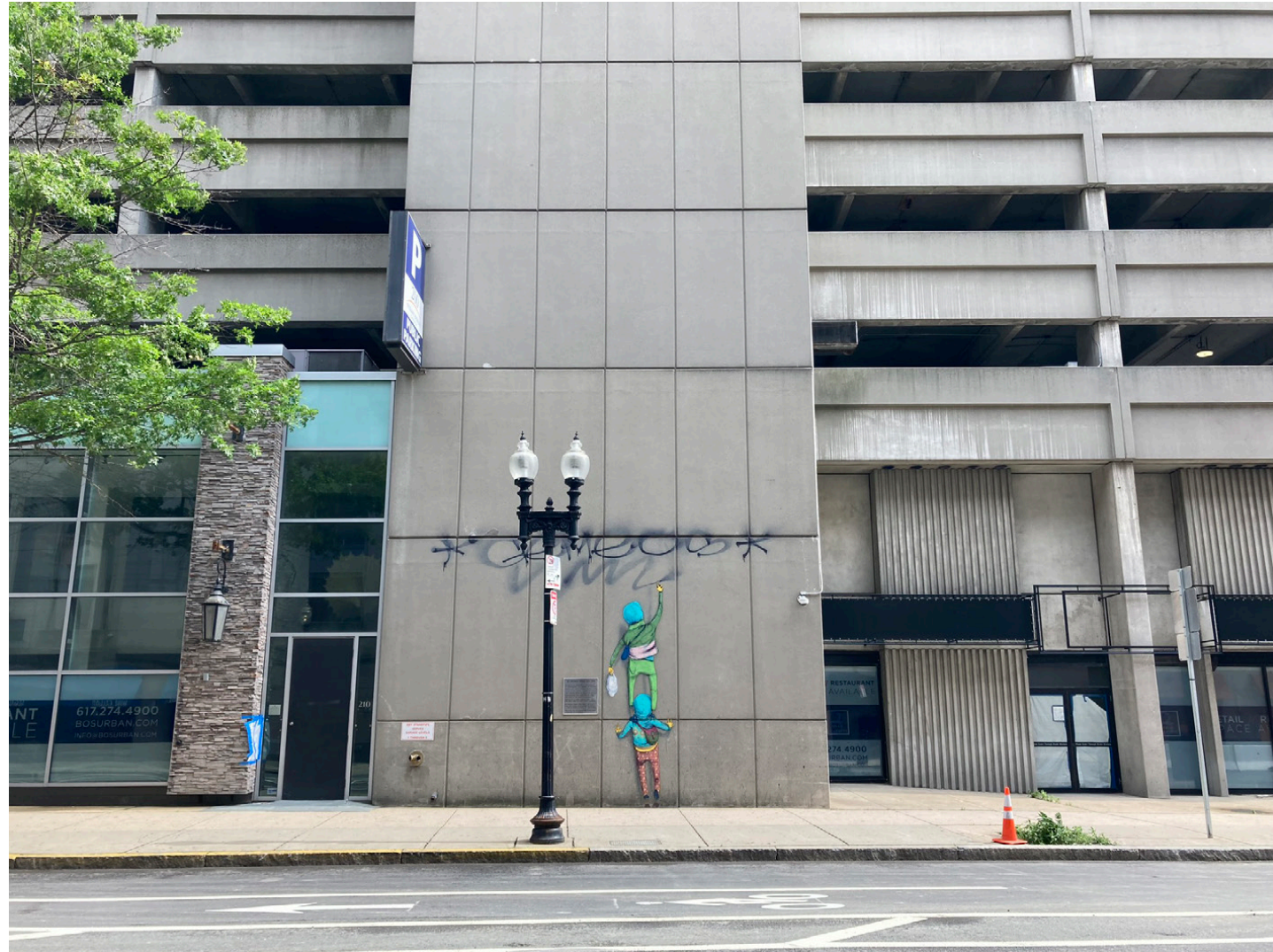
View of Existing Graffiti on Garage Egress (To be preserved and lit)
