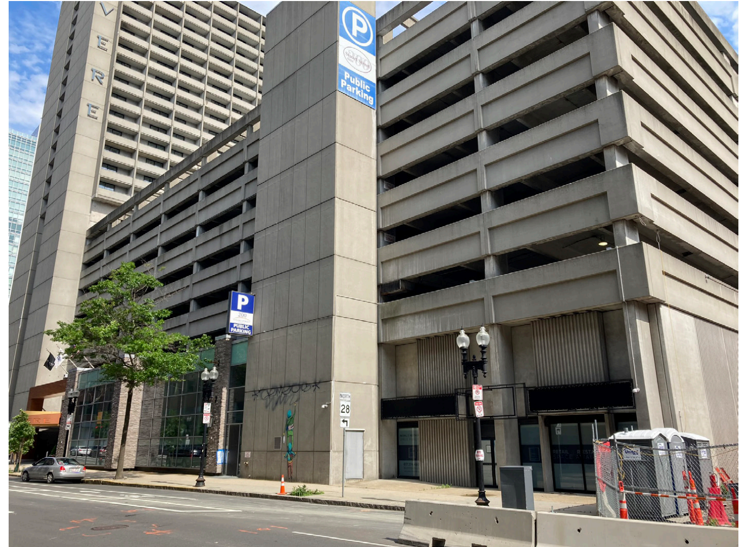
View from Stuart Street of Existing Retail Storefront (Future Tenant Side)
