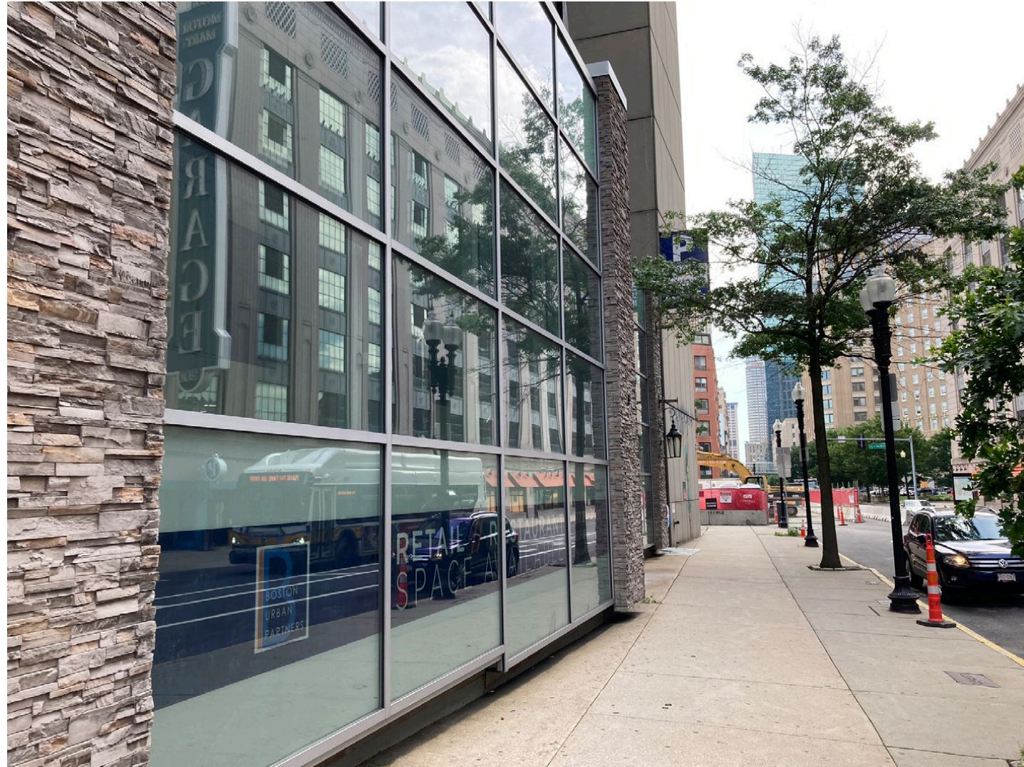
Detail View of Existing Storefront (Minoti Side)
