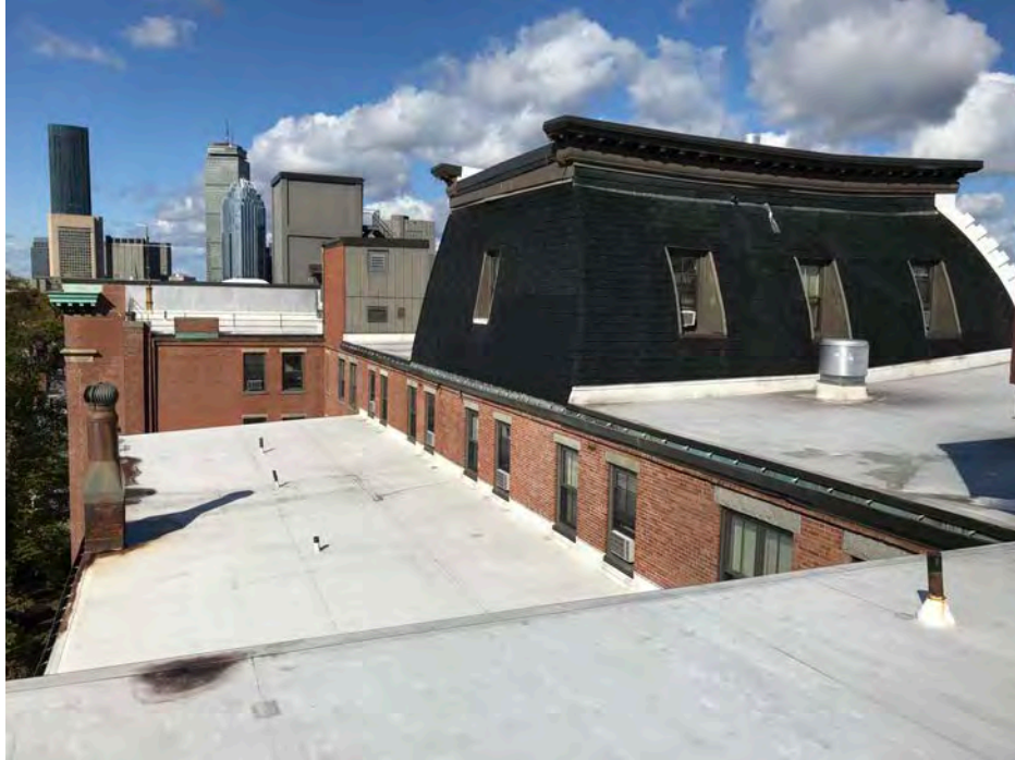
View facing north
