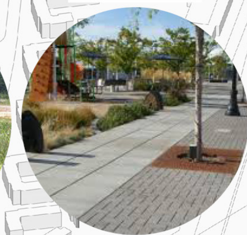
TREE TRENCH + POROUS PAVING
