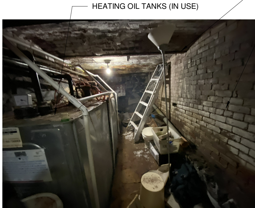
PHOTO ENTERING INTO VAULT UNDER ENTRY STAIR/WALK, LOOKING TOWARD BERKELEY ST.
