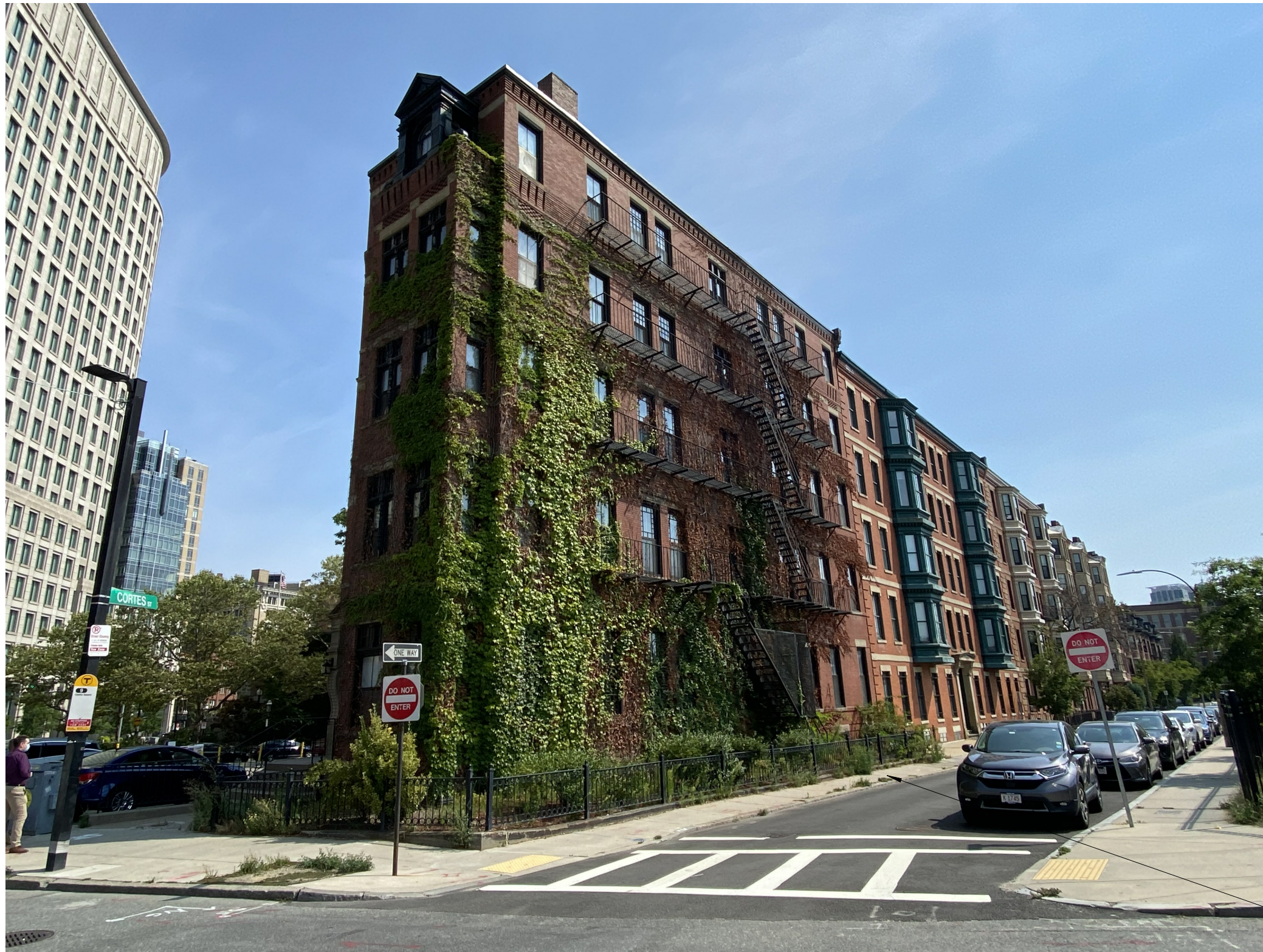
OVERALL FROM STREET CORNER
