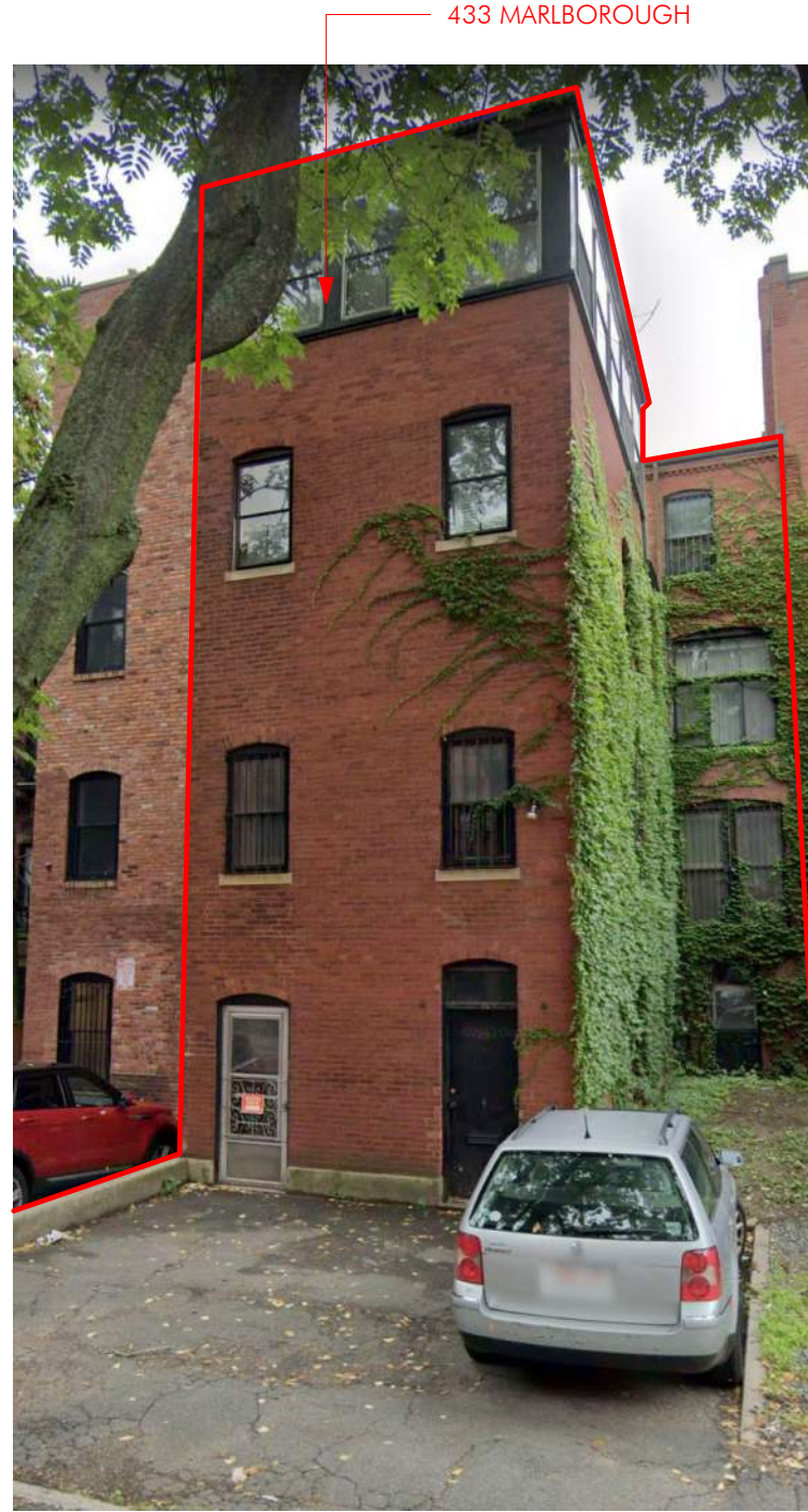
433 MARLBOROUGH ST REAR FACADE
