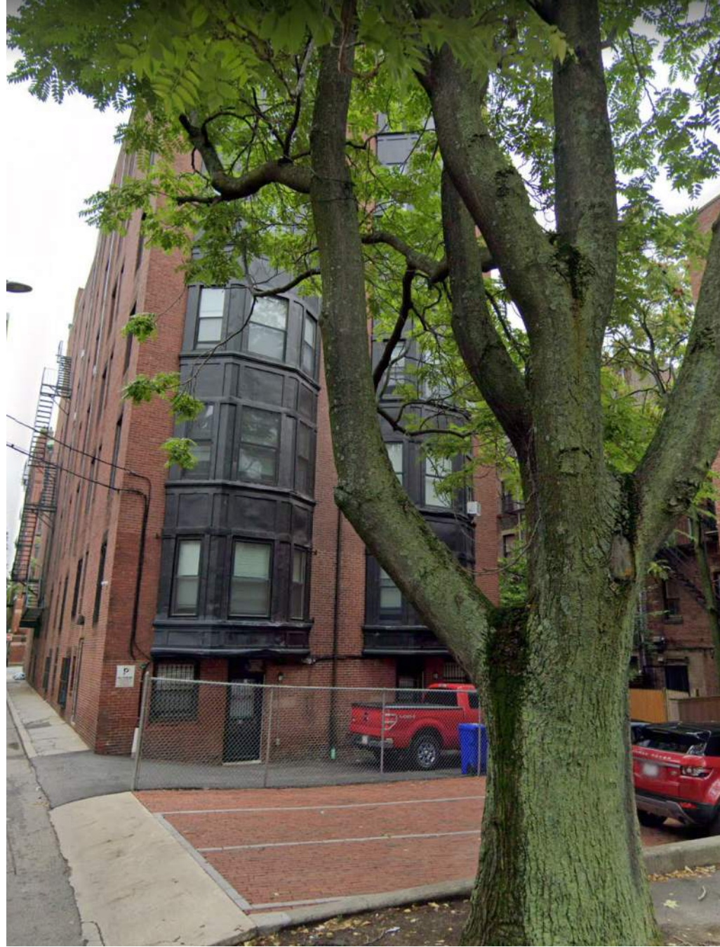
PUBLIC ALLEY 908 LOOKING EAST
