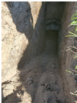
Figure 1: Completed Test Pit - View 1
