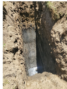
Figure 2: Completed Test Pit - View 2
