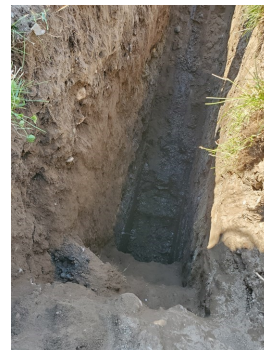
Figure 2: Completed Test Pit - View 2
