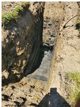
Figure 1: Completed Test Pit - View 1
