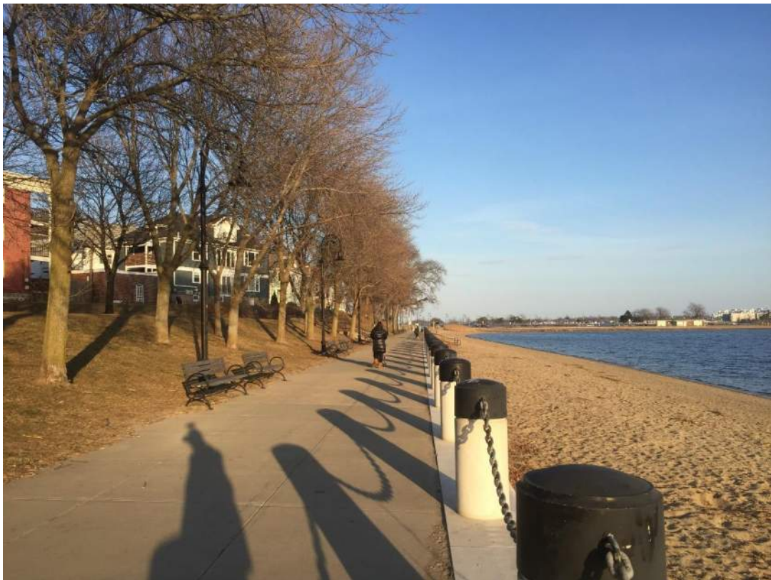
Photo 2: Retaining Wall Adjacent to Coastal Beach
