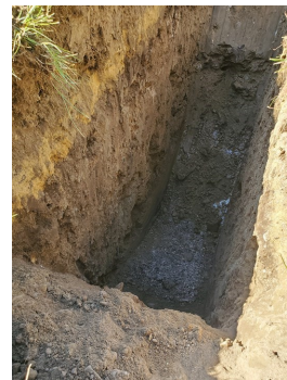
Figure 2: Completed Test Pit - View 2
