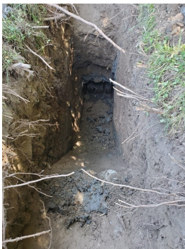
Figure 1: Completed Test Pit - View 1
