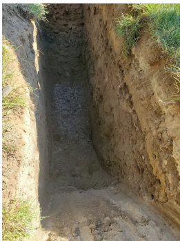
Figure 1: Completed Test Pit - View 1
