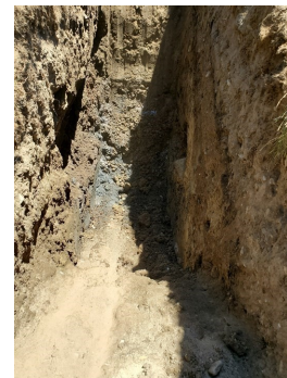
Figure 2: Completed Test Pit - View 2
