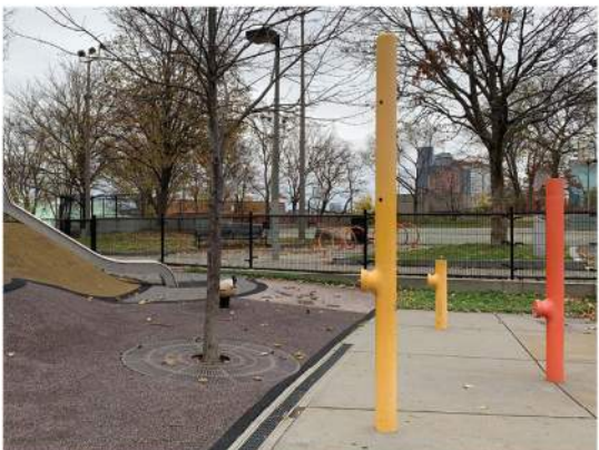
REPAIR OR REPLACE WATER PLAY EQUIPMENT
