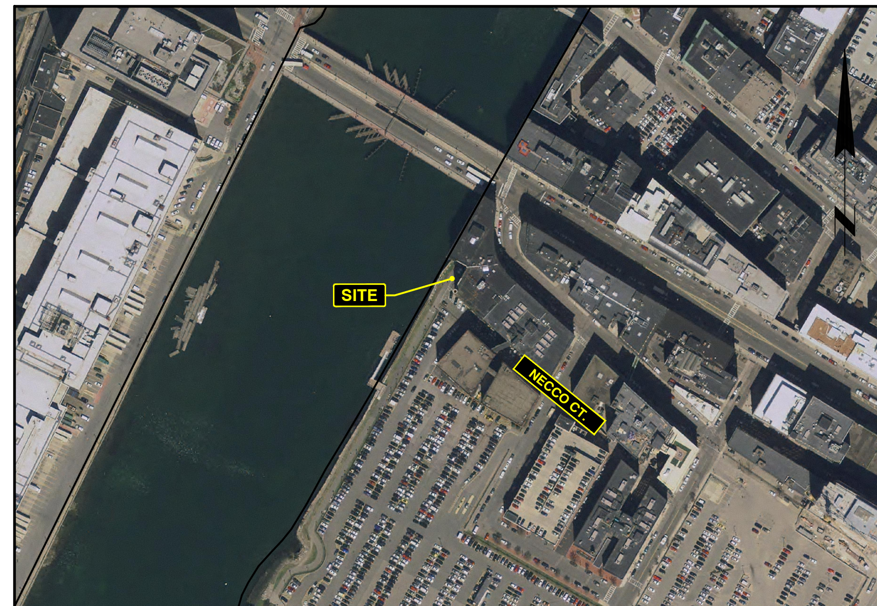
Reference: Aerial Orthophoto from MassGIS website. ( www.mass.gov/mgis ). Photo tile number coq2013_7. Orthophoto was taken in 2013.
