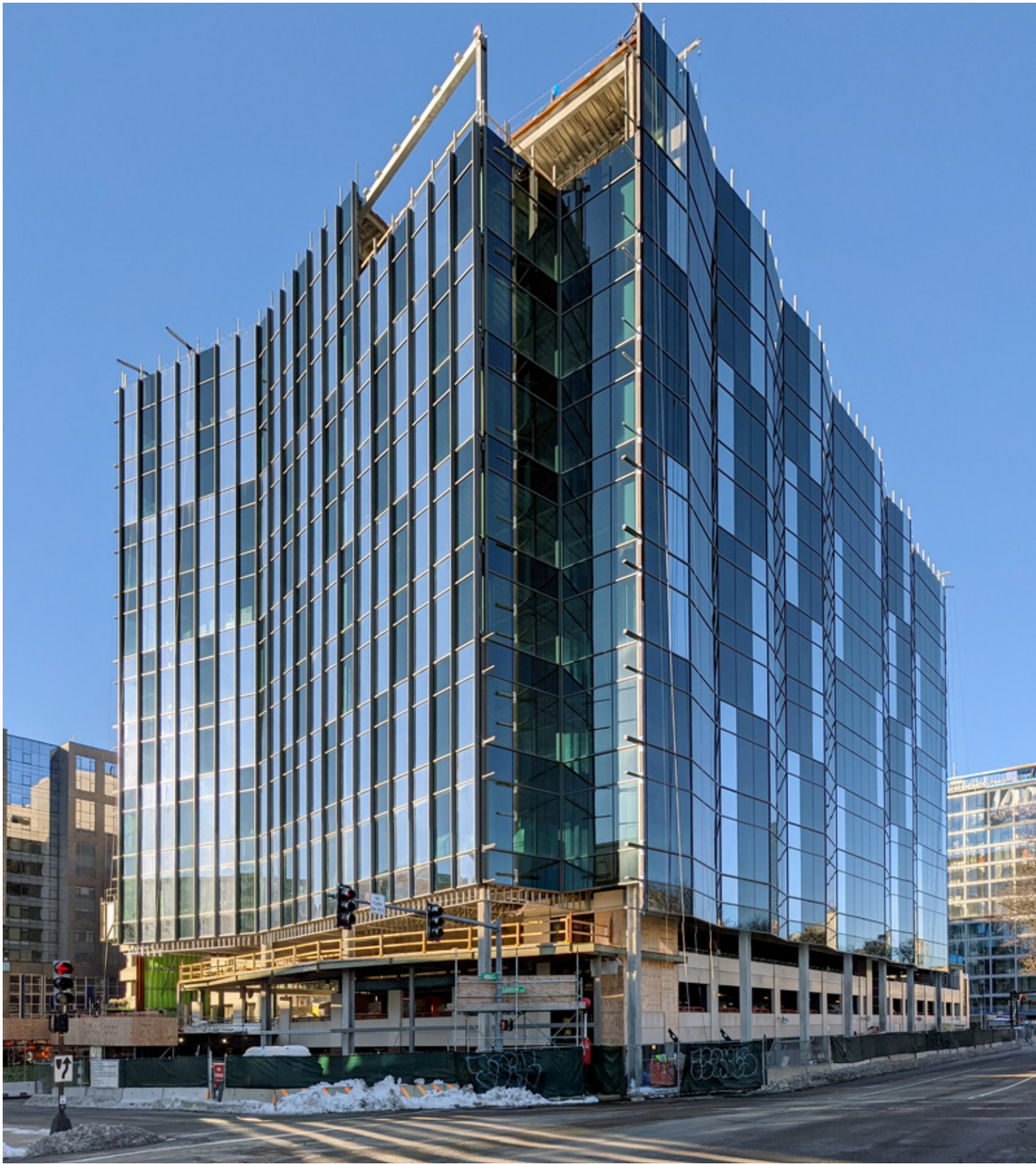
Harrison at Herald St.
