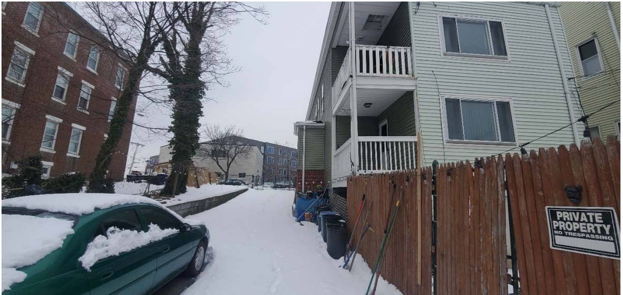
Existing Western Side Yard Facing North
