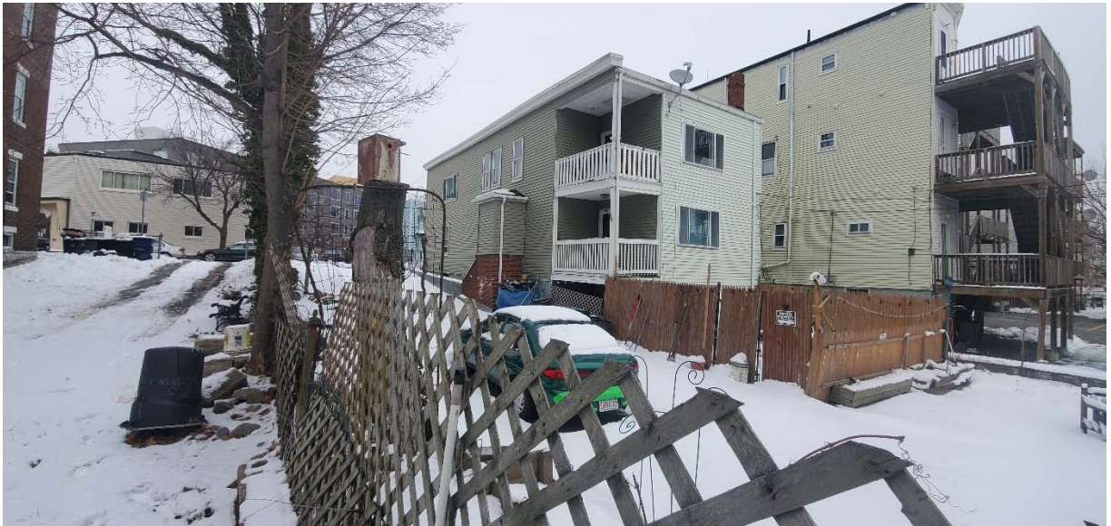
Existing Back Yard and Residential Building Facing North
