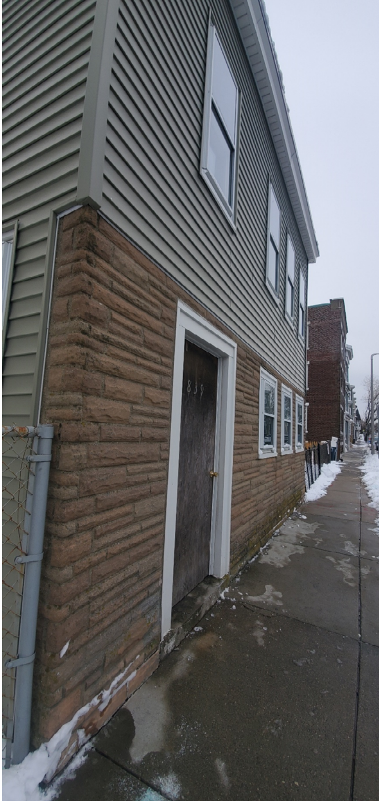
Existing Front Entrance from Saratoga Street
