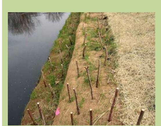
Figure 19. Live Staking
