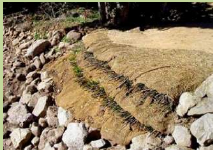
Figure 24. Brush Layering.
