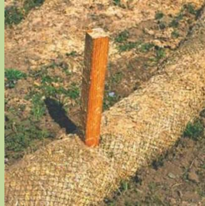
Figure 23. Contour Wattling
