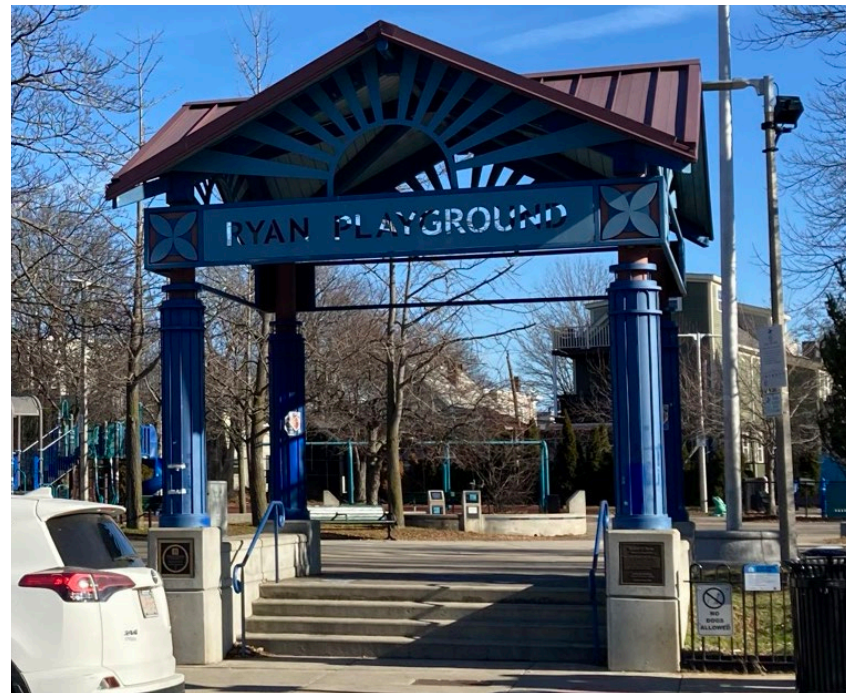
Stairs on Dorchester Avenue
