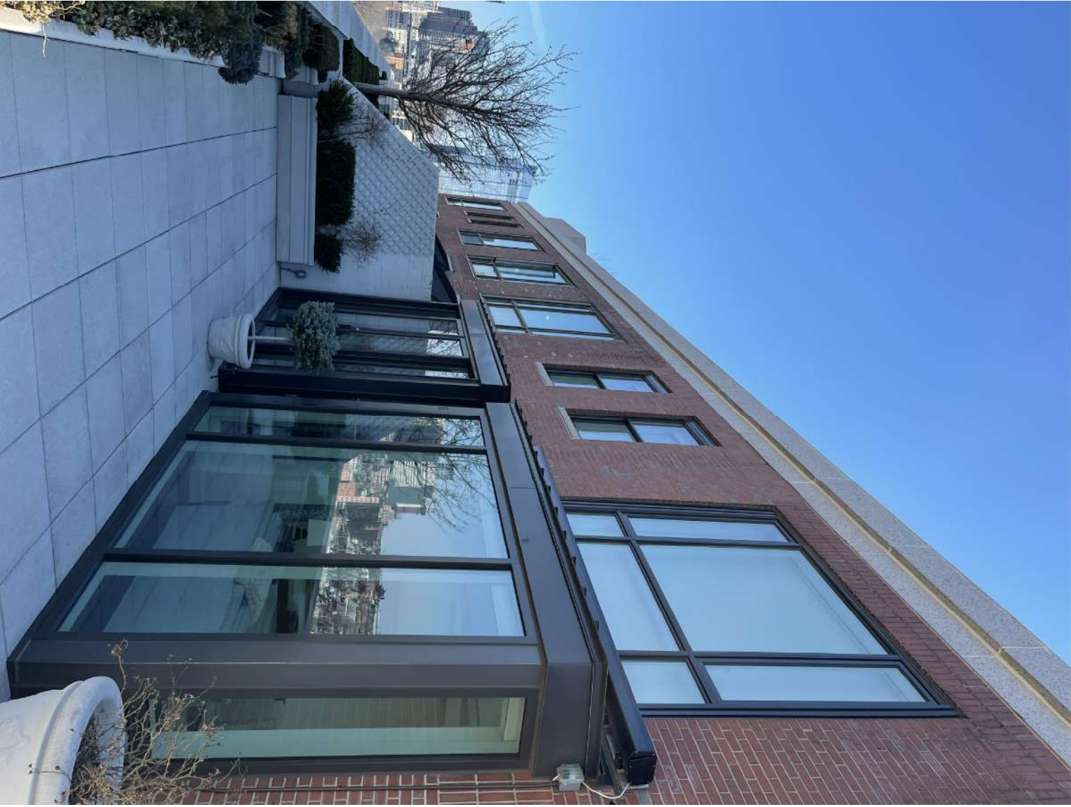
5 EXISTING VIEW 3 - NORTH FACADE, FLOORS 17 & 18
