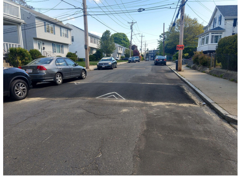
Speed hump with temporary markings and sign
