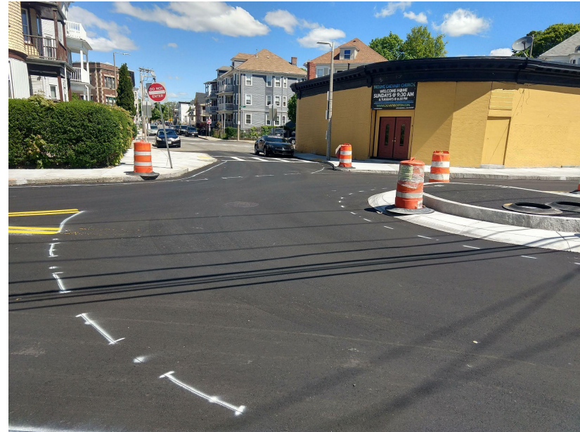
Construction in process on mini-roundabout in TNT zone
