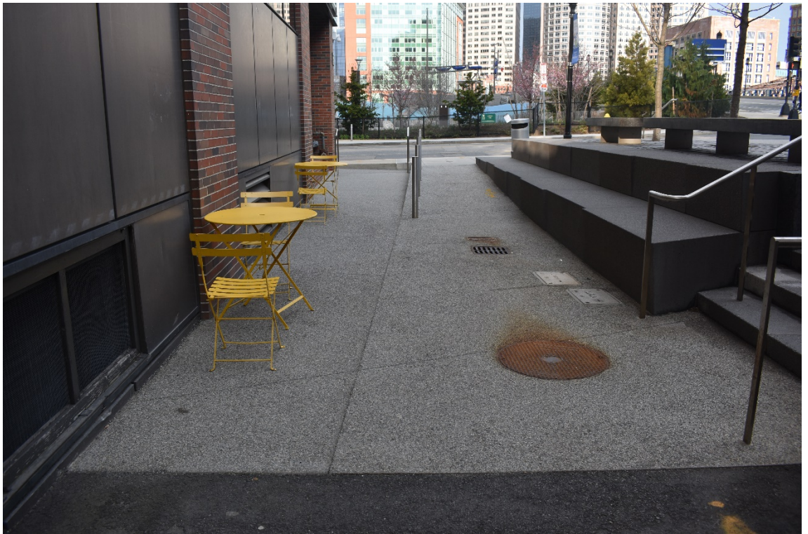
8. North alley between subject building and church plaza, showing grade change.
