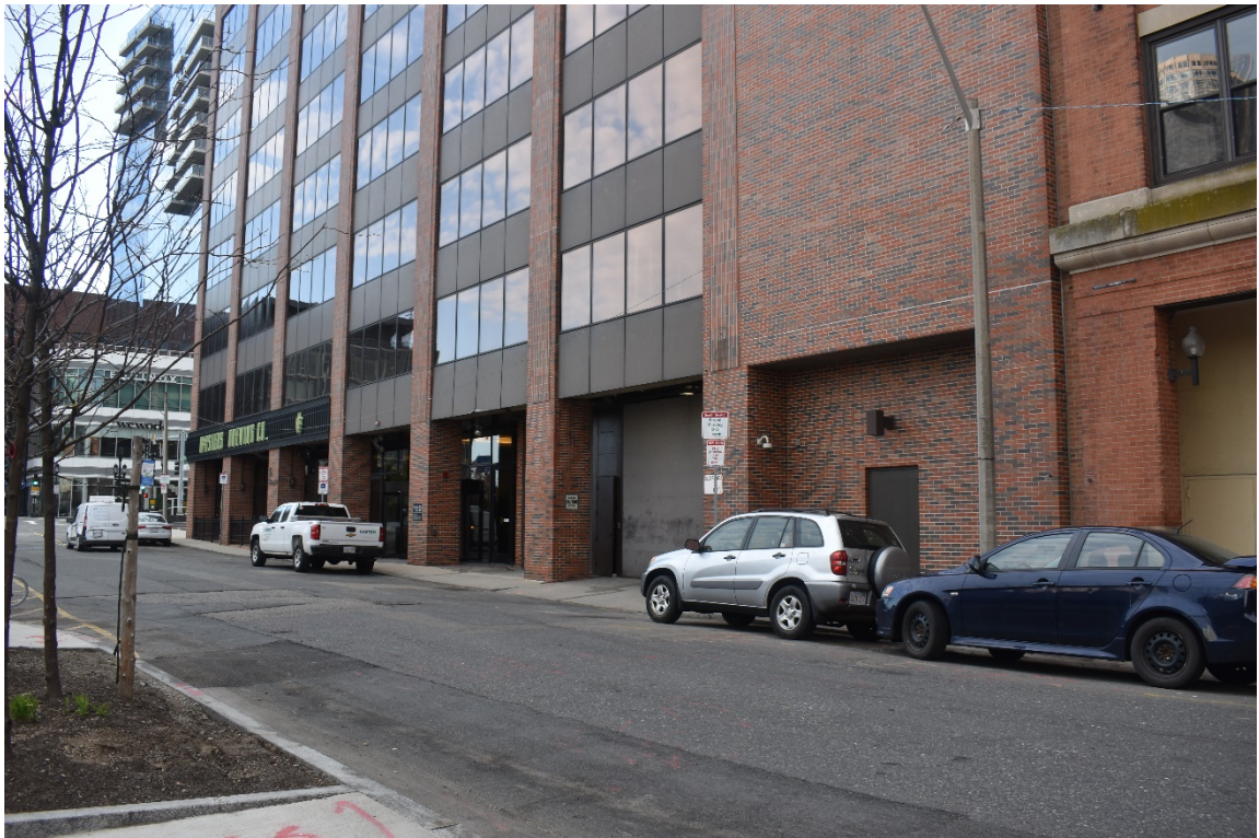
6. Sleeper Street (west) façade showing loading dock bays and stairtower exit. Building at extreme right is next door.
