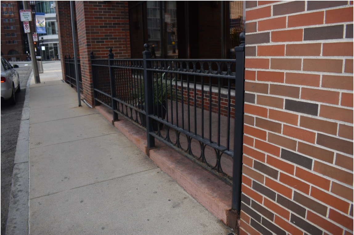
9. Sleeper Street façade at ground floor, showing grade change.
