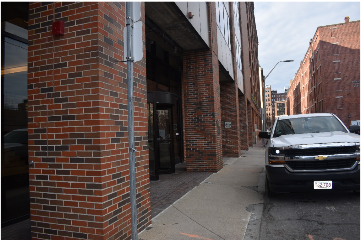
10. Sleeper Street façade at ground floor, showing grade change.
