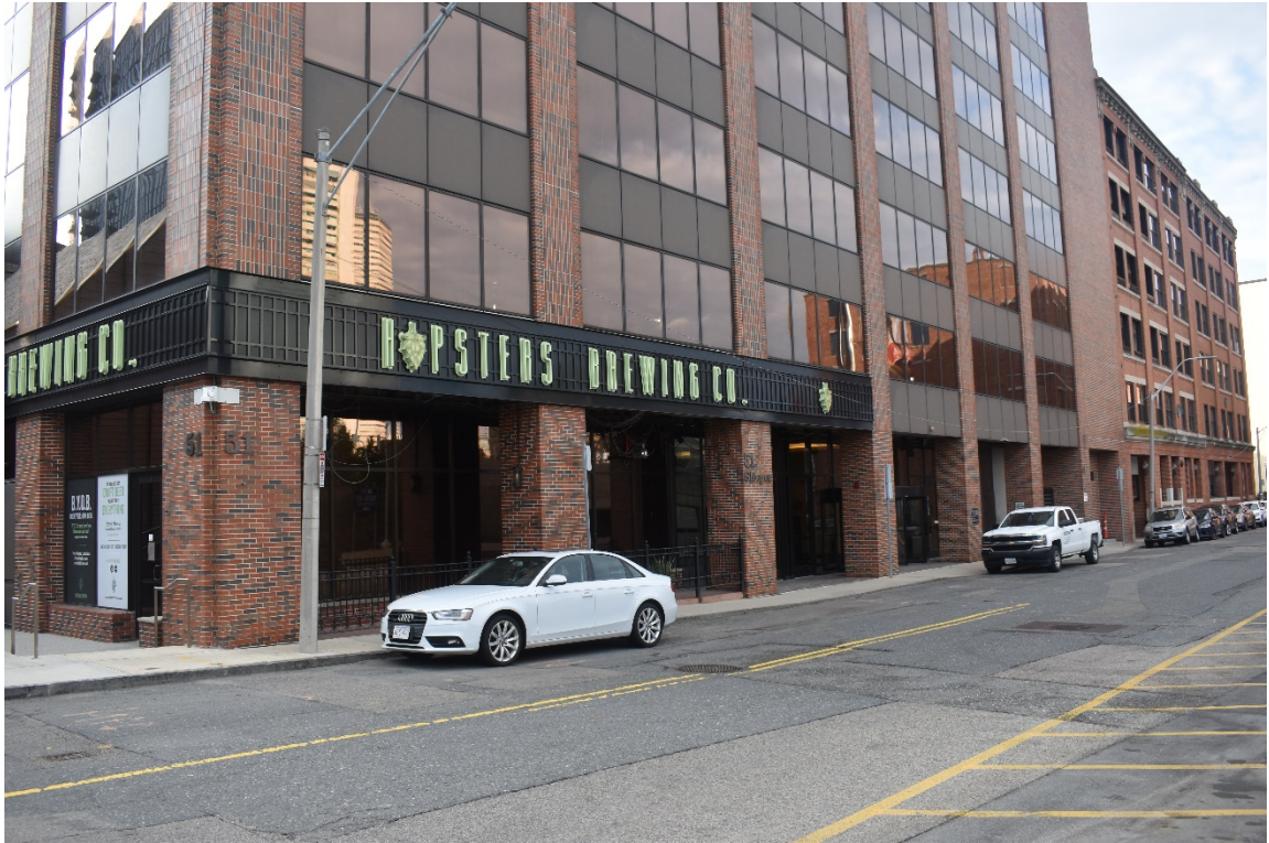
5. Sleeper Street (west) façade.
