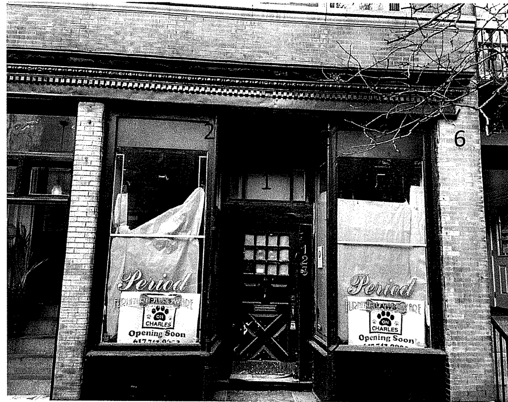
123 Charles' façade – Existing Conditions
