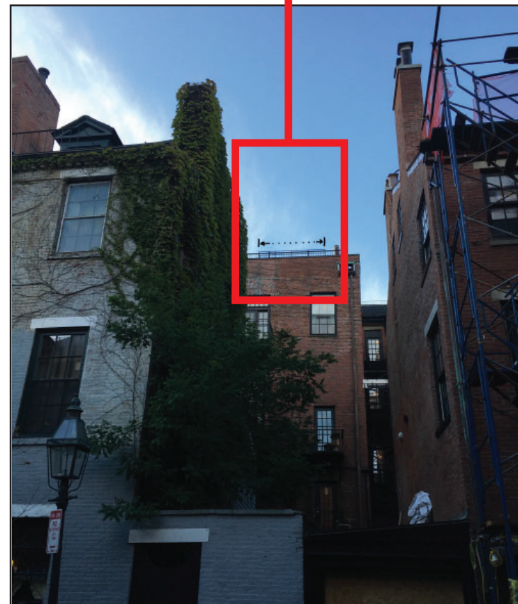
B View from Pinckney Street looking up at former deck railing behind downstairs neighbor's railing.
