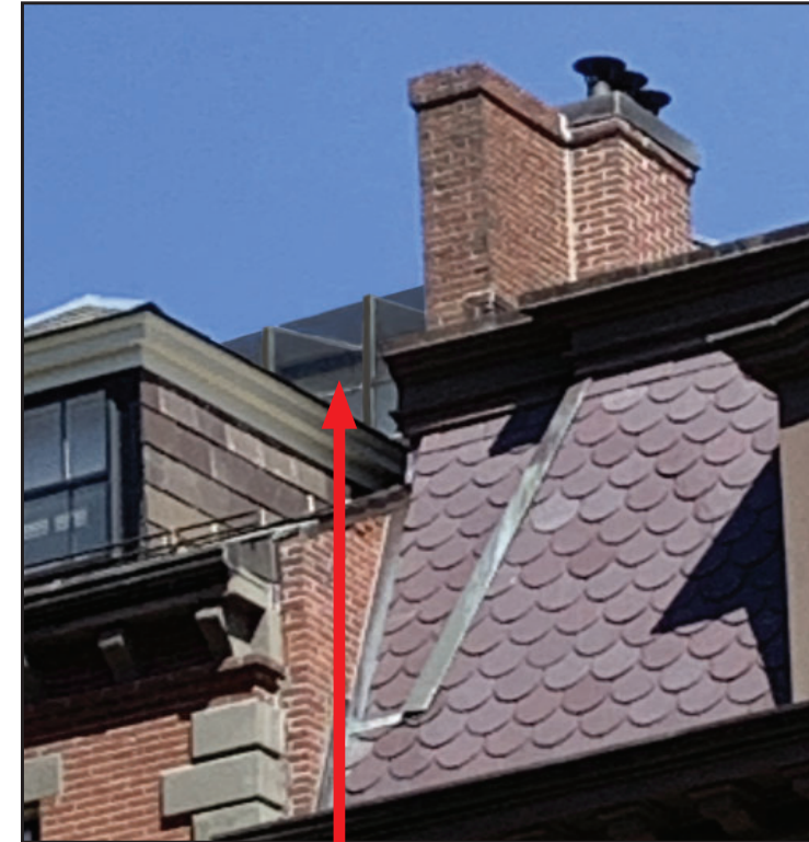
Close up of rendered image illustrating new glazed head house skylight to mimic existing with bronze exterior frame. The replacement frame and glass will be squared off rather than have the rounded design. The new glass has a higher R-value and as such, will be slightly darker in hue.
